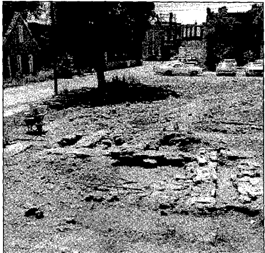
HS-9, June 1971: View to the south. Northeast corner of original foundation uncovered. Lincoln Avenue to the left and the intersection of Lincoln Avenue and Market Street in the center of the background.
