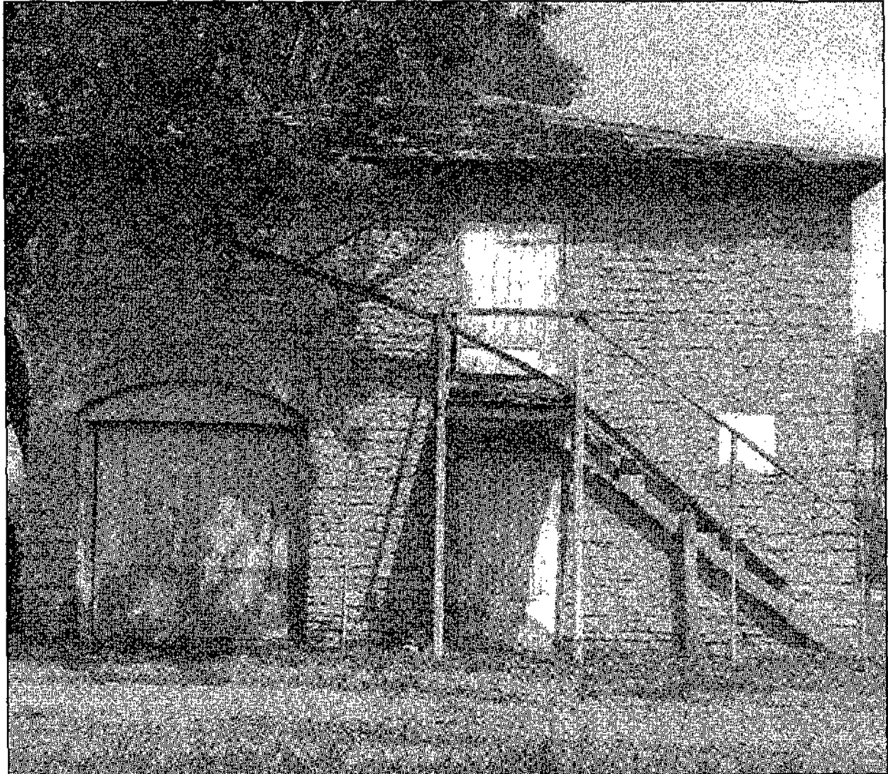
HS-32, Carriage House (South elevation), behind HS-4. Pre-restoration during Historic Building Survey, 1966.
