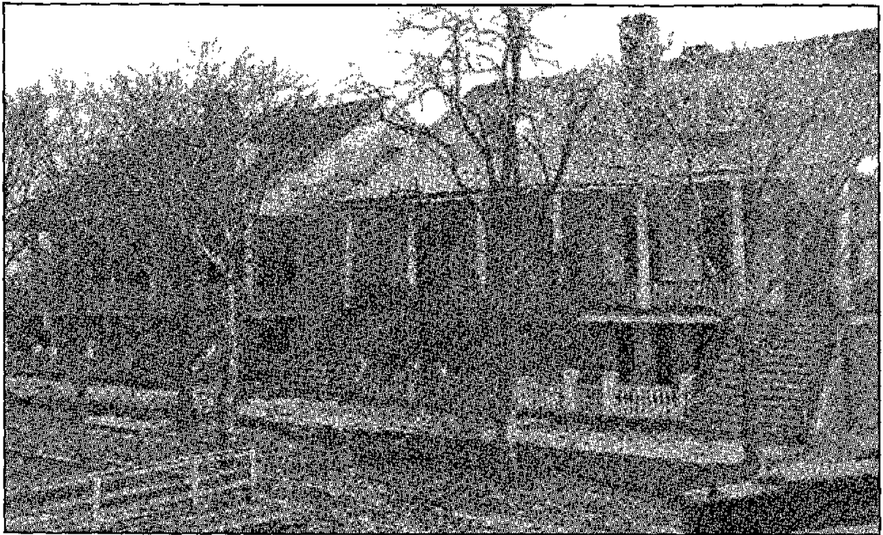
HS-3 (left) and HS-4, (right) front view (South elevation). Foreground: Blair Avenue. Circa 1900.
