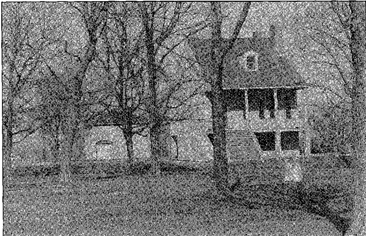
Restored HS-4, front view (Southwest elevation) from Carroll Plaza. Background: restored Carriage House (HS-32), 1976.
