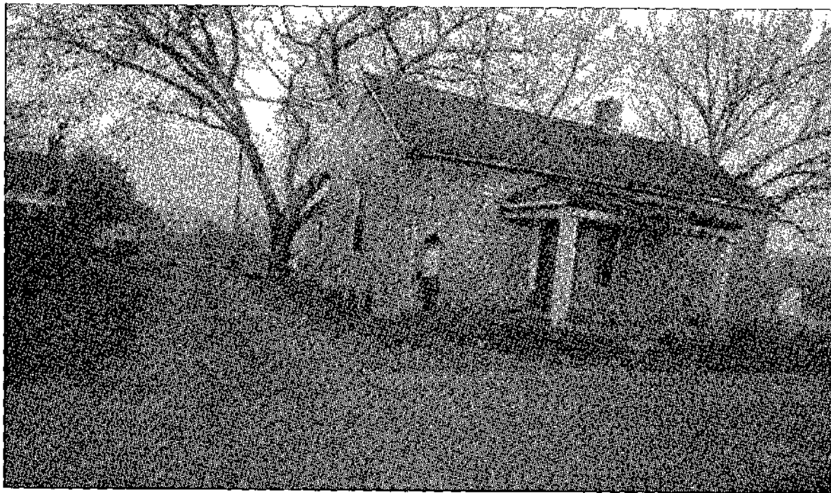
HS-14, Post Bakery, was used as a residence (Southwest elevation). October 1966.
