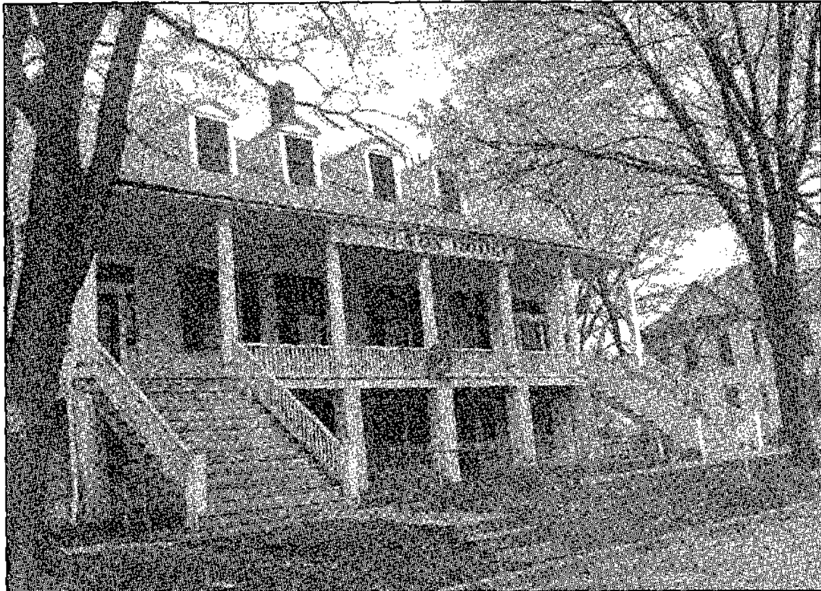
HS-2, front view (South elevation), 1970
