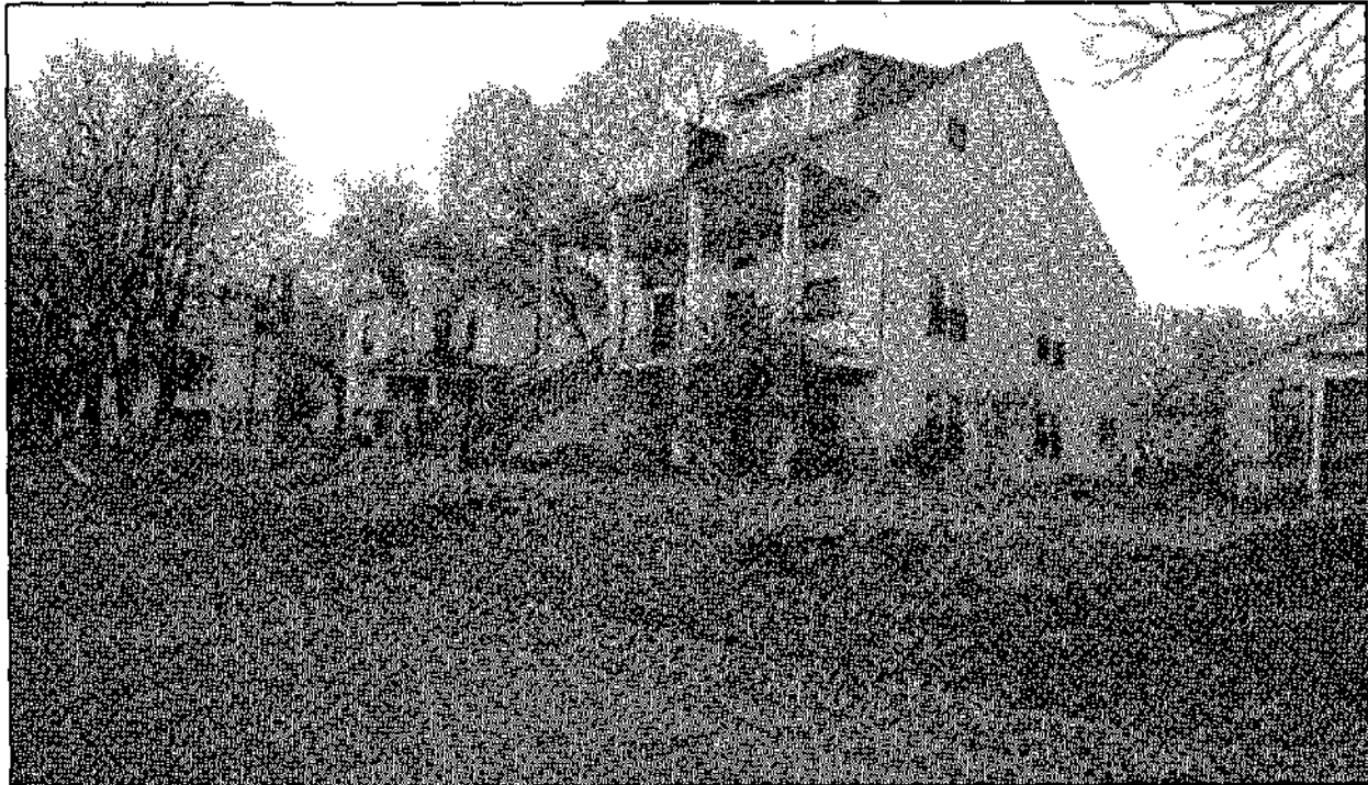
HS-4 west half (Southeast elevation). The east half of this building was destroyed by fire in 1945 and was never replaced. 1966.
