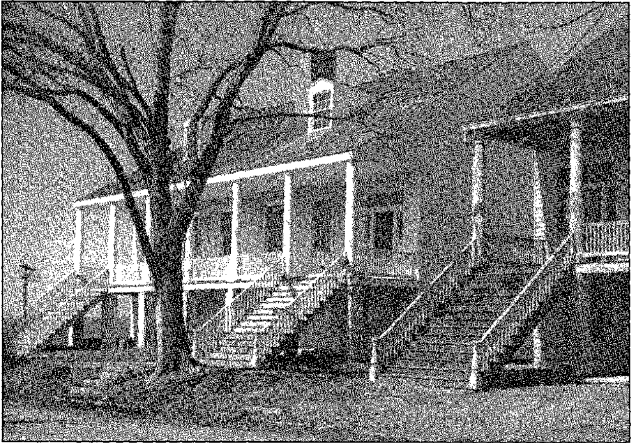
HS-1 (Southeast elevation). Restoration following the May 1967 fire. Photograph 1975.
