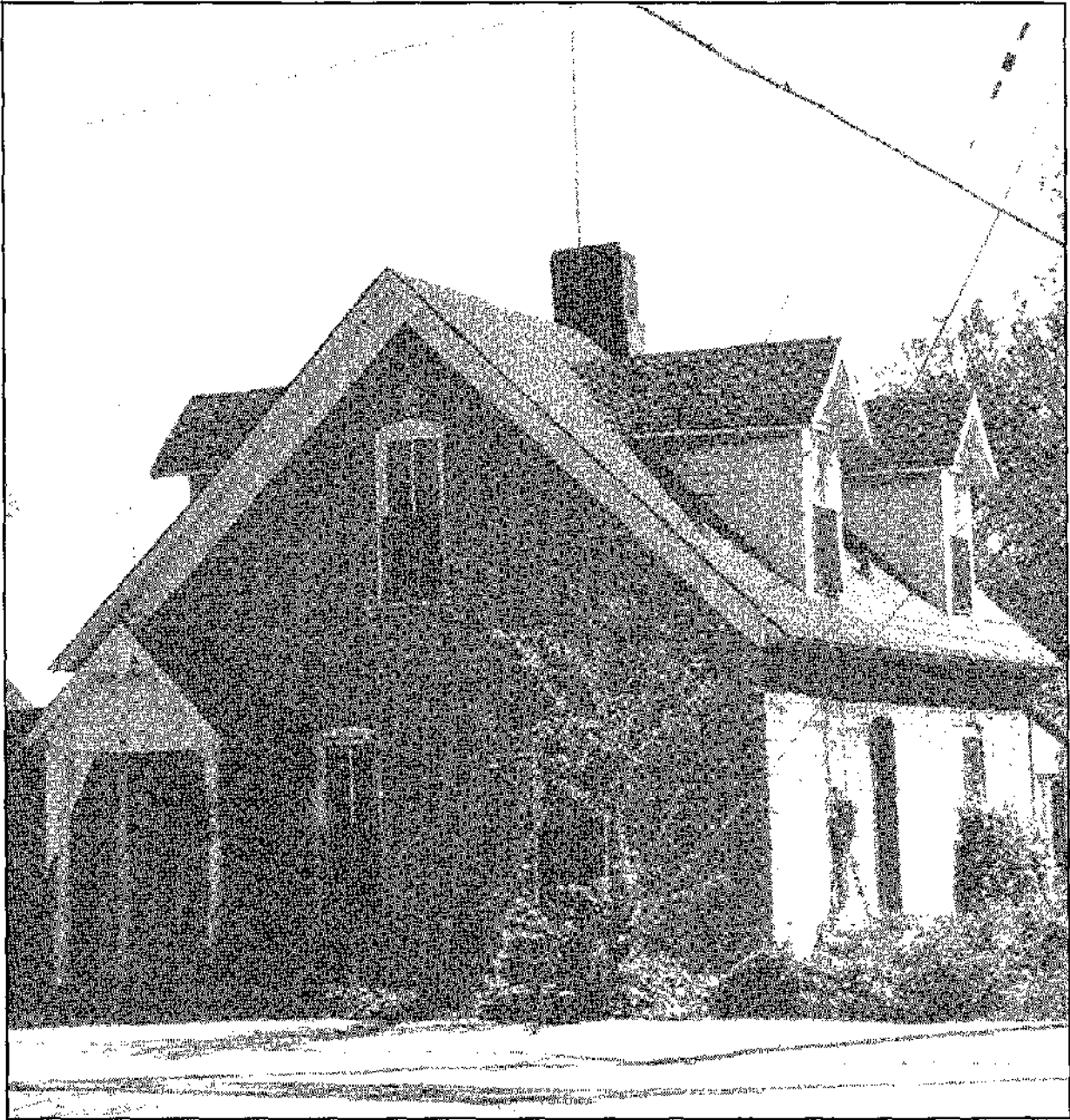
Stone residence razed during Fort Scott's Urban Renewal Project from 1965 to 1970, because it was not part of the site's historic period from 1842 to 1873. Formerly located on Lincoln Avenue, across from and south of the razed city jail where the present Post Guardhouse (HS-9) is located. Circa 1970. Note: Research indicates that this building was mistaken for HS-33. HS-33 was a small frame building located directly across from the former City Jail and the present reconstructed Post Guardhouse on the east side of Lincoln Avenue. It was razed prior to the Fort Scott Urban Renewal Project.
