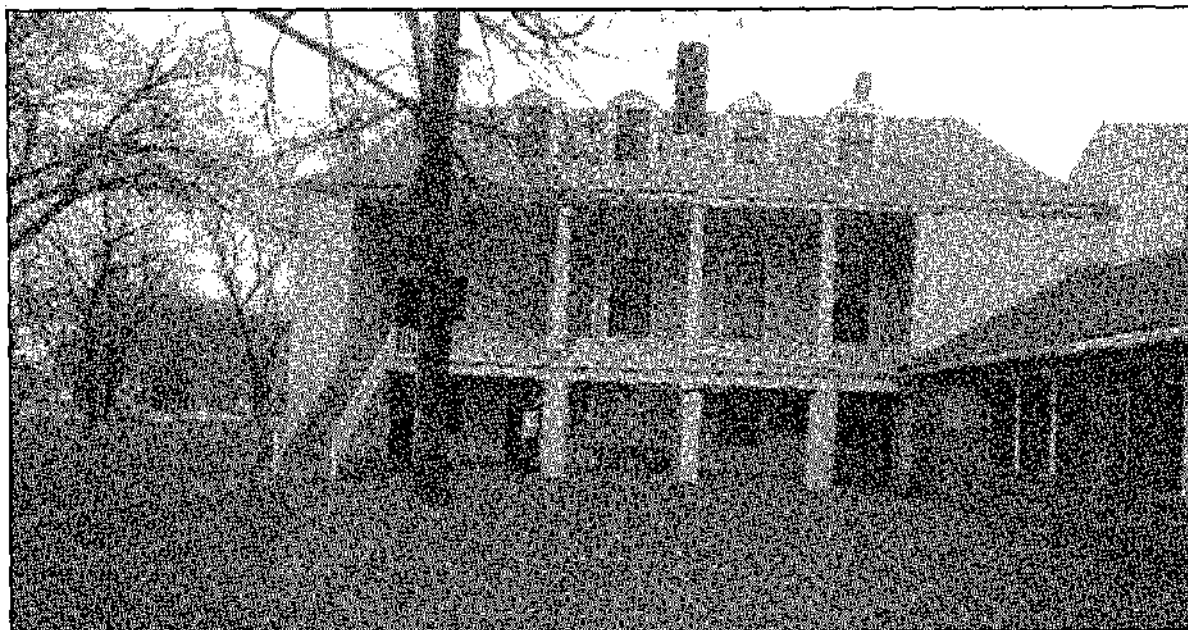
HS-2, rear view (North elevation). Note: brick addition, right, contained furnace room and steam laundry of the former Goodlander Home. 1970.
