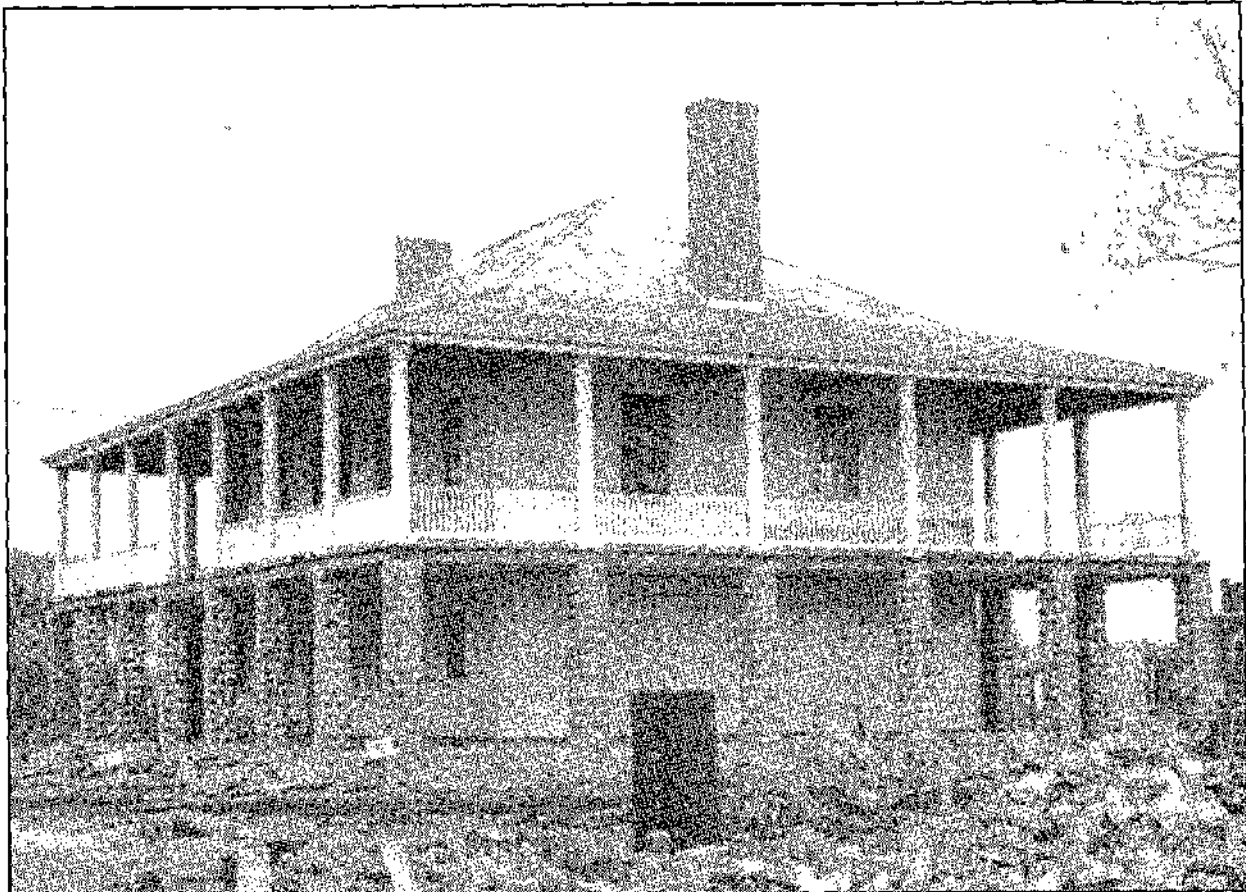
HS-8, Post Hospital/Visitor Center, reconstruction in progress (Northwest elevation). 1974.
