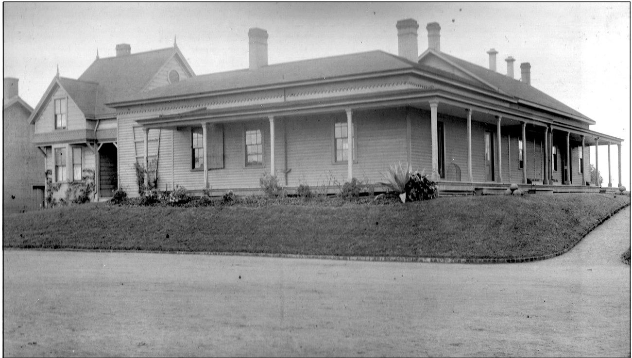
Figure 2.3.7: Though consistently well-kept throughout, treatment of vegetation varied from building to building. “Hospital & Stewards Quarters,” c. 1891. National Archives RG92, Still Photography Division, Box 10, Series F, (92-F-37-7).
