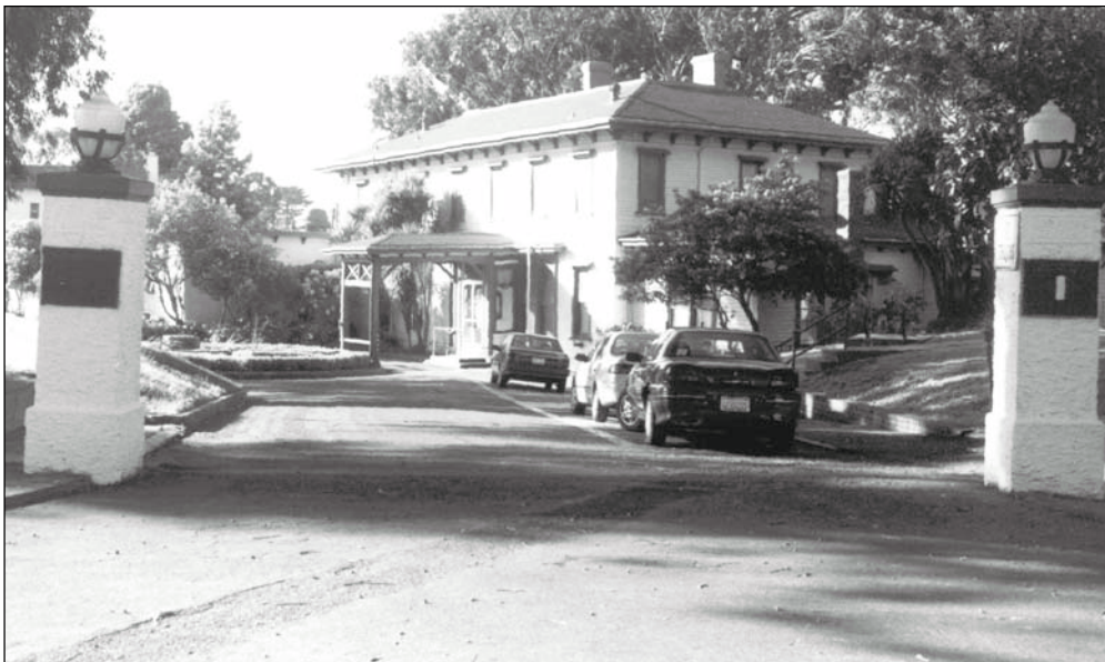
Figure 5.2.3: McDowell Hall Driveway and Carriage Turn. Excluding the gateposts, the configuration of this driveway is consistent with its appearance on an 1890 map of the post. Contributing. 7/02 - OCLP.
