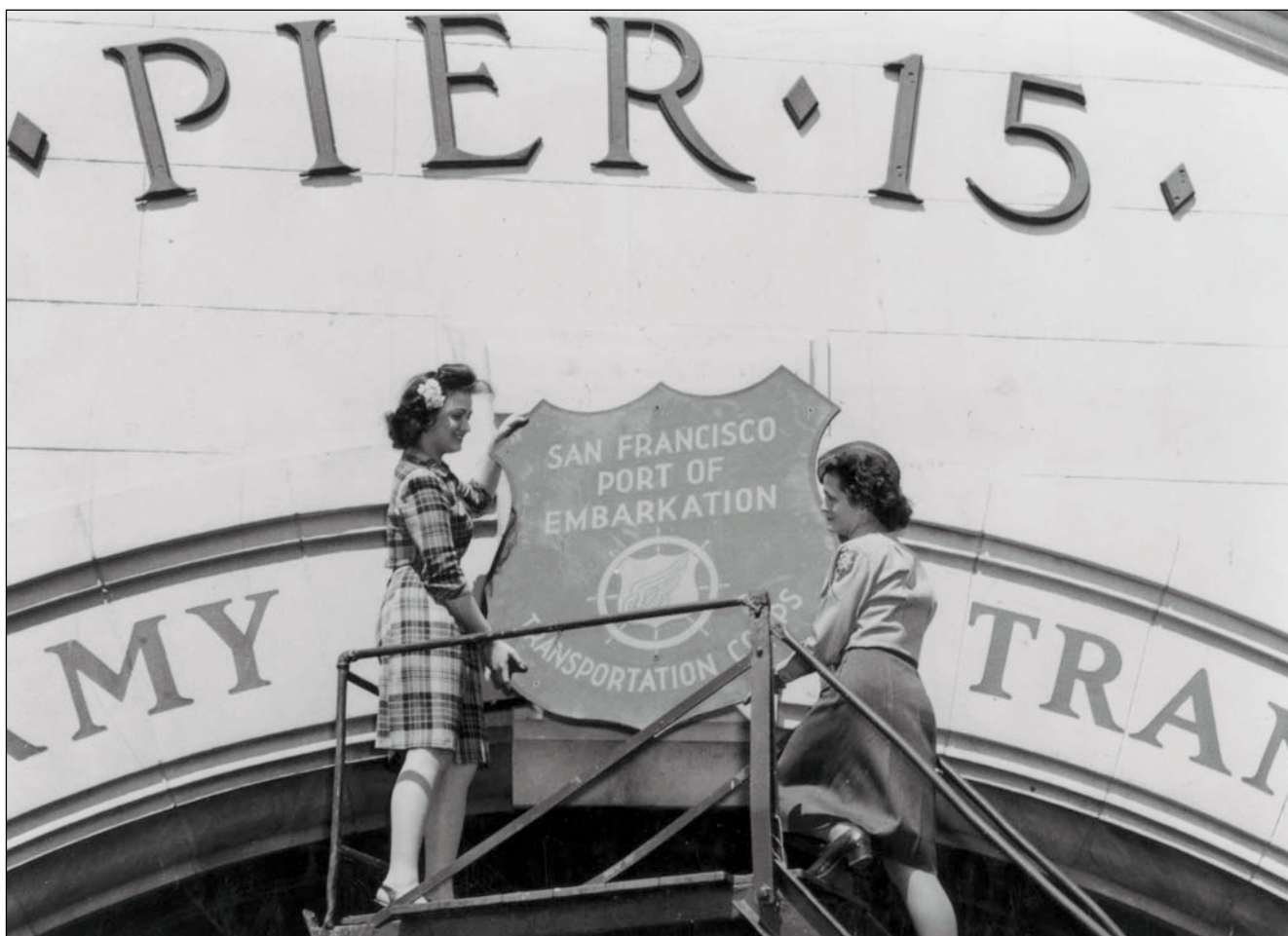
Figure 2.5.25: In 1932, the Army's operation of the San Francisco General Depot at Fort Mason was linked to other Transportation Corps facilities in the Bay area, becoming the headquarters of the San Francisco Port of Embarkation (SFPE). This World War II era image is of the port facilities located along the Embarcadero. San Francisco Public Library, San Francisco Historical Photograph Collection, Record AAC-2315, June 29, 1946.
