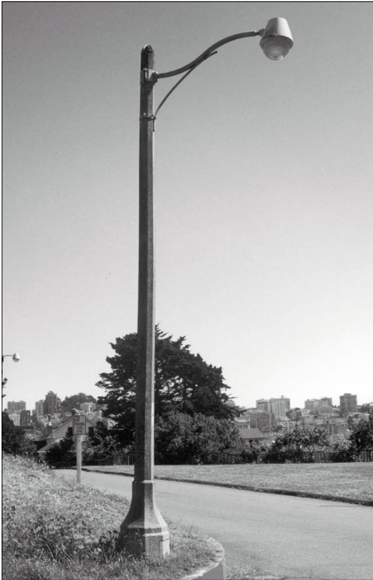
Figure 5.1.3: Cast Concrete Light Poles. These features are known to be post WWII. Post maps suggest that they were installed c. 1960. Requires further evaluation. 7/02 - OCLP.
