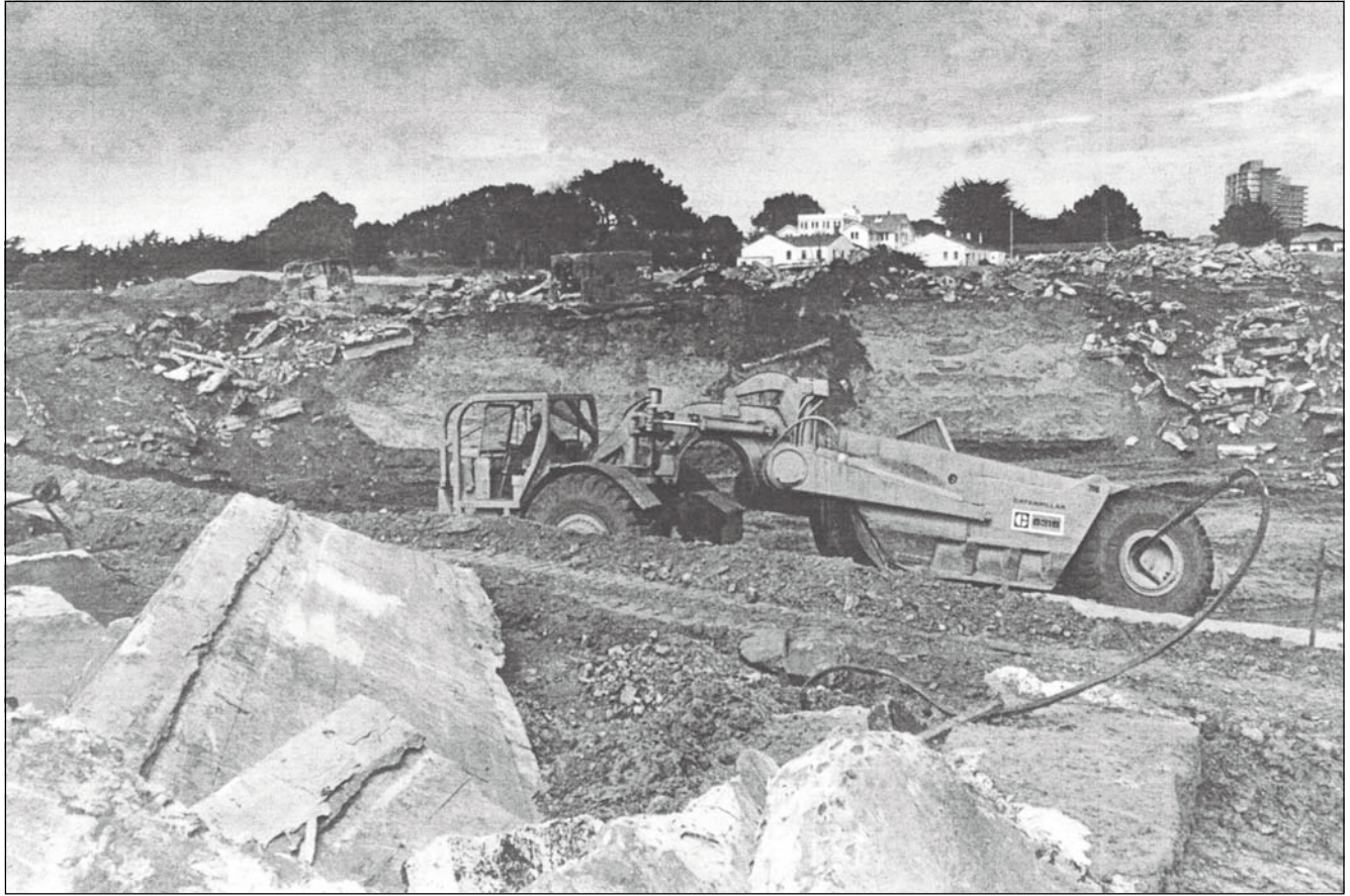
Figure 2.7.6: The creation of the “Great Meadow” suggested by the planning process, required the removal of dozens of building foundations and the western half of MacArthur Avenue. Image is c.1980. NPS, GGNRA Archives, Richard Frear Collection.
