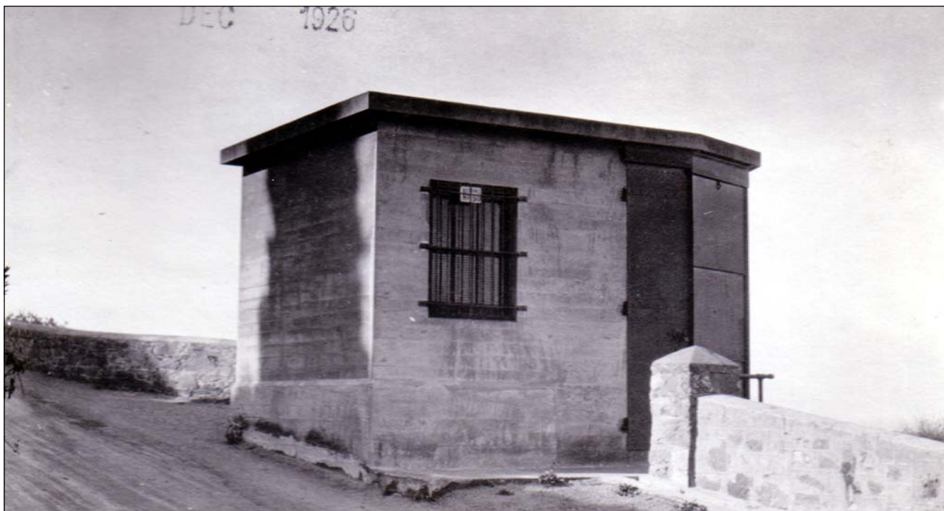
Figure 2.5.14: After the removal of Fort Mason's artillery in 1908, and prior to the invention of radar, powerful 60-inch searchlights became the last vestige of the fort's defensive mission. This was one of approximately one dozen similar installations located near the entrance to the bay, 1926. National Archives, RG 77, Office of the Quartermaster General, Records of the Construction Division - Annual Construction, Maintenance, and Repair Reports (1924-1938) Box 135NM.
