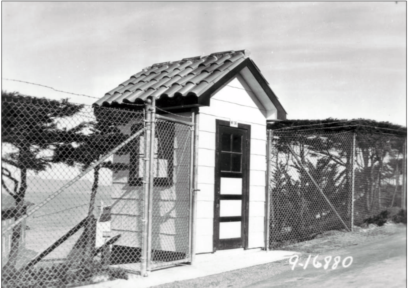
Figure 2.5.22: Red tile roofing, a characteristic feature of the Mission Revival was later applied to even the most humble architecture at Fort Mason. Note the consistent pruned height and scarcity of lower branches of the hedge material at the top of the slope at this date. Watch station, August 1939. National Archives, RG 77 Office of the Quartermaster General, Records of the Construction Division - Annual Construction, Maintenance, and Repair Reports (1924-1938) Box 135NM.
