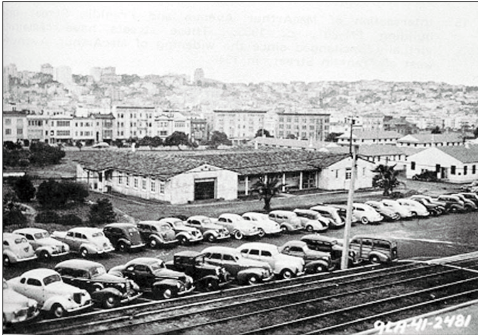
Figure 2.5.27: Although better known for its work at state and national parks, the Civilian Conservation Corps (CCC) also worked at many military bases. Many changes were made to Fort Mason during the CCC program, including the parking area along MacArthur Avenue shown in this post-CCC photograph. Image copied from “Historic Structure Report, Western Grounds, Old Parade Ground and MacArthur Avenue,” Figure Number 13, Page 105, 1980.
