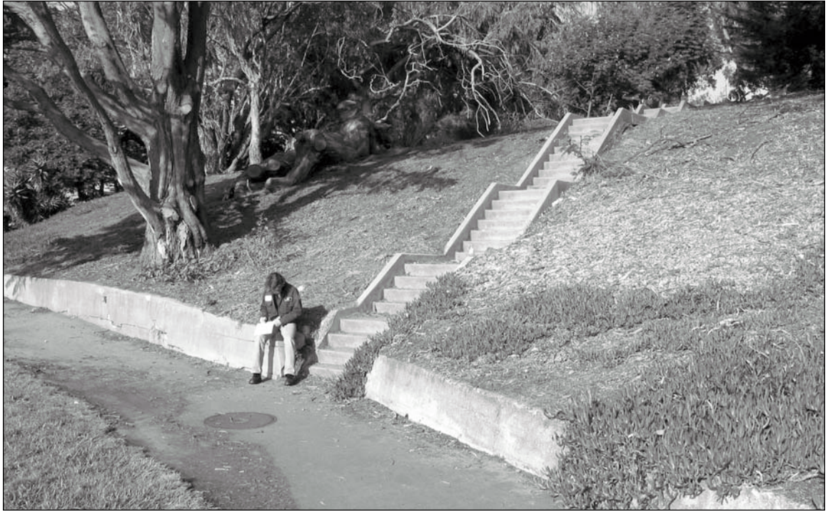
Figure 5.4.4: Concrete Stair Between Parade Ground and Great Meadow, (FM - 407). This stairway was constructed c1938, replacing an earlier wooden stair at the same location. Contributing. 12/02 - OCLP.
