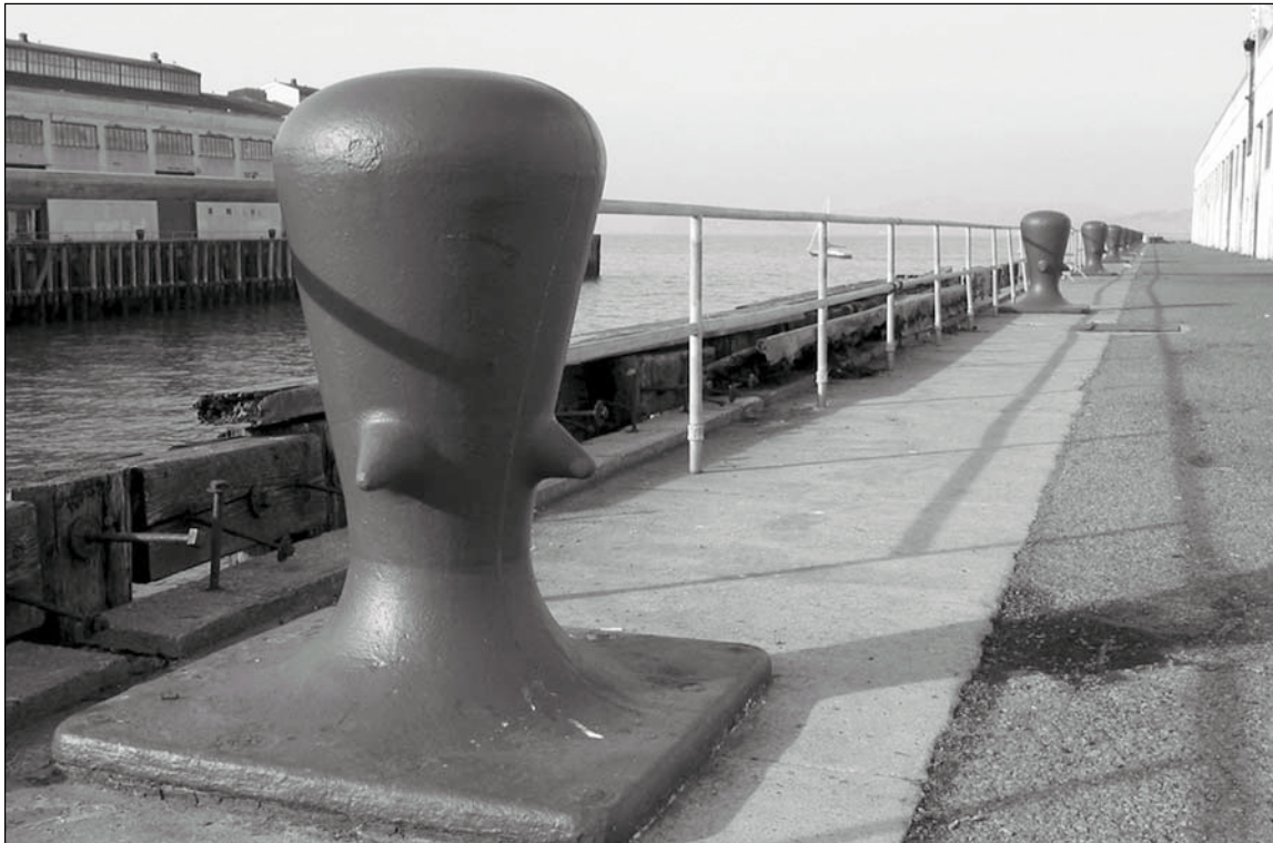
Figure 5.10.10: Mooring Bollards. Large marine bollards such as this were once used to moor large ocean-going ships. Contributing. 12/02 - OCLP.
