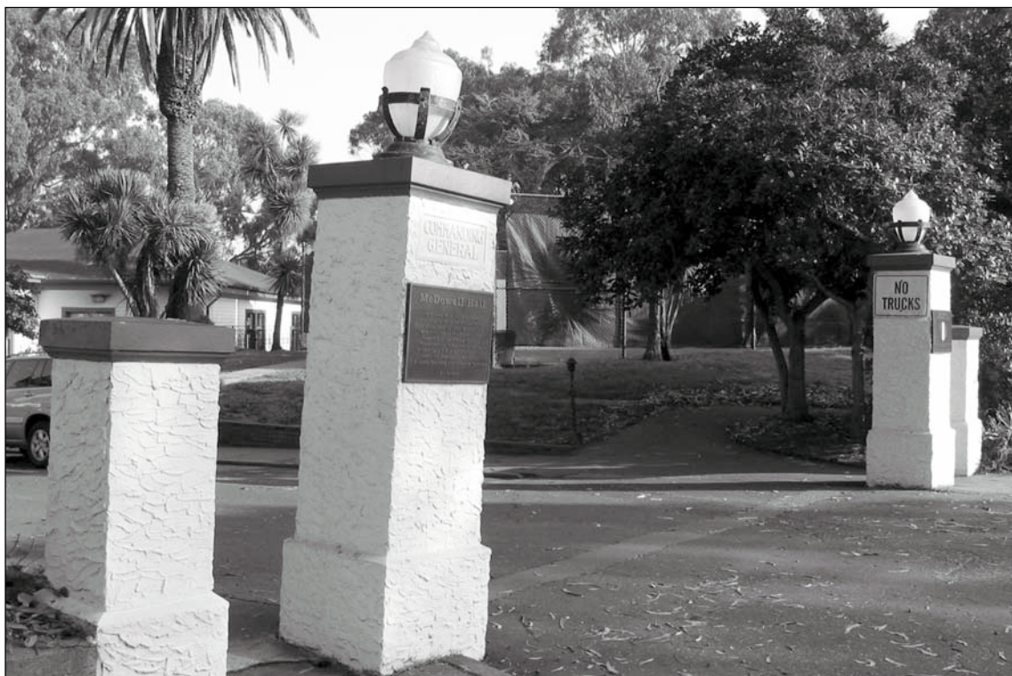
Figure 5.2.14: McDowell Hall Entrance Gate. Gates of various designs have appeared at this location since 1877, when this building became the residence of the Commanding General of the Department of the Pacific. Construction dates for the existing gateposts are unknown, but are thought to have been in place prior to WWII. Contributing. 12/02 - OCLP.
