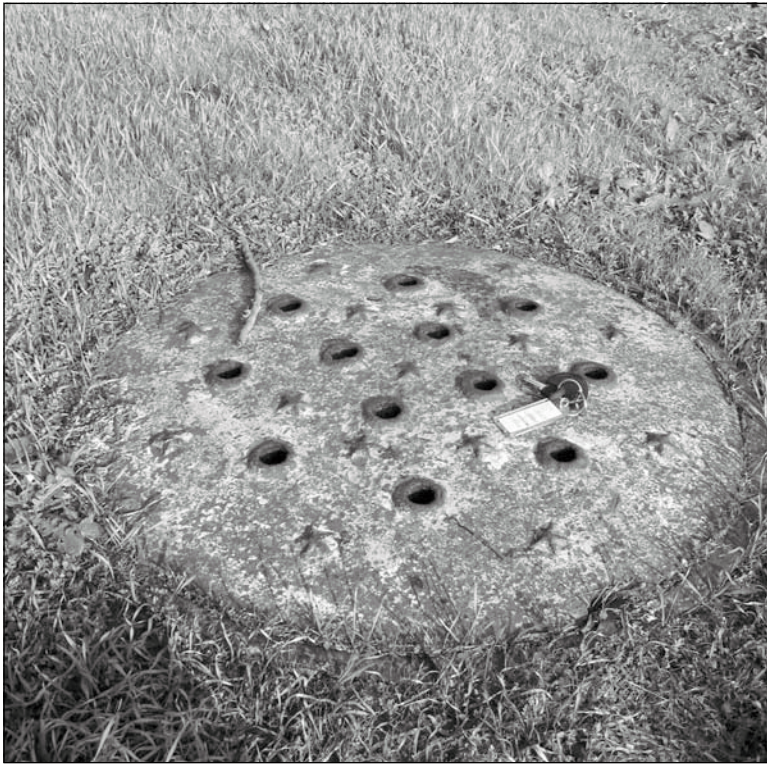
Figure 5.1.11: Manhole Covers. Many of the access covers to sewers and utility vaults bear military insignia, designations and decorations. Contributing. 12/02 - OCLP
