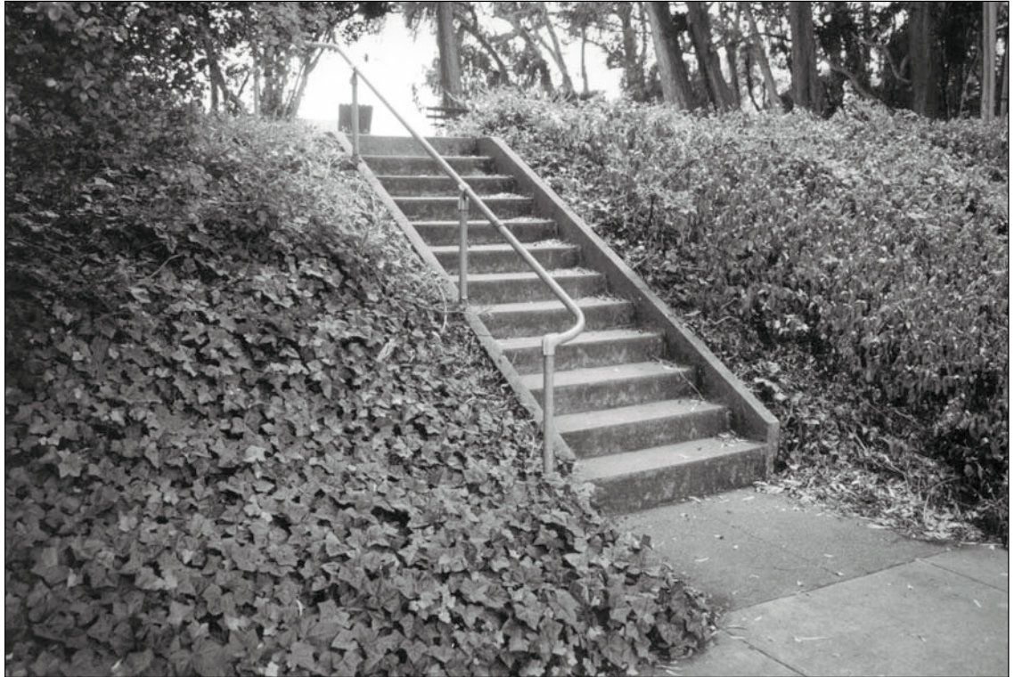
Figure 5.3.4: System of Pedestrian Paths and Stairs. Pedestrian paths and walks are commonly surfaced with poured-in-place concrete. Concrete stairs are fitted with modern safety handrailings. Contributing. 12/02 - OCLP.
