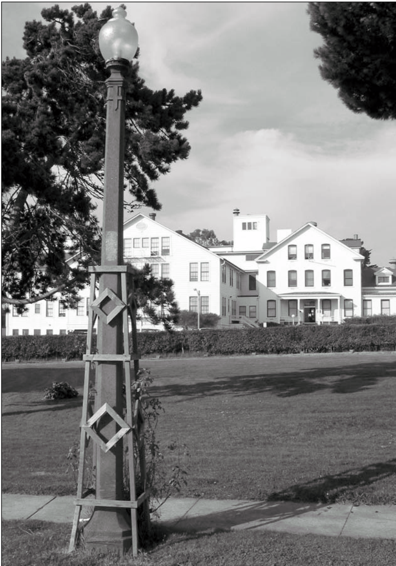
Figure 5.9.11: Cast-concrete Lightpoles - Officers' Park. Contributing. Neither the plastic replacement globes or the lattice vine supports are historic. 12/02 - OCLP.
