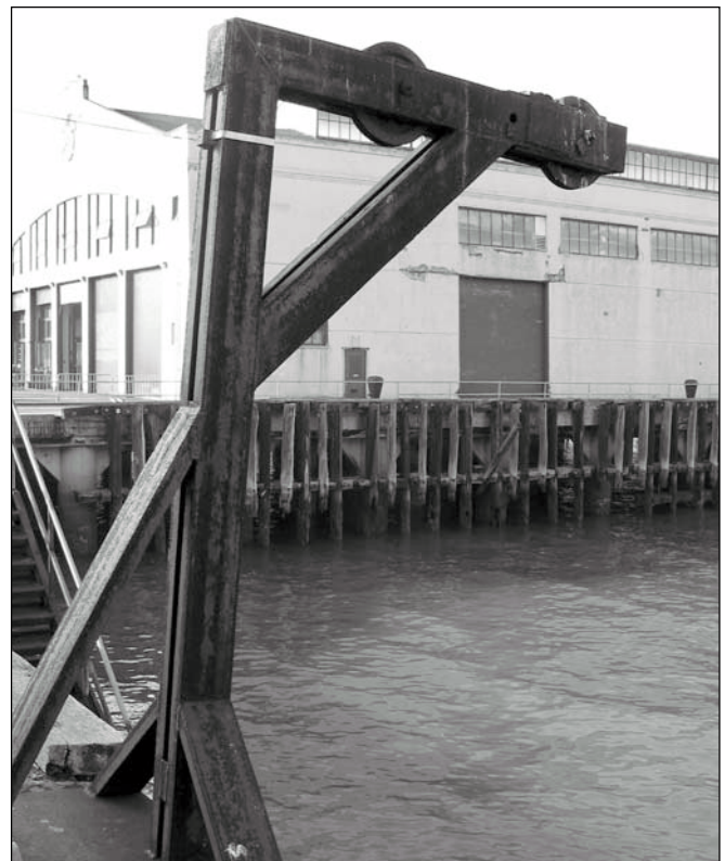
Figure 5.10.8: When found in pairs, small hoists such as this are known as “davits.” These are used to move small boats in and out of the water. This pair of davits is in poor condition and is likely to date to the period of significance. Contributing. Pier #2 and Pier Shed #2 are shown in the background. 12/02 - OCLP.
