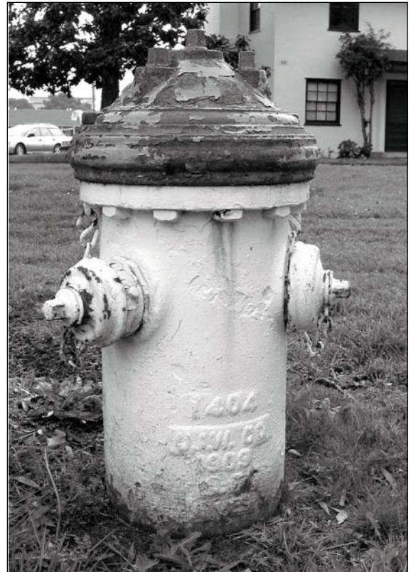
Figure 5.1.6: Emergency High Pressure Fire Hydrant. These features, dated 1909, were installed 1910-1911 in conjunction with the city's emergency pumping stations at Van Ness Avenue and Townsend Street. Contributing. The status of other types of fire hydrants at Fort Mason requires further evaluation. 12/02 - OCLP.
