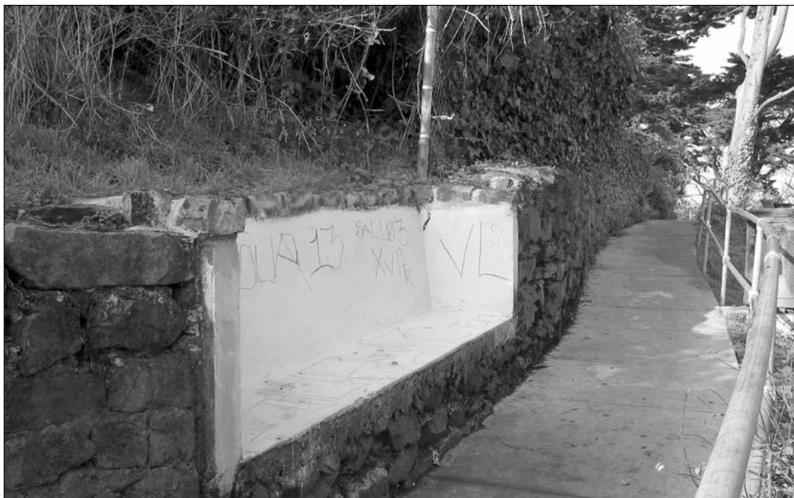
Figure 5.2.15: Stone Retaining Walls with Built-in Seats. After the U.S. Army's arrival in 1863, the garden pathways belonging to the formerly private residences were reused for the pleasure of the Officers' corps. This wall and seat is a fairly well-maintained example of many similar arrangements found on the east slope of the peninsula. Contributing. 12/02 - OCLP.
