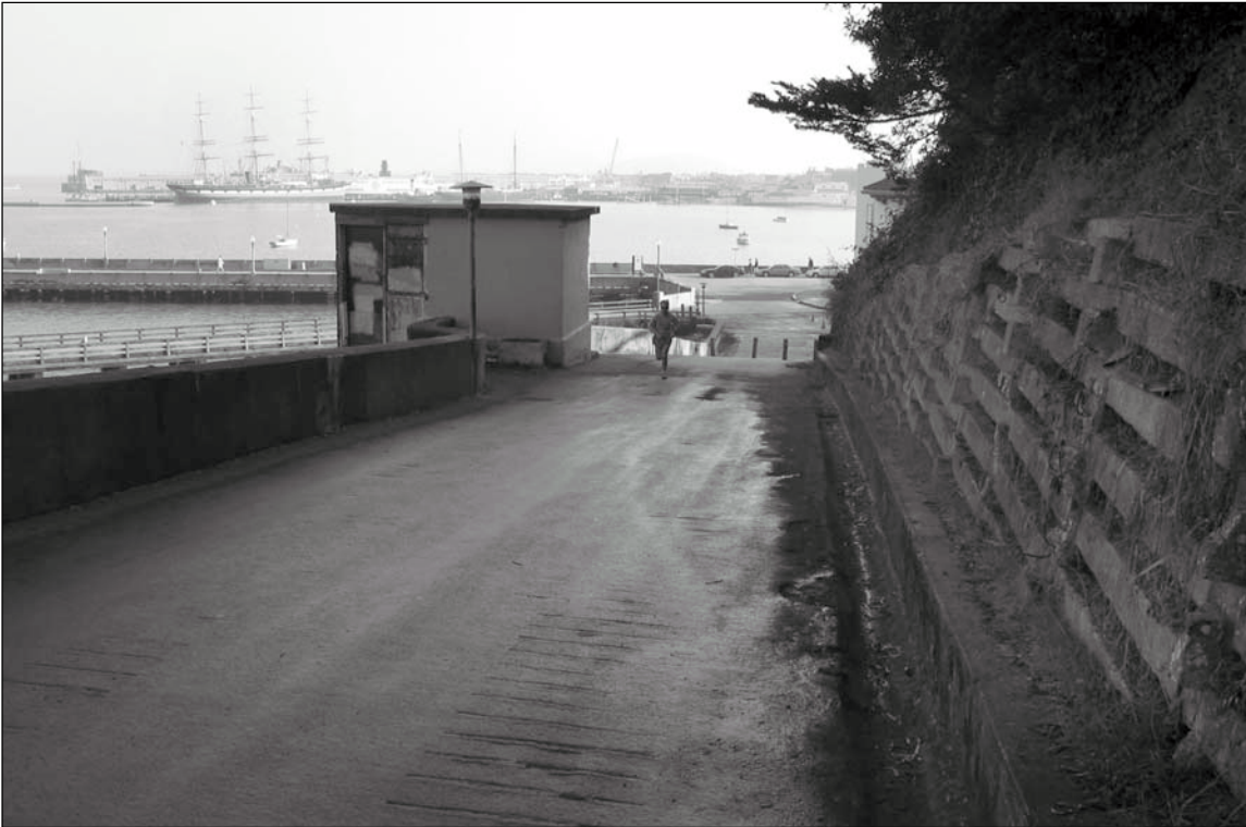
Figure 5.3.2: McDowell Avenue. This road was constructed into the northern cliff of Black Point c.1877 to provide access to the Quartermaster Wharf (Pier 4). Contributing. 12/02 - OCLP.
