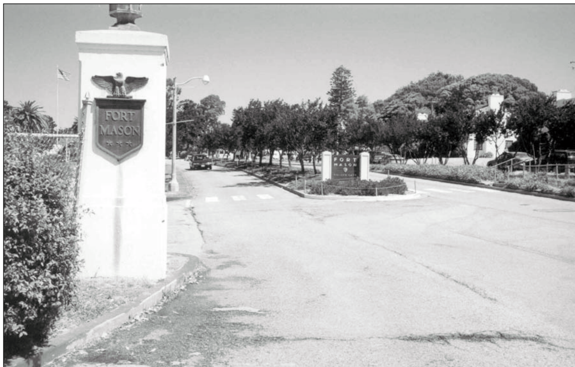
Figure 5.9.3: Franklin Street Extension, (section between Bay Street and MacArthur Avenue). This section of road was constructed between 1944 and 1947 as an improvement to an entrance in the same location. Contributing. The center median was added by the NPS in 1974. 7/02 - OCLP.
