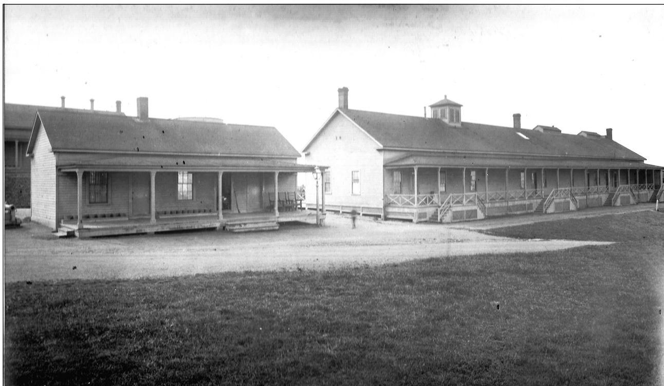
Figure 2.3.9: A guard house, or jail, was an integral fixture in administering military discipline. Its proximity to the main barracks was a convenience. The landscape details were more spartan in this area. “Guard House & Barracks,” c.1891. National Archives, RG92, Still Photography Division, Box 10, Series F, (92-F-37-4).
