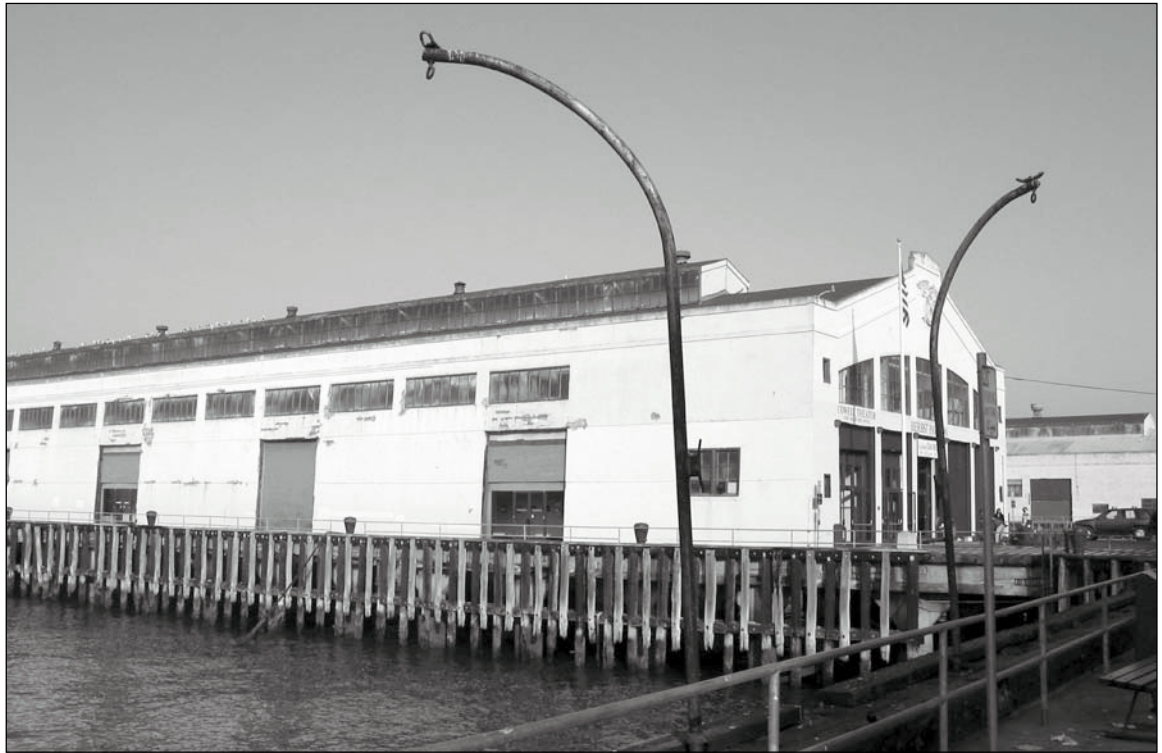
Figure 5.10.8: When found in pairs, small hoists such as this are known as “davits.” These are used to move small boats in and out of the water. This pair of davits is in poor condition and is likely to date to the period of significance. Contributing. Pier #2 and Pier Shed #2 are shown in the background. 12/02 - OCLP.
