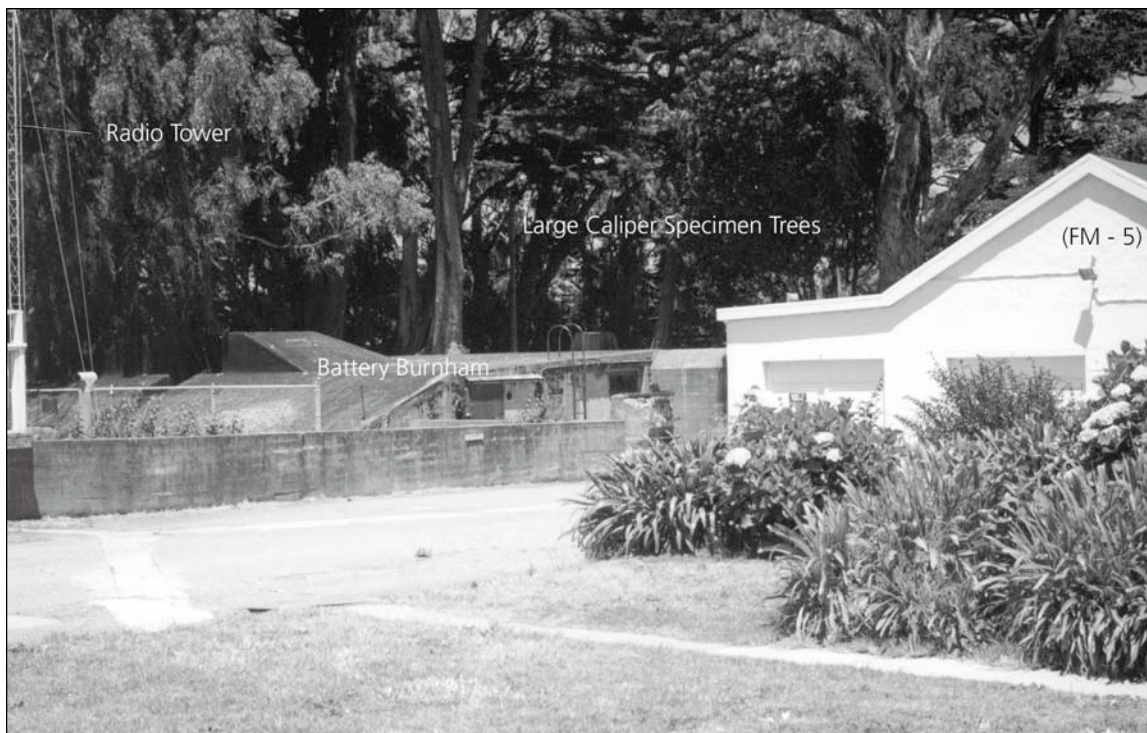
Figure 5.3.7: BLR Battery and Magazine (Battery Burnham). This fortification was part of the Endicott system of coastal defenses. Battery Burnham was armed with a single breech-loading rifle (BLR) between 1899 and 1909. A two-stall garage was built within its footprint c.1914. Contributing. Note the blocked view out to the bay from this historic artillery position, 12/02 -OCLP.
