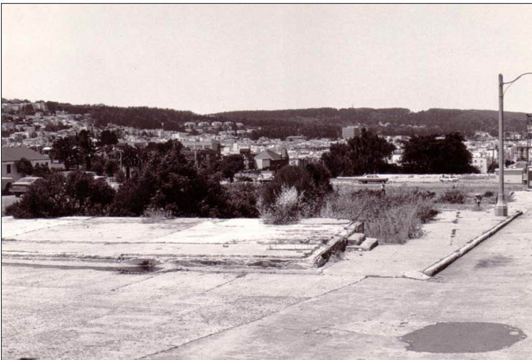
Figure 2.6.13: Many deteriorated temporary buildings were removed, leaving only the foundation, during the GSA administration of the site. Image c. 1970. NPS, GGNRA Archives, Richard Frear Collection.
