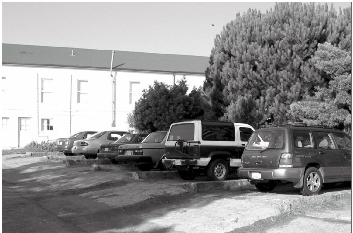
Figure 5.4.13: Stepped-Slab Garage Foundation Remnant. The garage once sitting atop this foundation was demolished between 1968 and 1972. Contributing. 7/02 - OCLP.
