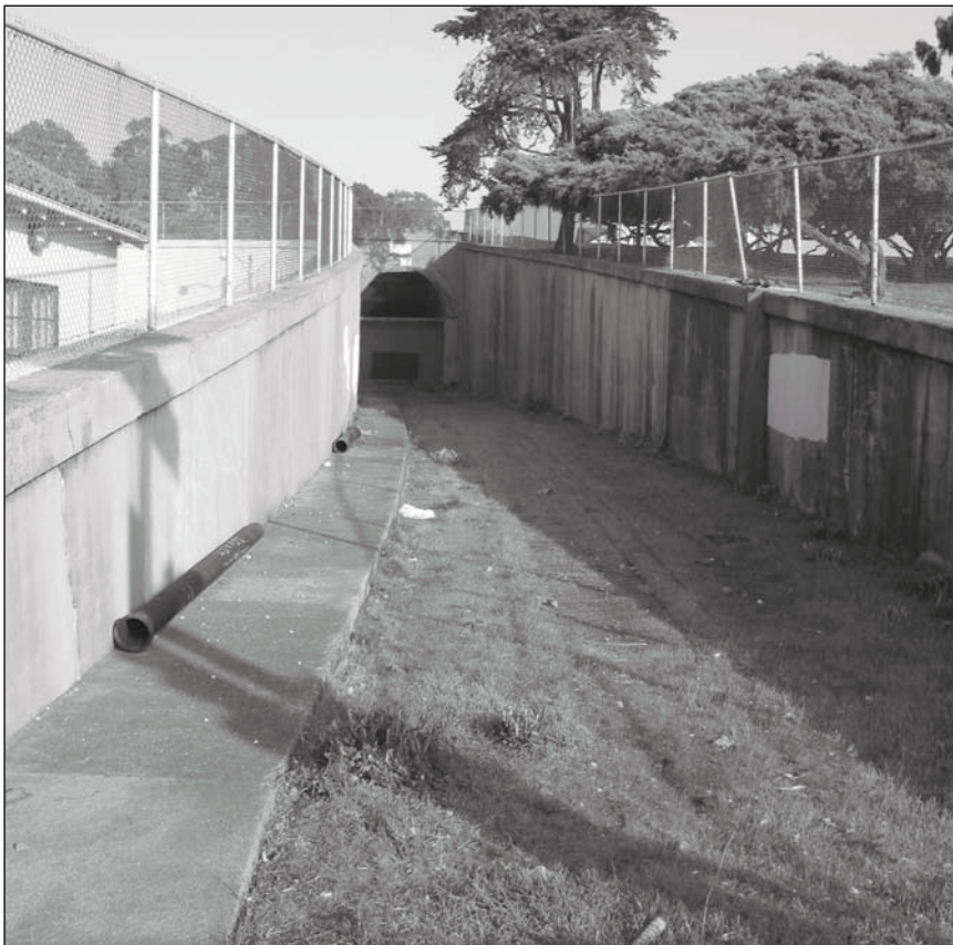
Figure 5.10.3: West Portal - Railroad Tunnel, (FM - 300). Constructed 1914. Contributing. 12/02 - OCLP.
