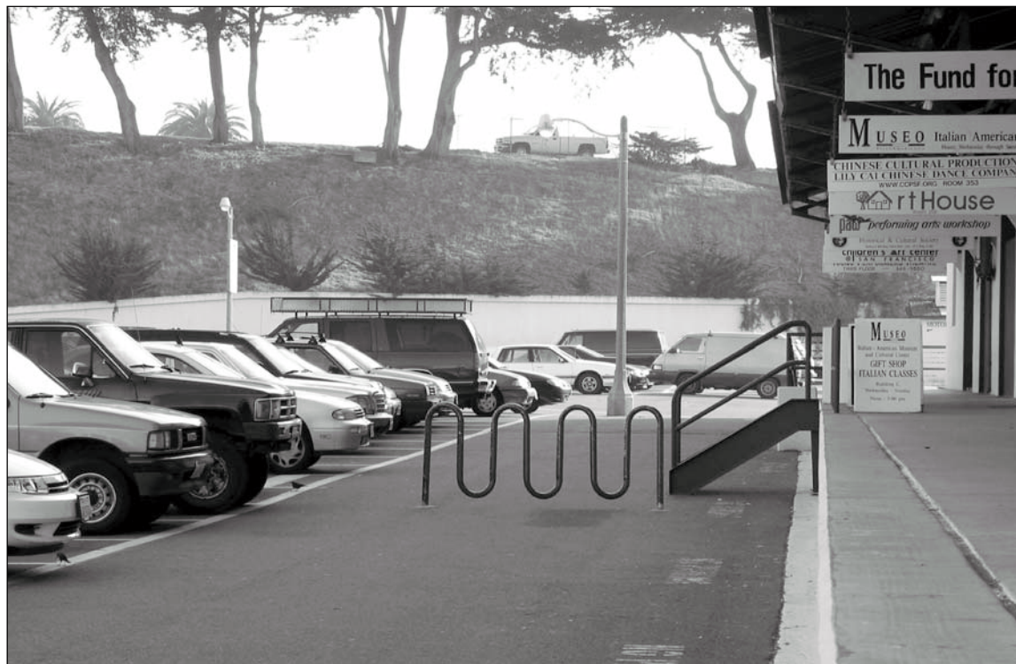
Figure 5.10.7: Bicycle Racks. Features such as this were installed during the 1970s and 1980s to facilitate the re-use of Lower Fort Mason as a cultural center. Non-contributing. Also note the tenant signage on the building. Non-contributing. 12/02 - OCLP.
