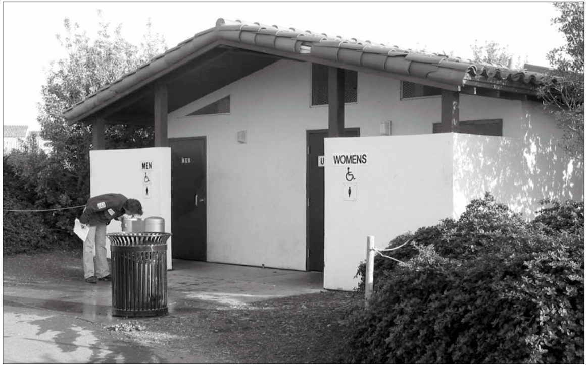
Figure 5.8.4: Great Meadow Comfort Station. This building was constructed by the NPS during the early 1990s as part of GGNRA's development of the Great Meadow at Fort Mason. Non-contributing. 12/02 - OCLP.
