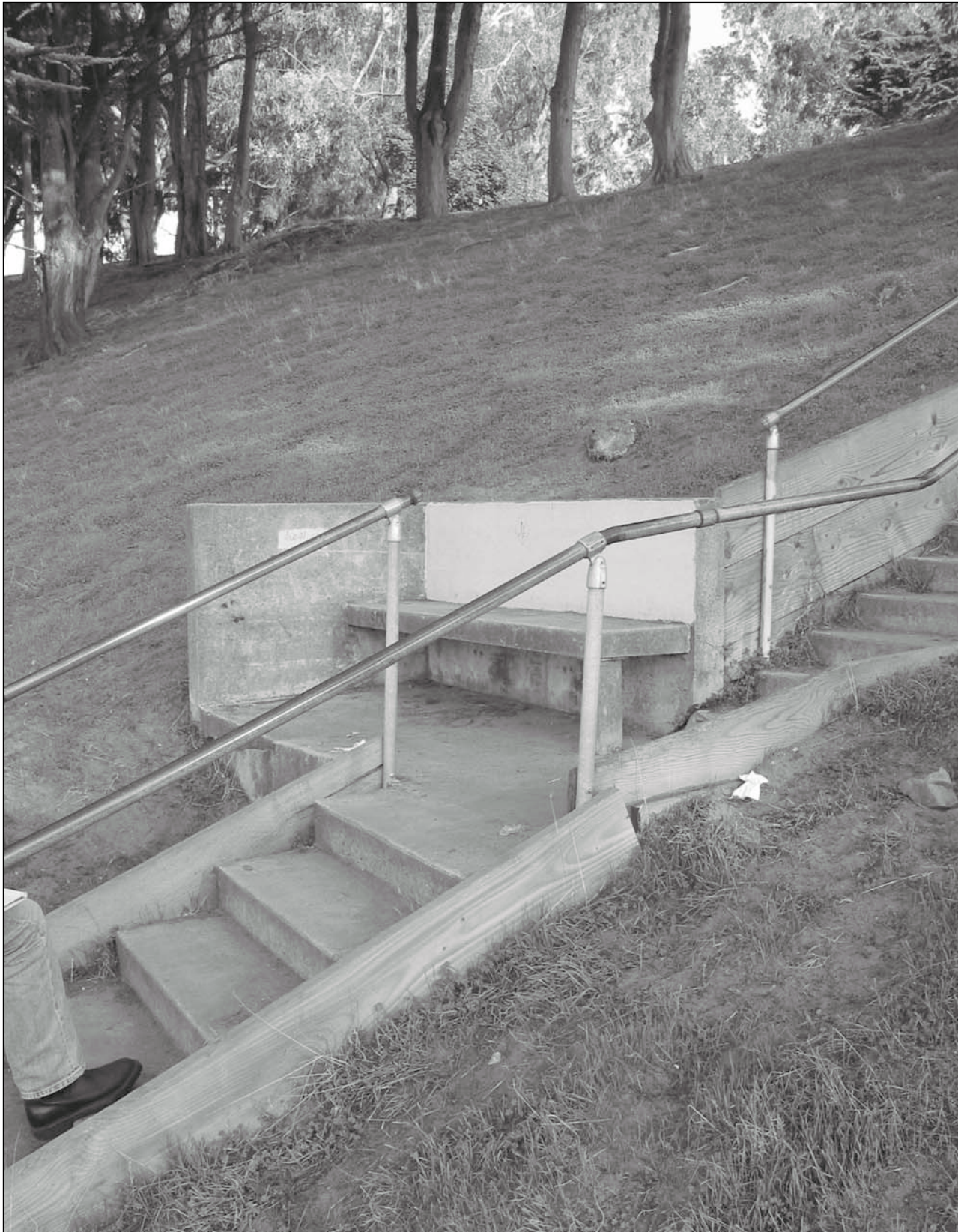
Figure 5.7.2: Stairs between Upper and Lower Fort Mason, (FM - 408). This set of stairs was built in 1938 replacing an earlier set of stairs first appearing on 1922 maps of the post. Contributing. Safety railings and wooden cribbing are non-historic. 12/02 - OCLP.
