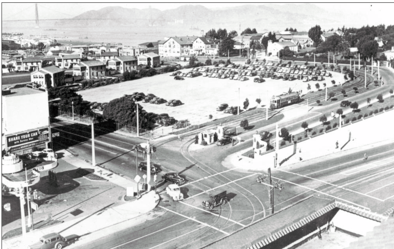
Figure 2.6.2: The parking lot at the corner of Bay Street and Van Ness Avenue remained free of buildings as the open lot was needed for the large number of civilian employees working on the base. Note the guard shack at the entrance and the planting of young Acacia trees along MacArthur Ave. Following the removal of the trolley tracks through the base in 1948, the iron gates at the Van Ness and Bay entrance were closed, limiting access to pedestrians only at that location. Image c.1942, NPS, GGNRA Archives, GOGA-2316, Interpretation Photograph Collection.
