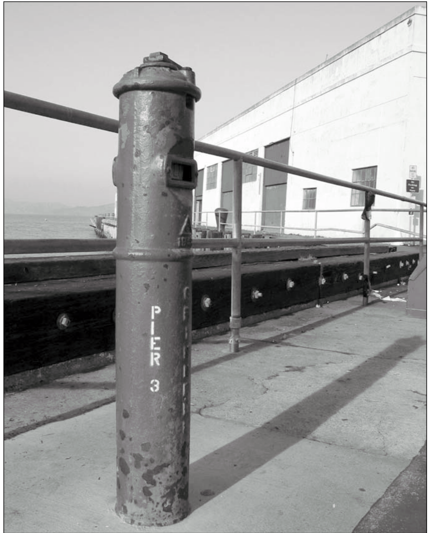
Figure 5.10.12: Waterfront Safety Railings and Fire Hydrant. Metal railings were added to the piers at Lower Fort Mason after it had ceased to serve as a working waterfront. Non-contributing. The fire hydrant fixture also shown above is recommended for contributing status, however this may require further evaluation. 12/02 - OCLP.
