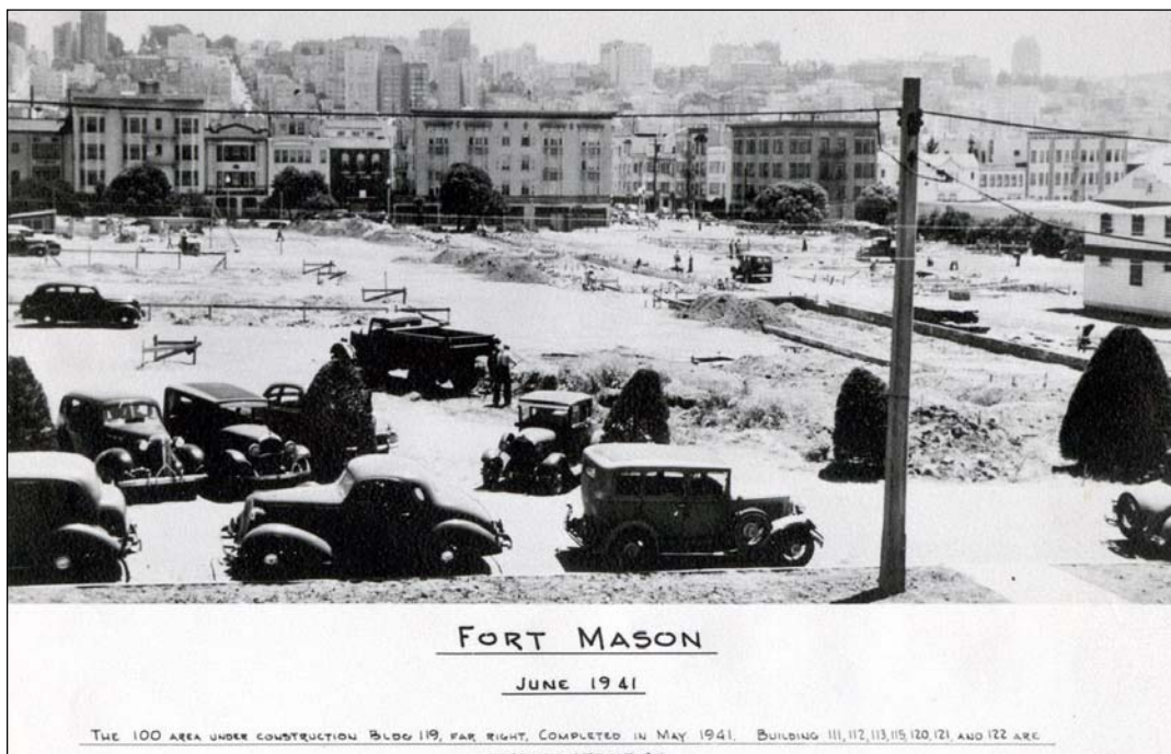
Figure 2.5.30: With a second worldwide conflict looming on the horizon, expansion of facilities at Fort Mason began even before the United States entry into war. This June 1941 image shows the construction of facilities taking place in the southwest quadrant of Fort Mason. NPS, GGNRA Archives, TASC Negative Collection, Box No. N16, 027, Fort Mason Folder, Acc/P# GOGA – 2266, Contact Print.
