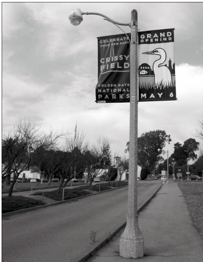
Figure 3.1.19: The most common type of street lighting found at Fort Mason is an exposed aggregate, cast-concrete light pole with a tubular steel bracket suspending the luminaire. It is known that these fixtures were installed post-WWII, but the exact dates of their installation have not yet been determined. 12/02 - OCLP.
