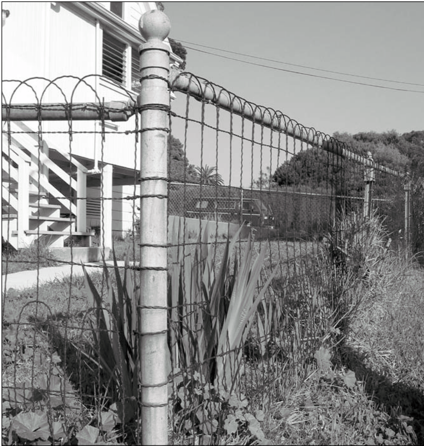
Figure 5.4.14: Woven-wire domestic fencing - NCO quarters. Contributing. 12/02 - OCLP
