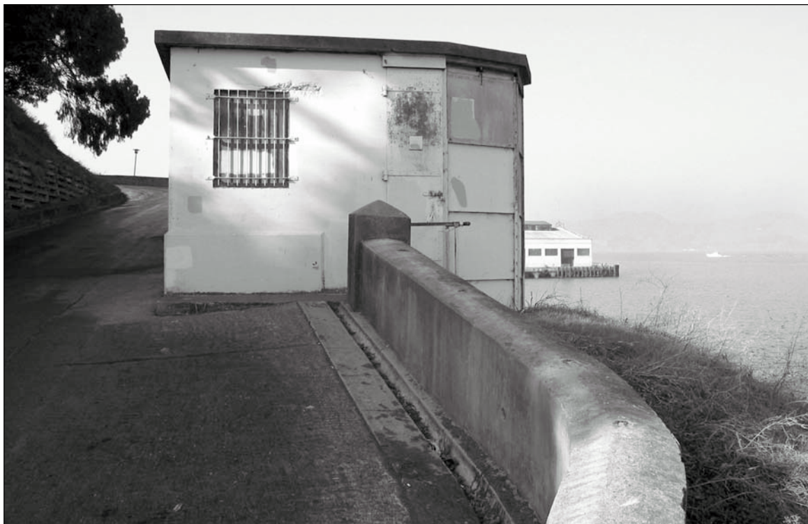
Figure 5.3.11: Searchlight shelter, (FM - 15). Constructed in 1911, prior to the invention of radar, this building and its searchlight continued the defensive mission of Fort Mason after the weaponry had been removed from Battery Burnham. Contributing. 12/02 - OCLP.
