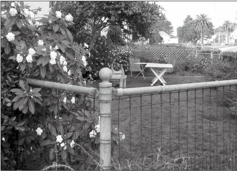
Figure 5.9.10: Woven-wire Domestic Fencing - Officers' Park. Contributing. 12/02 - OCLP.
