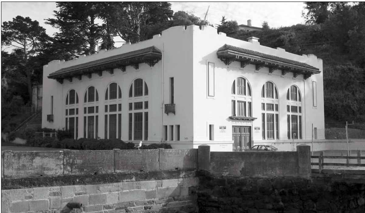
Figure 5.5.3: Emergency Pumping Station, (FM - 403). Contributing. 5/03 - OCLP.
