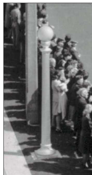
Figure 2.5.26: These decorative lamp posts were installed at Fort Mason in 1935 following the placement of overhead utility lines into underground conduits in 1934. The fixtures were Style #717 from the Union Metallic Lamp Standard Company. Detail from photograph of 8 March 1945. National Archives RG 111 - SC Box 156 - 311438.
