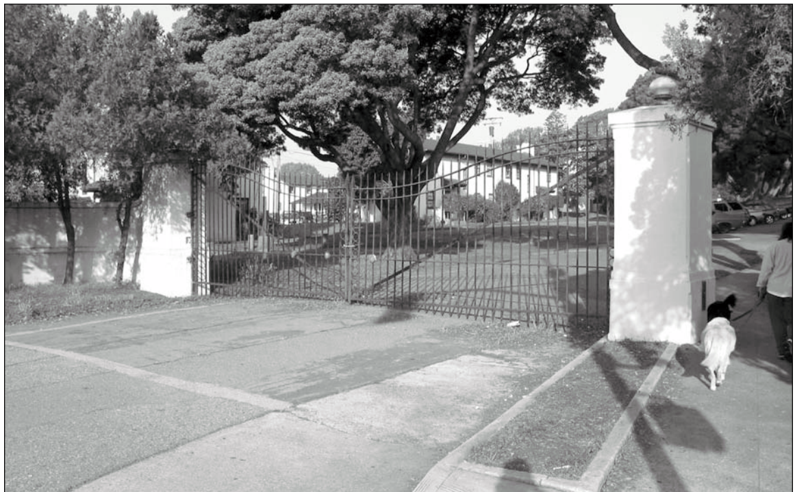
Figure 5.2.13: MacArthur Avenue Entrance Gate. This entrance gate was built during the 1930s as part of WPA "make-work" economic relief efforts prior to WWII. Contributing. 12/02 - OCLP.
