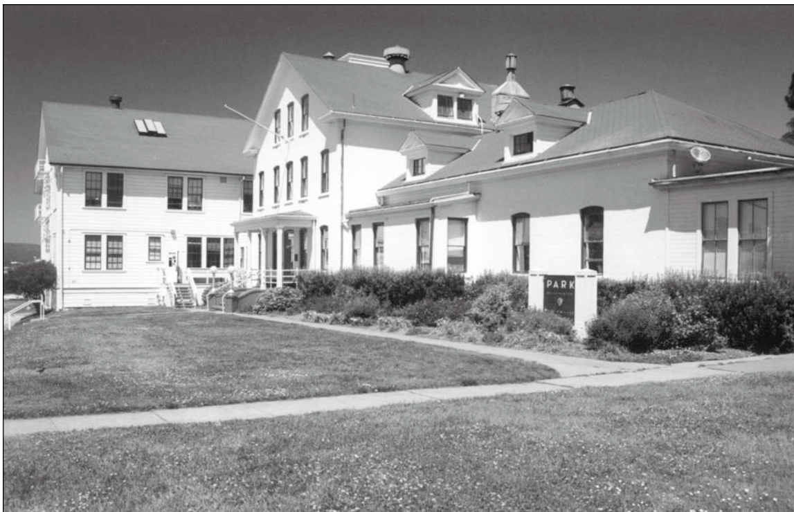
Figure 5.4.7: Foundation Plantings. The foundation planting on the south facade of FM - 201 was replaced by the NPS. The planting is accompanied by a large park sign identifying this building as GGNRA headquarters. Non-contributing. 7/02 - OCLP.
