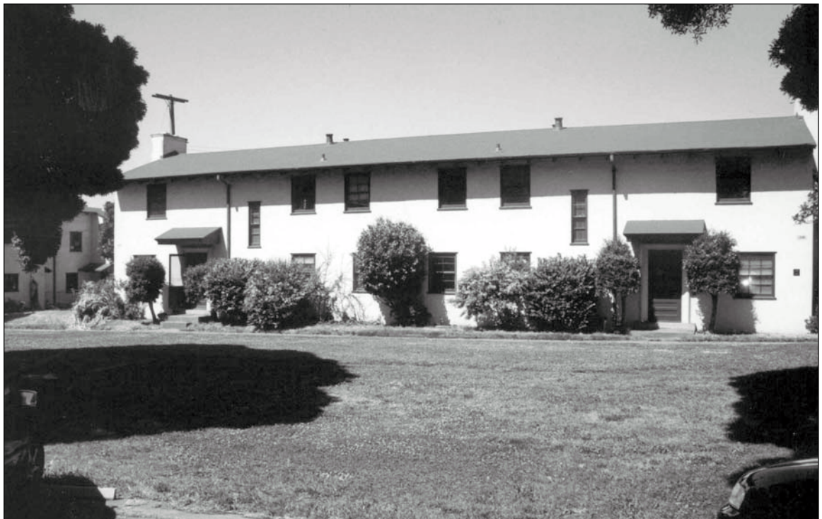
Figure 5.9.5: Foundation Plantings - the "Quad." Foundation plantings are consistently overgrown in the "Quad" portion of the South Expansion landscape character area. Requires further evaluation. 7/02 - OCLP.
