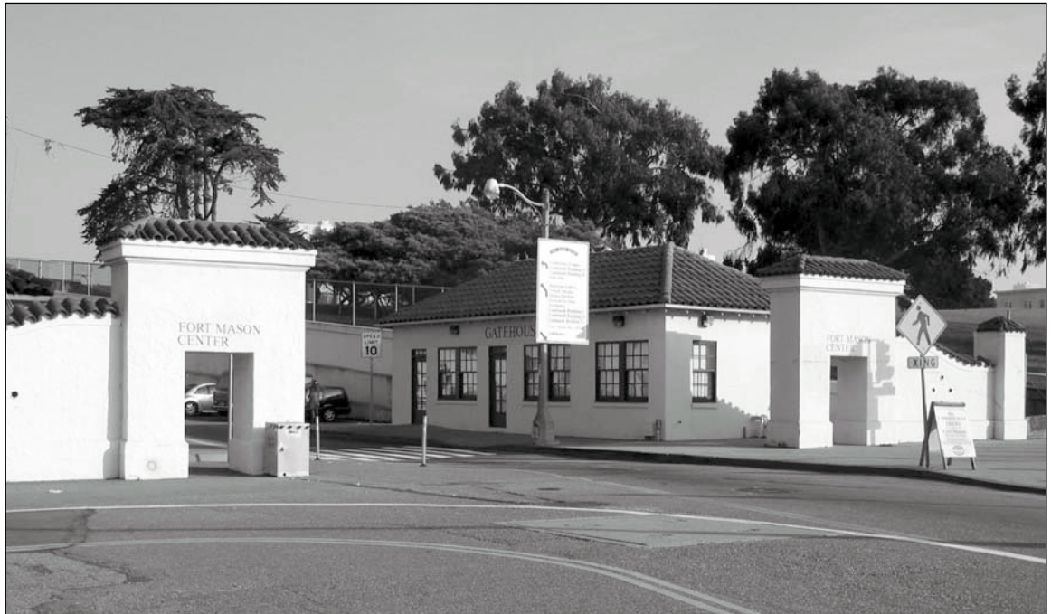
Figure 5.10.4: Lower Entrance Gate (FM - 301). This gateway into Lower Fort Mason was constructed c.1926, controlling access into what was once the Army's second largest shipping and logistical center. Contributing. 12/02 - OCLP.
