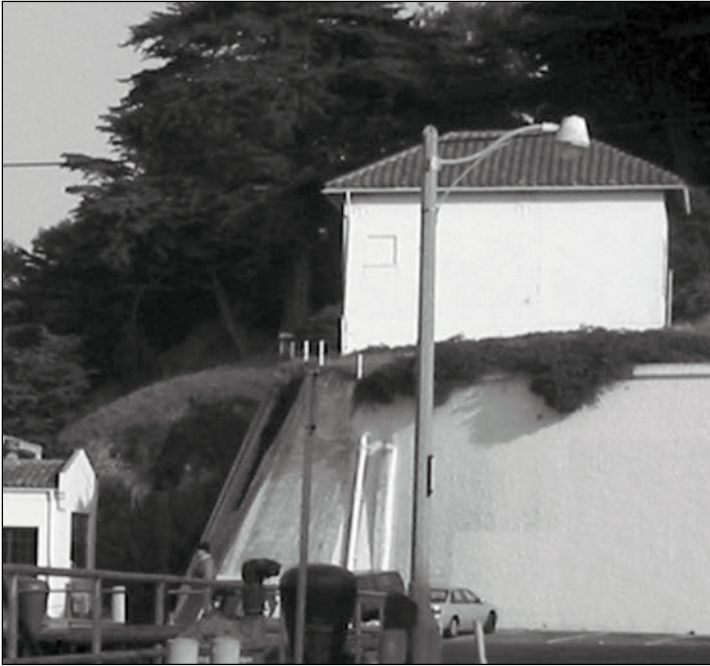
Figure 5.7.5: Transformer house, (FM - 248). This building was constructed c.1913 to serve the Army's transport docks at Lower Fort Mason. Contributing. 12/02 - OCLP.
