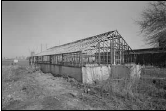
Figure 6.11 The greenhouse on Island One prior to its demolition. The recreation shelter is shown in the right background. March 1985. (Library of Congress, Prints and Photographs Division, HABS, NY, 31-ELLIS, 1A-1 [Stephen Zane, NY-6086-A-1])
