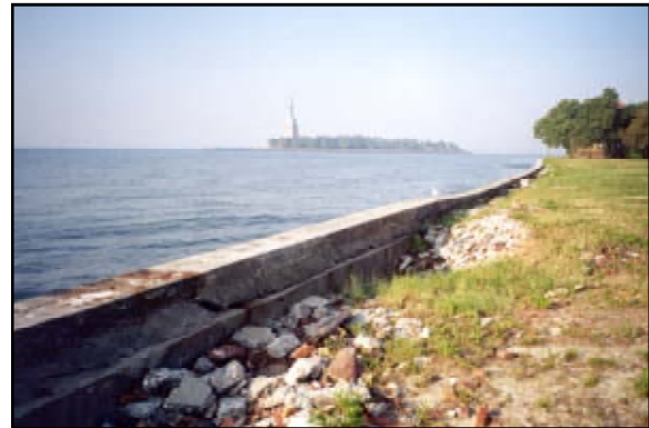
Figure 6.18 Some sinkholes continue to exist along the seawall, including this section on the south side of Island Two. August 2002. (Photo by author)
