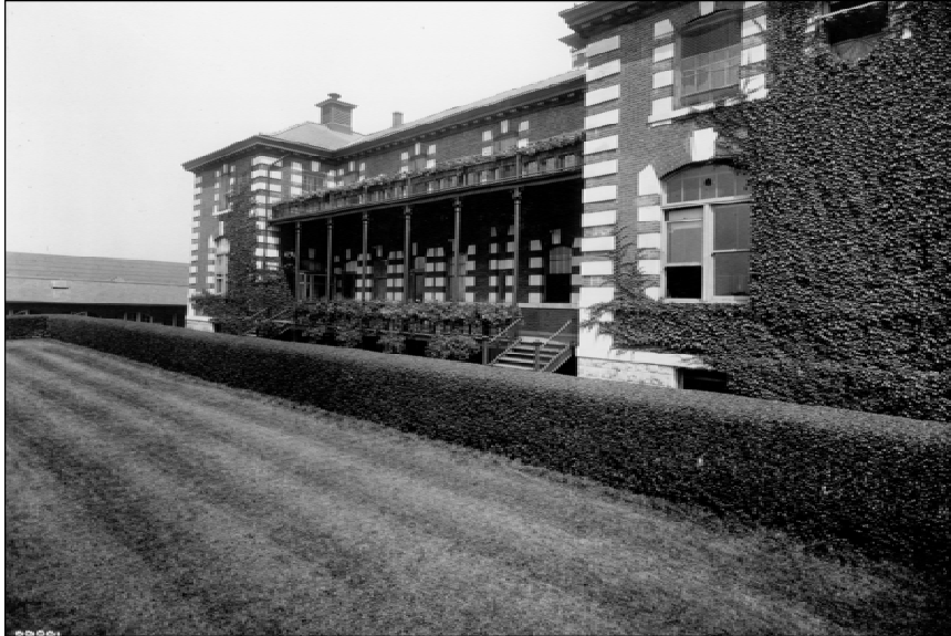
Figure 4.5 Ornamental vines, shrubs, and window boxes filled with flowers embellished the front facade of the kitchen and laundry building. Circa 1913. (William Williams Collection, #28881, Photography Collection, Miriam and Ira D. Wallach Division of Art, Prints and Photographs, The New York Public Library, Astor, Lenox and Tilden Foundations)
