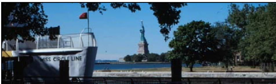
Figure 6.32 View toward Liberty Island from Island One. 1999. ("Cultural Landscapes Inventory")
