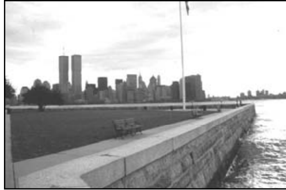
Figure 6.26 A view of the concrete and granite seawall surrounding all three islands. 1999. (“Cultural Landscapes Inventory”)
