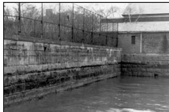
Figure 5.36 The INS added this fence in the 1940s west of the new immigration building around the site of the former tennis courts. It remained in place until the 1970s. (BOSO Engineering Files, 1978)
