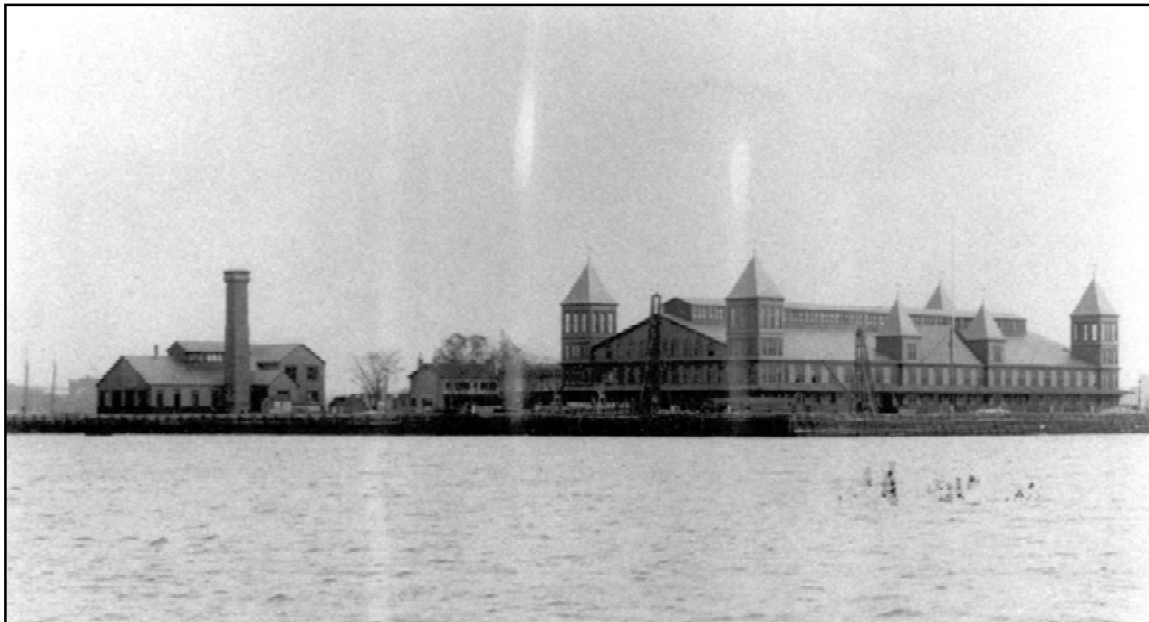
Figure 2.2 The first immigration station on Ellis Island. The buildings from left to right are the tank and coal house, boiler house, surgeon's quarters, and main building. 1892. (National Archives and Records Administration, RG121-BCP-37D-5)
