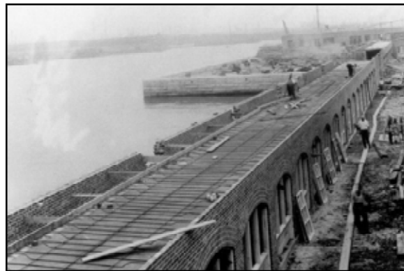
Figure 5.9 Construction of the covered masonry walkway between Island Two and Island Three. July 26, 1935. (National Archives and Records Administration, RG121-BCP-38B-28)
