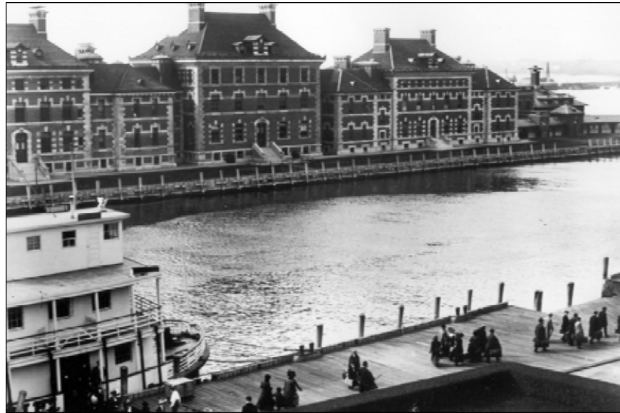
Figure 4.11 Island Two is viewed from Island One in this circa 1913 photograph, showing (left to right) the new hospital extension, administration building, and the original main hospital building. The boardwalk, wooden cribwork seawall, and fender pilings along the ferry basin on Island One are shown in the foreground. (STLI Library, 19.5, #14)
