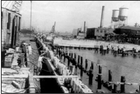
Figure 5.10 A new seawall and pilings were added to accommodate construction of the new immigration building on the northwest side of the island. September 24, 1934. (National Archives and Records
