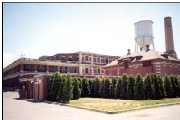
Figure 6.30 Arborvitae hedges ( Thuja species ) are used to screen the fuel tanks and HVAC units in the utility area on Island One. August 2002. (Photo by author)
