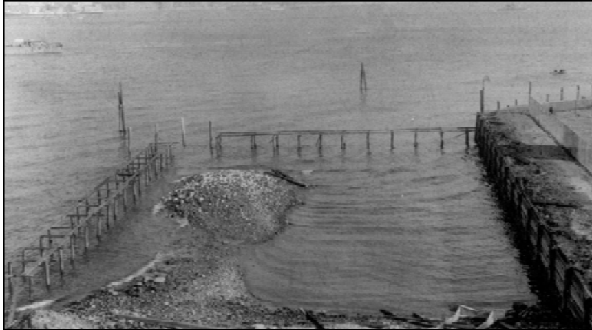
Figure 5.14 This area northeast of the main immigration building adjacent to the recreation yard was the last section of landfill added to the island. Its addition increased the available space for immigrant recreation. It may have been constructed as part of Federal Project No. 61. April 2, 1934. (National Archives and Records Administration, RG121-BCP-38C-12)
