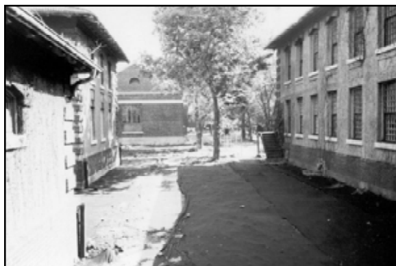
Figure 6.17 After vegetation clearing, crews installed landscape fabric to deter vegetation from resprouting in the courtyard areas. This recently cleared space is between the nurses' quarters and wards 11 & 12 on Island Three. August 2002. (Photo by author)
