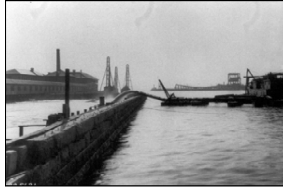
Figure 5.11 After seawall completion, dredging and fill created a land area for the new immigration building. The old wooden covered walkway is shown in the background. October 24, 1934. (National Archives
