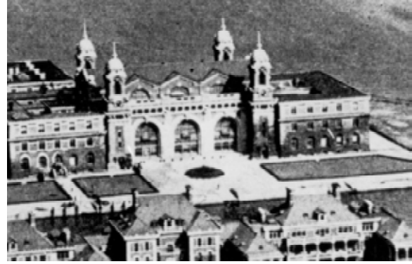
Figure 5.6 One of the improvements initiated by Commissioner Corsi was the replacement of the entry portico in front of the main immigration building with a large circular planting bed. January 9, 1934. (STLI Library, 25.2, #8, copy also located at National Archives and Records Administration, RG90-G-90-16)
