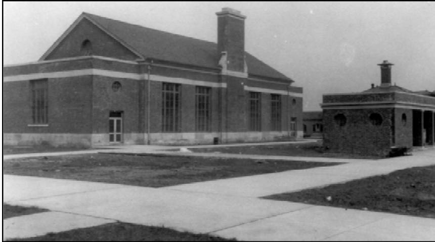
Figure 5.15 Newly completed recreation building and shelter between Islands Two and Three. February 26, 1937. (National Archives and Records Administration, RG121-BCP-38B-3)
