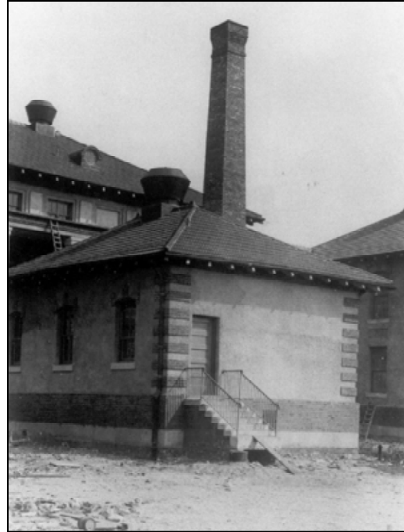
Figure 4.16 Upon completion of the mortuary (animal house) on Island Three, there was still a considerable amount of fill needed to raise the island's grade to its planned elevation. Notice the distance between the bottom of the staircase and the rough grade prior to the addition of topsoil fill. October 14, 1907. (National Archives and Records Administration, RG121-BCP-38A-3)
