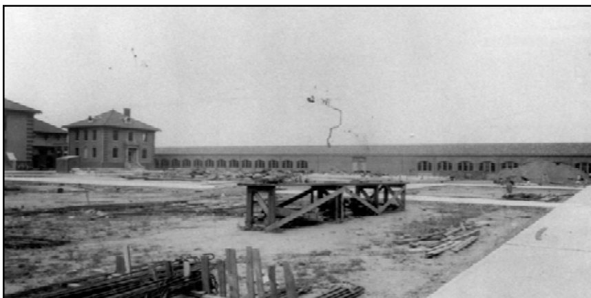
Figure 5.19 Newly poured concrete walkways in the recreation area between Islands Two and Three. June 25, 1936. (National Archives and Records Administration, RG121-BCP-38B-26)
