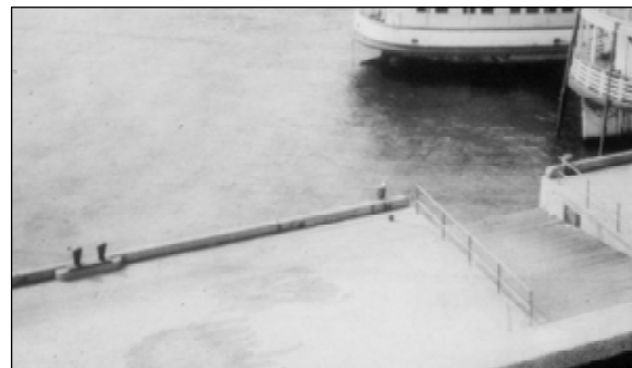
Figure 4.25 Iron mooring cleats along the seawall, as shown in the lower left of the photo, assisted with docking ships. They were added to the landscape sometime between 1907 and 1913. Circa 1915. (STLI Library, 19.6, #29)
