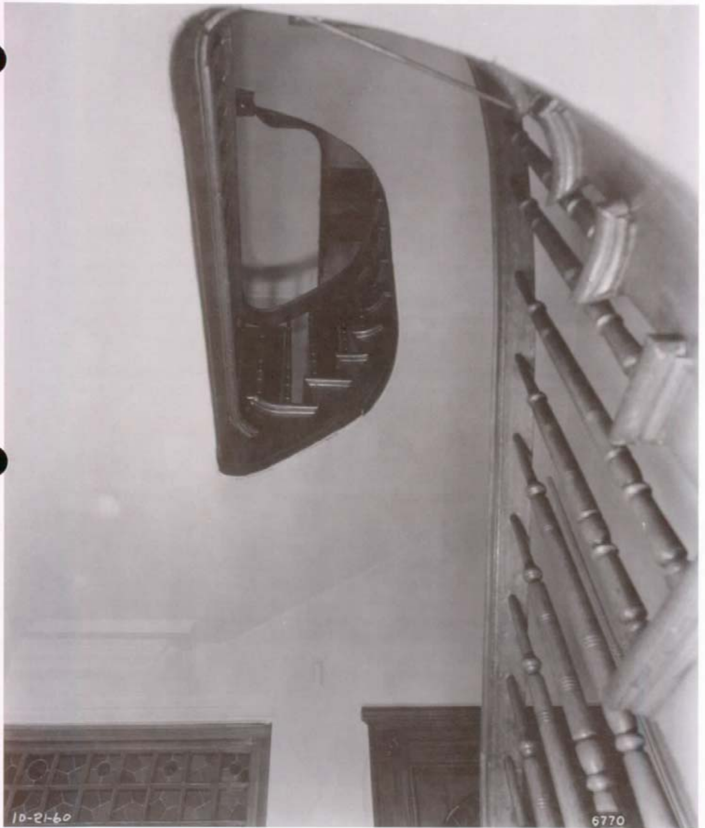
Figure 116. South part of Service Hall (Room 117), looking up at the Service Stairway, 1960.
