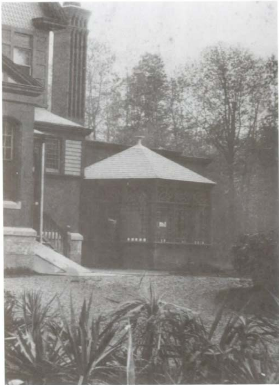
Figure 7. Detail of Figure 6, showing the "well house."
