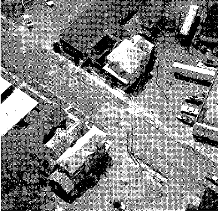
Figure 3 This aerial photo, taken April 26, 1986, of a portion of South Williams Street shows The Wright Cycle Company building immediately in the foreground. The two houses to the south of the building and the two houses across the street on the west side of South Williams are also part of the West Third Street Historic District.
