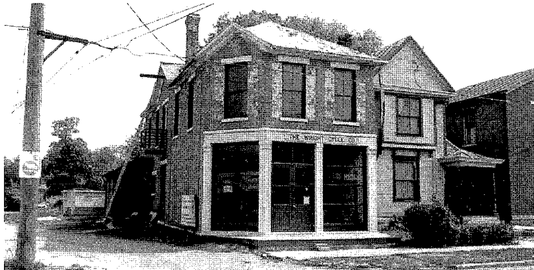
Figure 4 View of The Wright Cycle Company building in 1986 with most of the restoration work completed. Photo courtesy of Aviation Trail, Inc.
