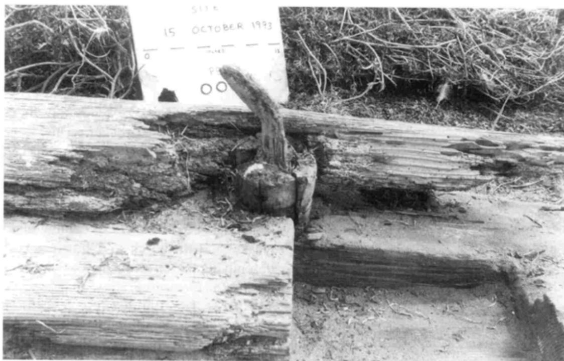
Figure 4.40. Iron fastener driven through an oak plug on feature PB-002. NPS photo by Matt Russell.
