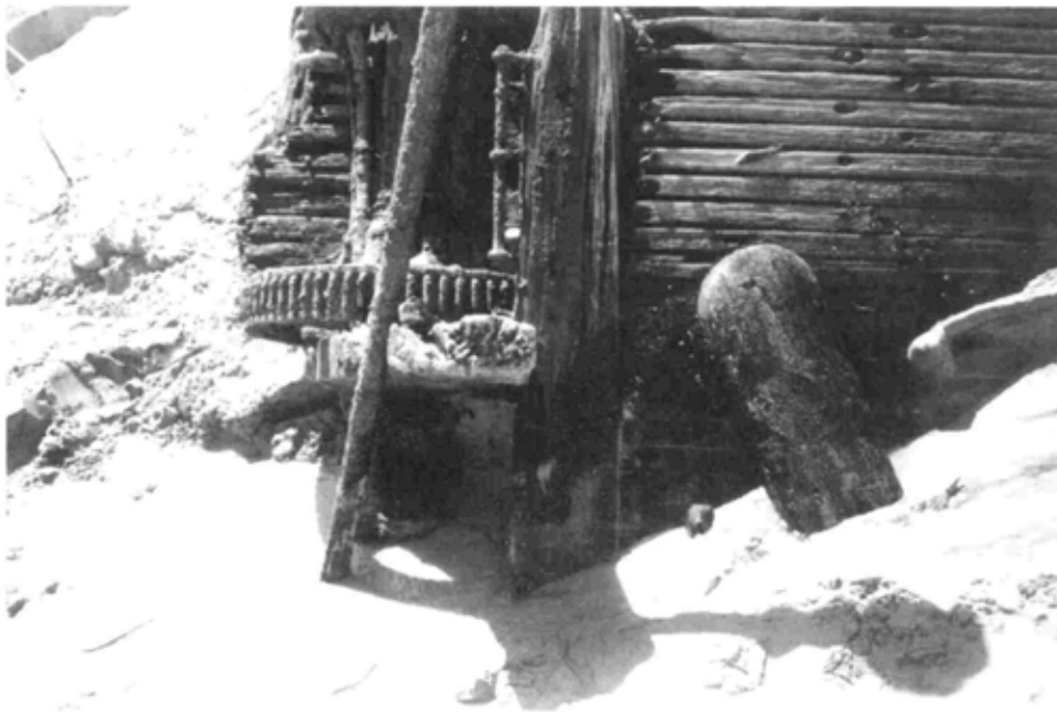
Figure 4.81. Top view of the aft end of the forecastle deck. The aft-most forecastle deck beam is the vertical timber in the center of the photo. The windlass is to the left, mounted on the main deck below; the starboard cathead is the angled timber to the right. NPS photo by Matt Russell.
