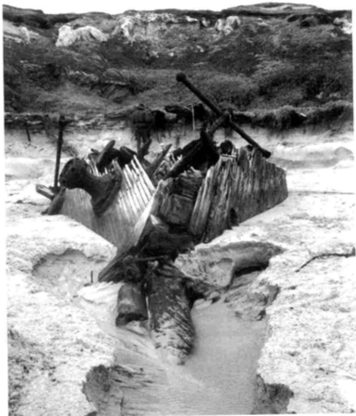
Figure 4.69. Comet site in April 1999, looking straight towards the bow, which is canted to the left in this photo. The forecastle deck is to the left, port side outer hull planking to the right and the bowsprit is in the bottom of the photo. NPS photo by Matt Russell.
