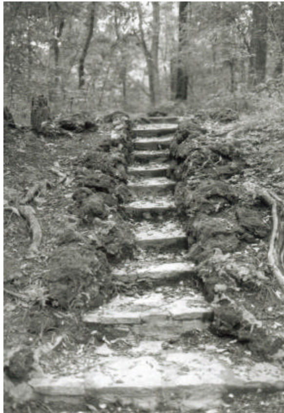
CCC STONE STEPS Pavilion Springs/Travertine Creek Trail
