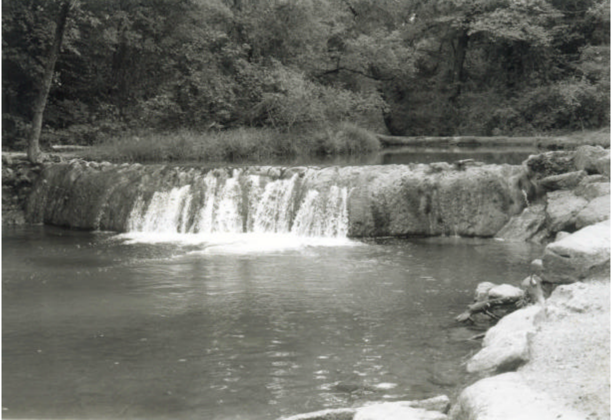
RECREATIONAL DAM, GARFIELD FALLS
