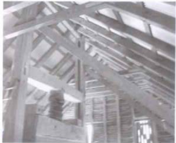
Figure 30 View southwest of roof framing installed in 1996. (NPS-SERO-CRS, 2001)
