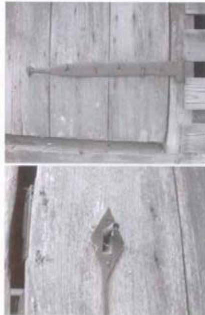
Figure 35 View of hinge and escutcheon on Door D. (NPS-SERO-CRS, 2001)
