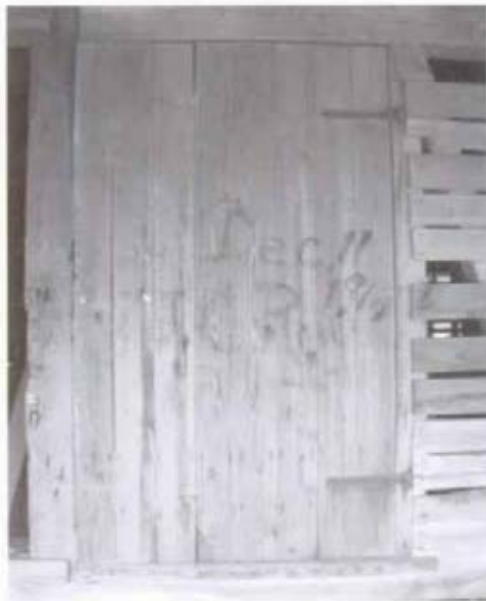
Figure 33 View of Door A, added to second floor around cotton press. (NPS-SERO-CRS, 2001)
