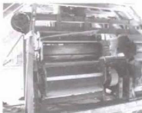
Figure 41 View of Continental gin stand on second floor. (NPS-SERO-CRS, 2001)
