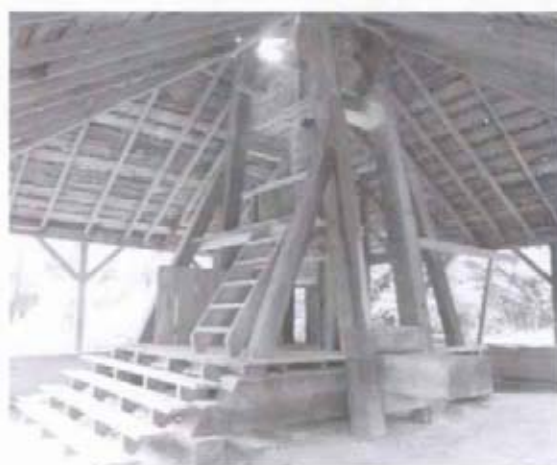
Figure 3 View of interior of Westville press building. Antebellum presses did not always include the surrounding shed, which would have facilitated operation of the press in inclement weather as well as protecting the screw from the elements. (NPS-SERO-CRS, 2001)
