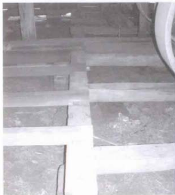
Figure 21 View of floor framing at east end of Gin Barn. (NPS-SERO-CRS, 2001)
