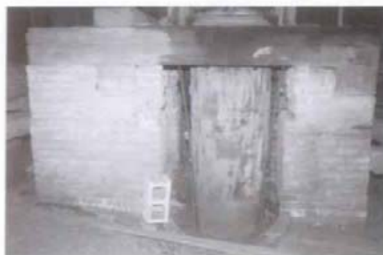
Figure 43 View of hydraulic cylinder and supporting brick piers for press. (NPS-SERO-CRS, 2001)
