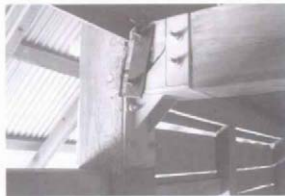
Figure 20 View of typical beam/post connection, reinforced with metal brackets in 1996. (NPS-SERO-CRS, 2001)
