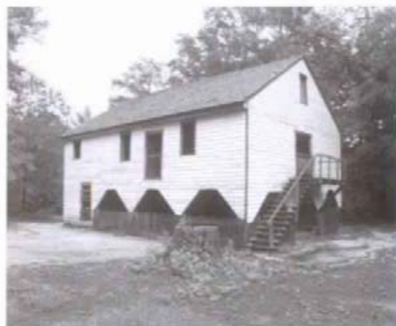
Figure 1 Gin House at Westville, c. 1840. The open first floor houses the drive wheel and sweeps for draft animals. Cotton was carried in baskets to the second floor for ginning before falling into the lint room, which is at the left end of the building in this image. (NPS-SERO-CRS, 2001)
