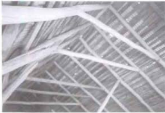
Figure 27 View of original pole-rafter roof in 1995. (NPS-SERO-Architecture, 1995)
