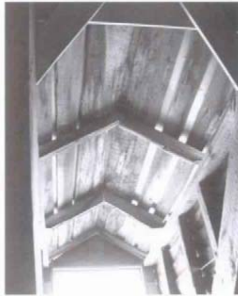
Figure 29 View of south dormer with original framing and decking intact. (NPS-SERO-CRS, 2001)
