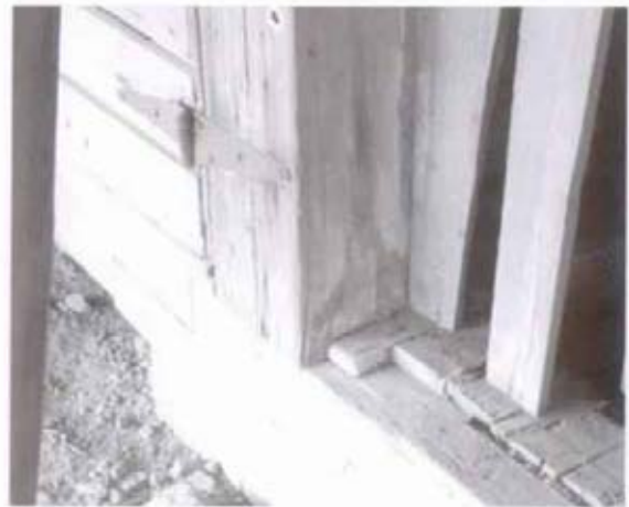
Figure 31 View of original flooring at south side of lint room. (NPS-SERO-CRS, 2001)
