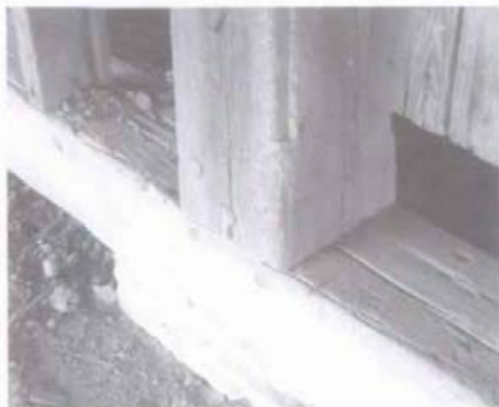
Figure 19 View of typical sill and post with historic splined connection intact. (NPS-SERO-CRS, 2001)
