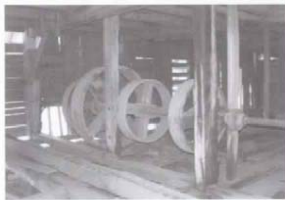
Figure 38 View of belt-driven flywheels at east end of barn, which would have been connected by leather belts to the engine outside the building and to the machinery inside. (NPS-SERO-CRS, 2001)
