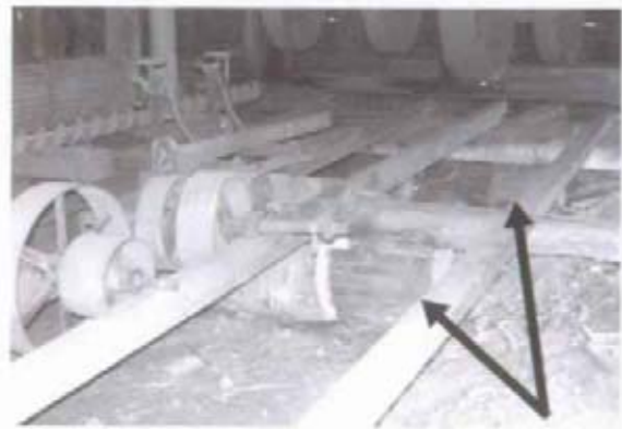
Figure 17 View of early brick piers under machinery room floor. (NPS-SERO-CRS, 2001)
