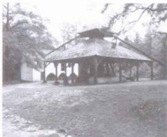
Figure 2 Westville cotton press, c. 1864. Note sweeps or “buzzard wings” above the roof. (NPS-SERO-CRS, 2001)
