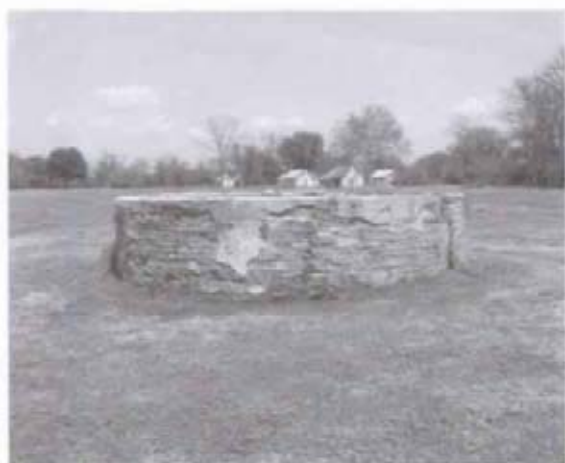
Figure 47 View to northeast of cistern at Gin Barn. (NPS-SERO-CRS, 2001)
