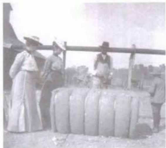
Figure 48 View of Prud'hommes' gin at Oakland, showing elevated flue to transport seed from gin to seed house. A similar apparatus would have been used at the Magnolia gin, but has now disappeared. (NPS-SERO-CRS, 2001)
