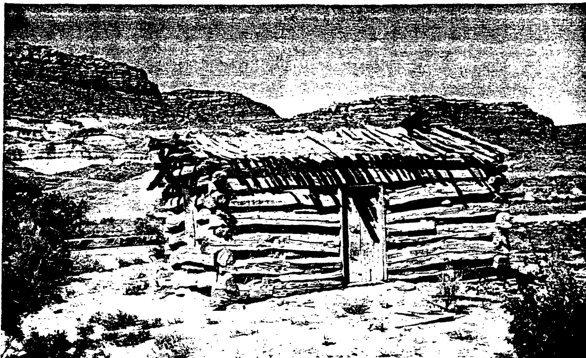
Pioneer log cabin at Paria. No one now lives at Paria but some of the old buildings are used by present day cattlemen
