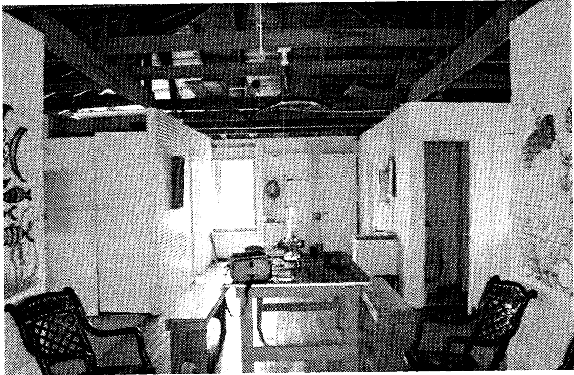
Figure 24 View to southeast showing back door now opening to the garage. (NPS-SERO-CR, 2003)
