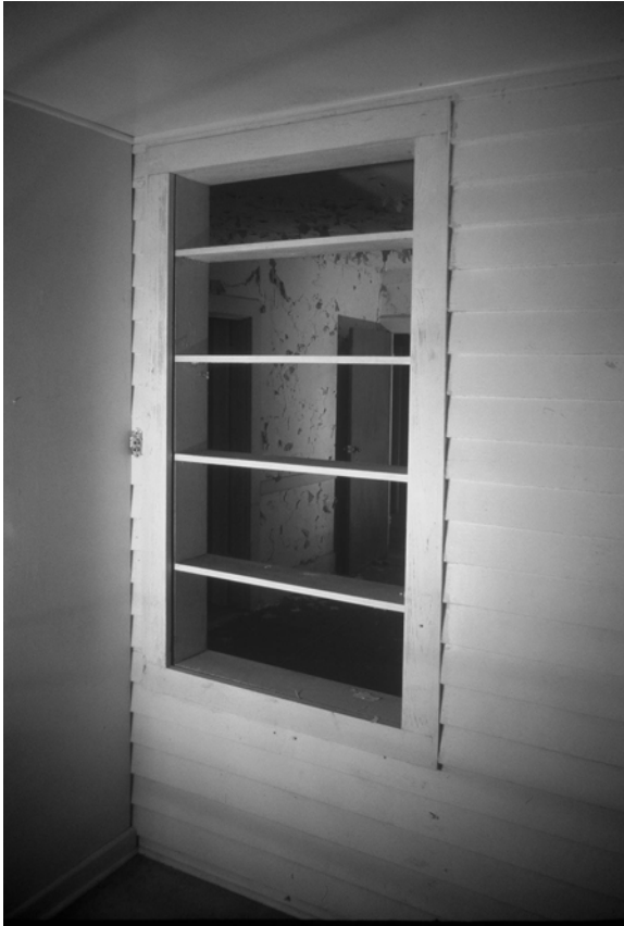
Figure C-31 Bookshelf created in original window opening in Room 111
