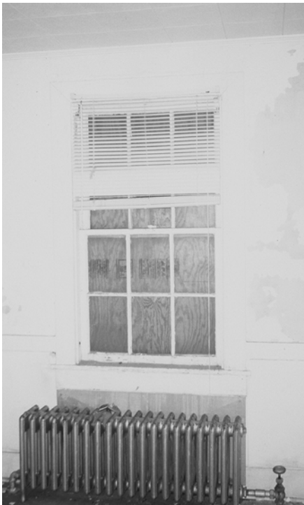
Figure C-7 Six-over-six window and radiator, probably both dating to 1925
