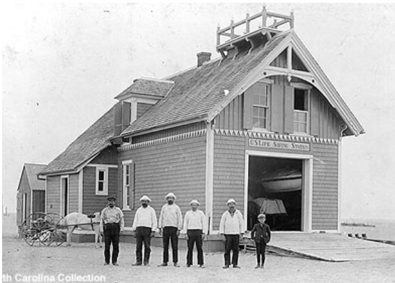
Figure A-5 1876 Type station at Big Kinnakeet, c. 1890s, North Carolina Collection, University of North Carolina – Chapel Hill, negative no. 83-659
