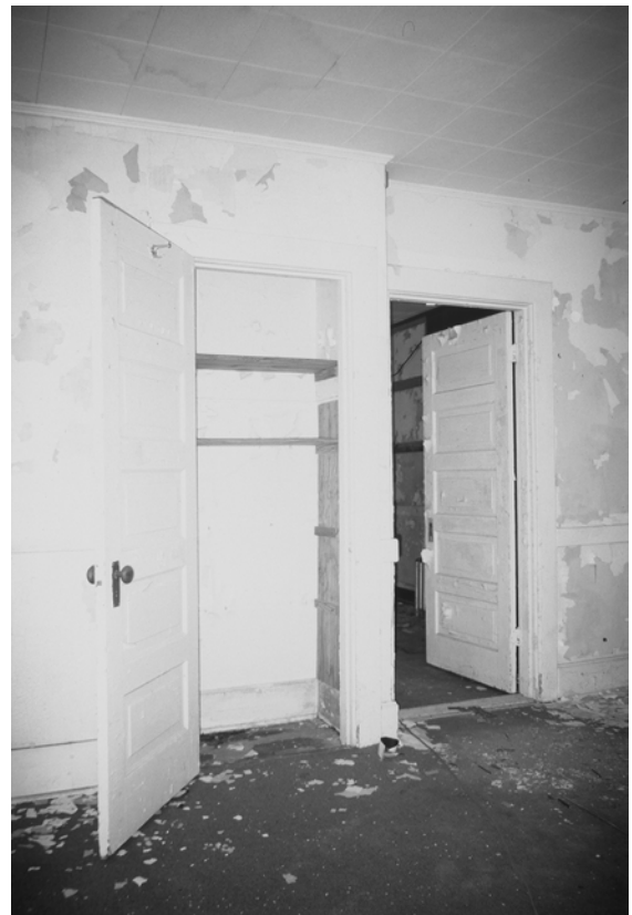
Figure C-26 Closet in Room 104
