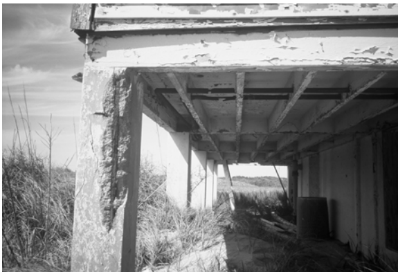
Figure C-4 Porch foundation and floor framing
