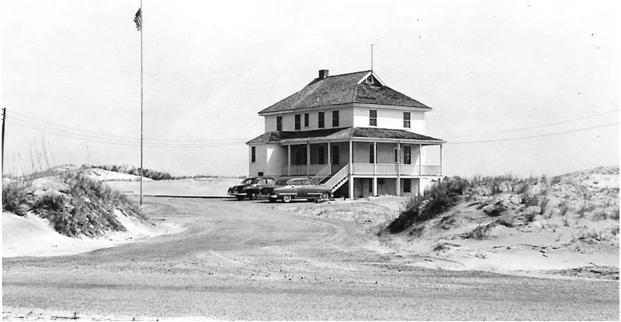
H.22 1925 Station from the southwest, May 1956. Label – “Neg. No: 56-204, Date: 5/4/56, Print File: St/A, General Description, Location, Other pertinent Data: Cape Hatteras National Seashore Headquarters, Negative by: W. V. Watson, Large Print: No” Shows stairs to porch added by NPS, and existing door into stair tower.
