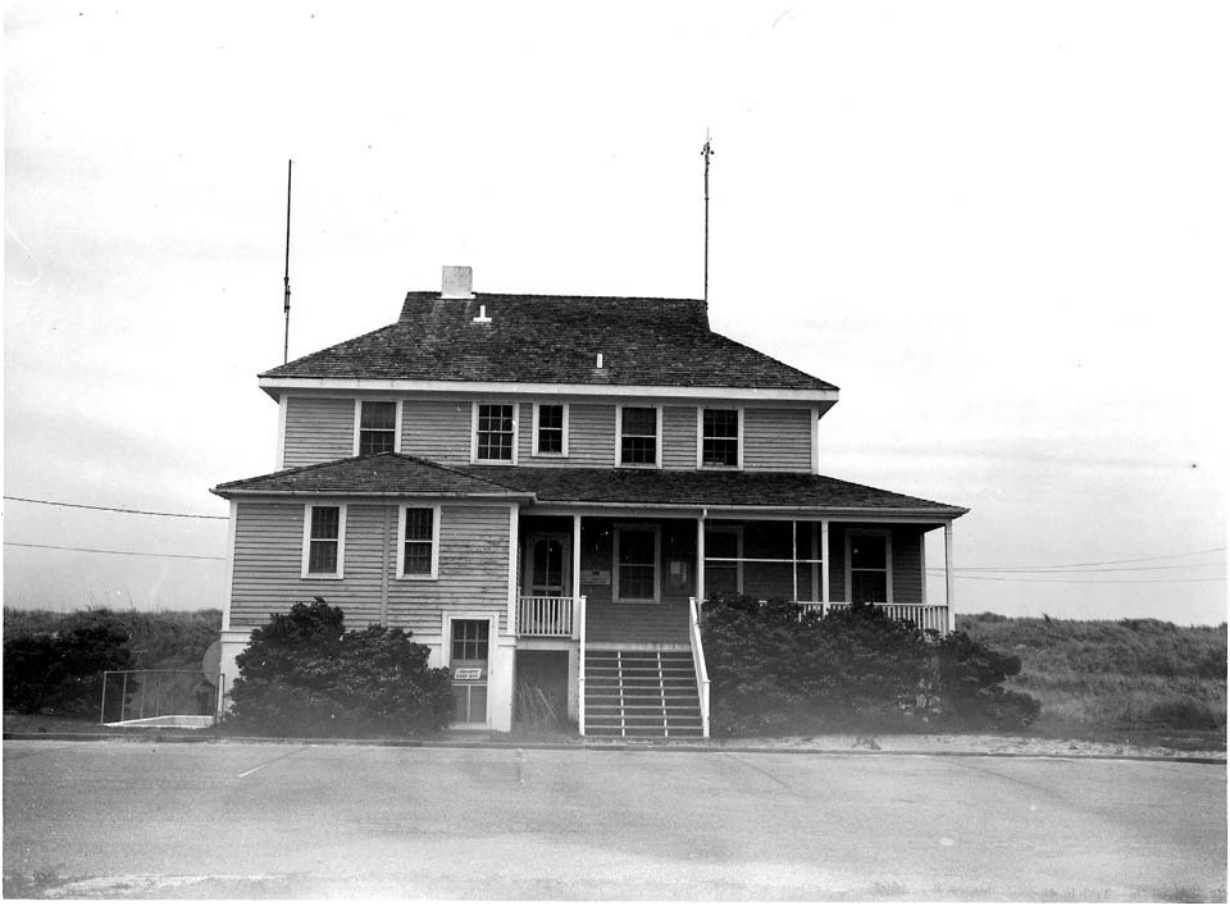
H.24 1925 Station from the west, ca. 1971. Label “CG Station (Ranger Station) 1971.” Shows restrooms added north of stair tower, stair to porch relocated northward, porch on south façade enclosed.
