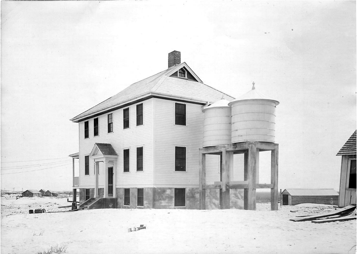
H.1 1925 Station from the northeast ca. 1928. One of a series of four images taken at the same time. Journal entry for July 7, 1928 notes that Frank L. Toon arrived to take picture of the station and crew. Shows station as originally constructed with four basement windows on east elevation, water storage tanks aligned north-south, and the oil house to the north.
