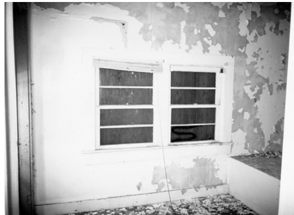
Figure C-29 Paired windows in the south wall of Room 109
