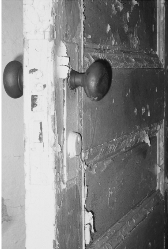
Figure C-11 Early back door's mortise lock
