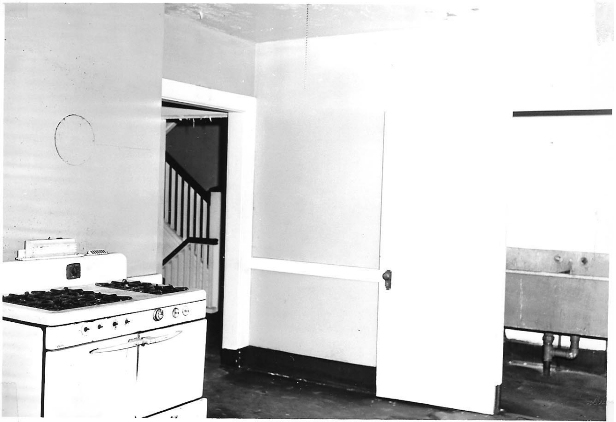
H.19 1925 Station kitchen in northwest corner of first floor, March 30, 1954 by J.C. McCabe, Photo no. 4. Label: "Former kitchen on main floor, Bodie Island C.G. Station." Shows large utility sink in area that would later become the entry hall for the NPS.
