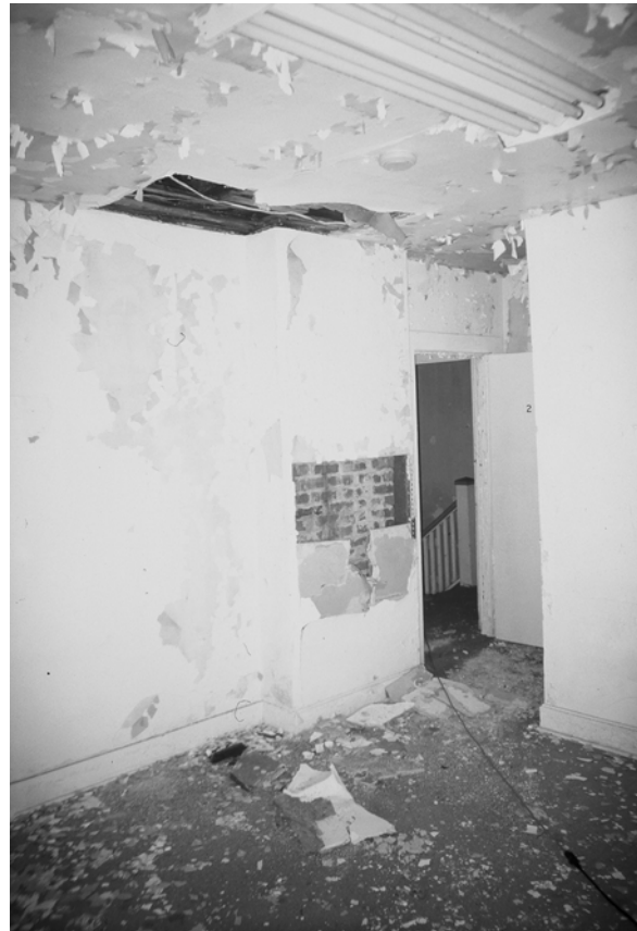
Figure C-36 Chimney in Room 205
