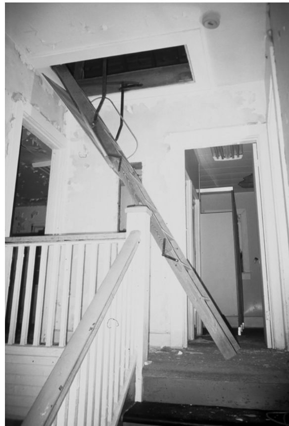
Figure C-34 Drop-down, folding attic stair in Room 202
