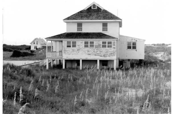
Figure B-16 Station from the south, with relocated 1879 Life-Saving Station at left, December 1986, NPS archives, Outer Banks Group
