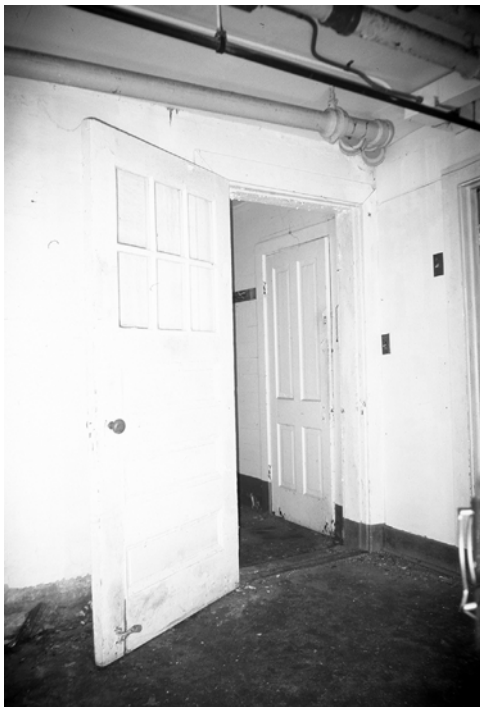
Figure C-10 1933 Doorway leading from the added west stair tower (Room 007)
