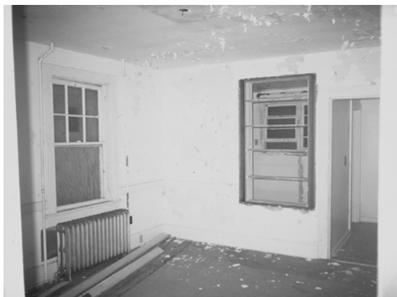
Figure C-23 Southeast corner of Room 101 with original window converted to an open bookcase
