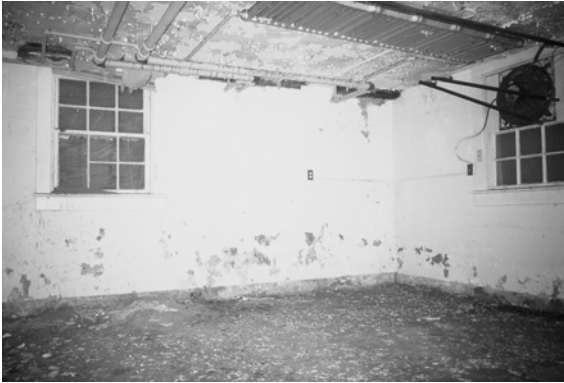
Figure C-9 Southeast corner of Room 001
