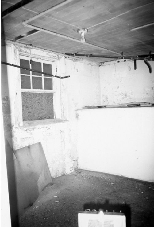
Figure C-16 Northeast corner of Room 004
