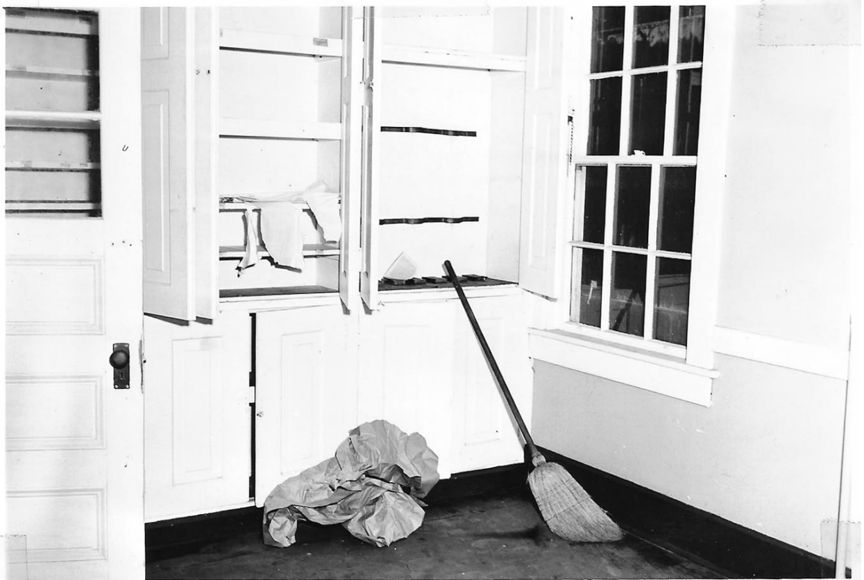
H.16 1925 Station north wall southeast room first floor, March 30, 1954 by J.C. McCabe, Photo no. 1. Label: "Reception Room Bodie Island G.G. Station. (Park Headquarters)." Shows cabinets in original location.
