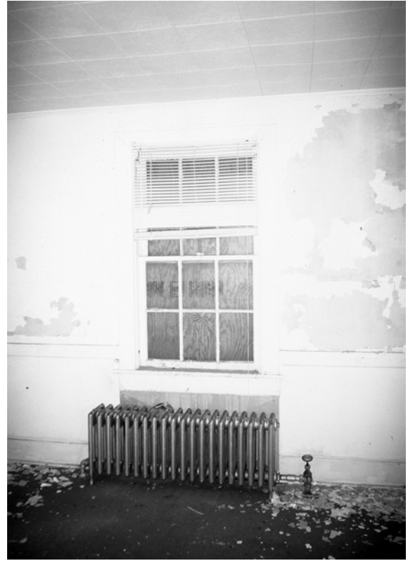
Figure C-25 Original window, Room 104
