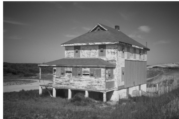
Figure C-3 Station from the southeast
