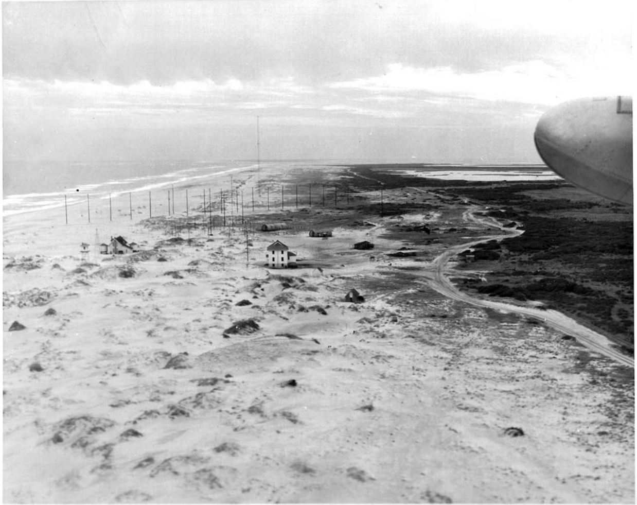
H.13 Aerial view of Station, September 1948, from the north. Shows LORAN system in place.
