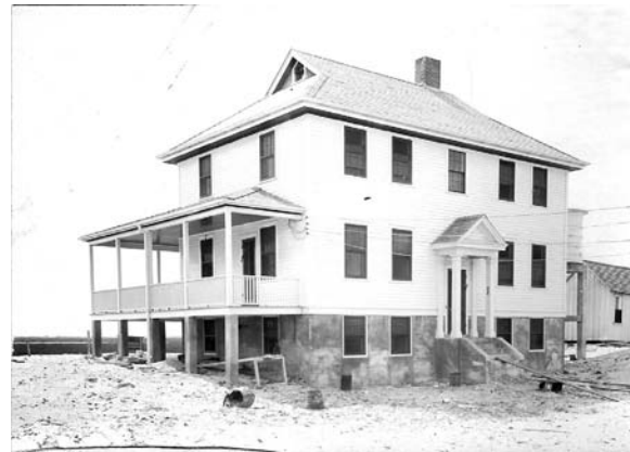
Figure B-8 1925 appearance of Bodie Island Coast Guard Station, c. 1925
