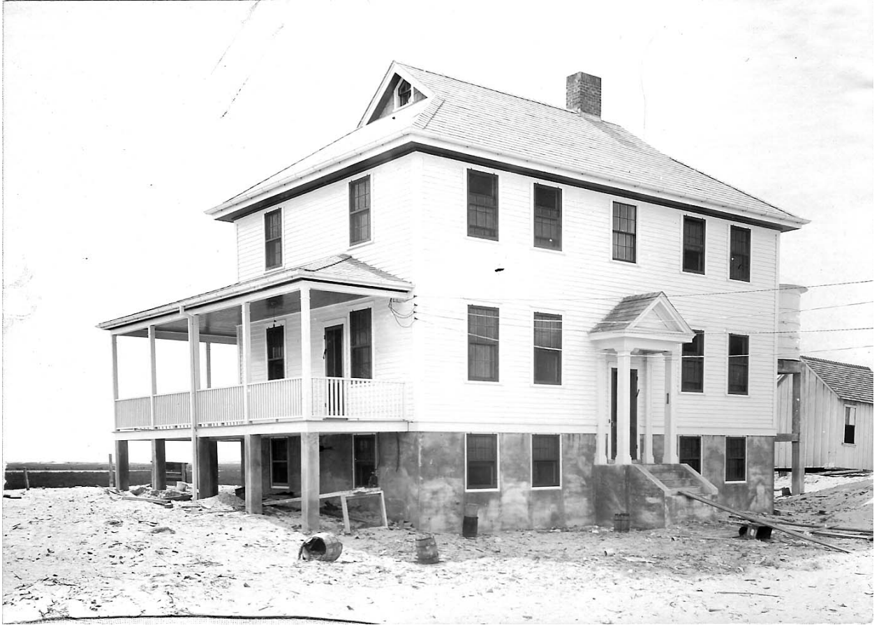
H.2 1925 Station from the southeast ca. 1928. Number 2 of 4 possible Frank L. Toon photographs. Shows station as originally constructed, east (front) and south elevations.
