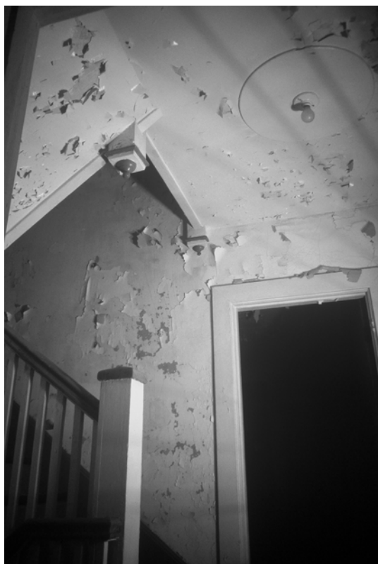
Figure C-24 Room 102 with plywood ceiling medallion and central light, staircase newel, balustrade, handrail, and pendants
