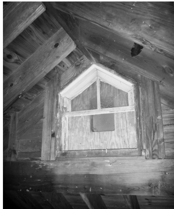
Figure C-39 Window in attic gable
