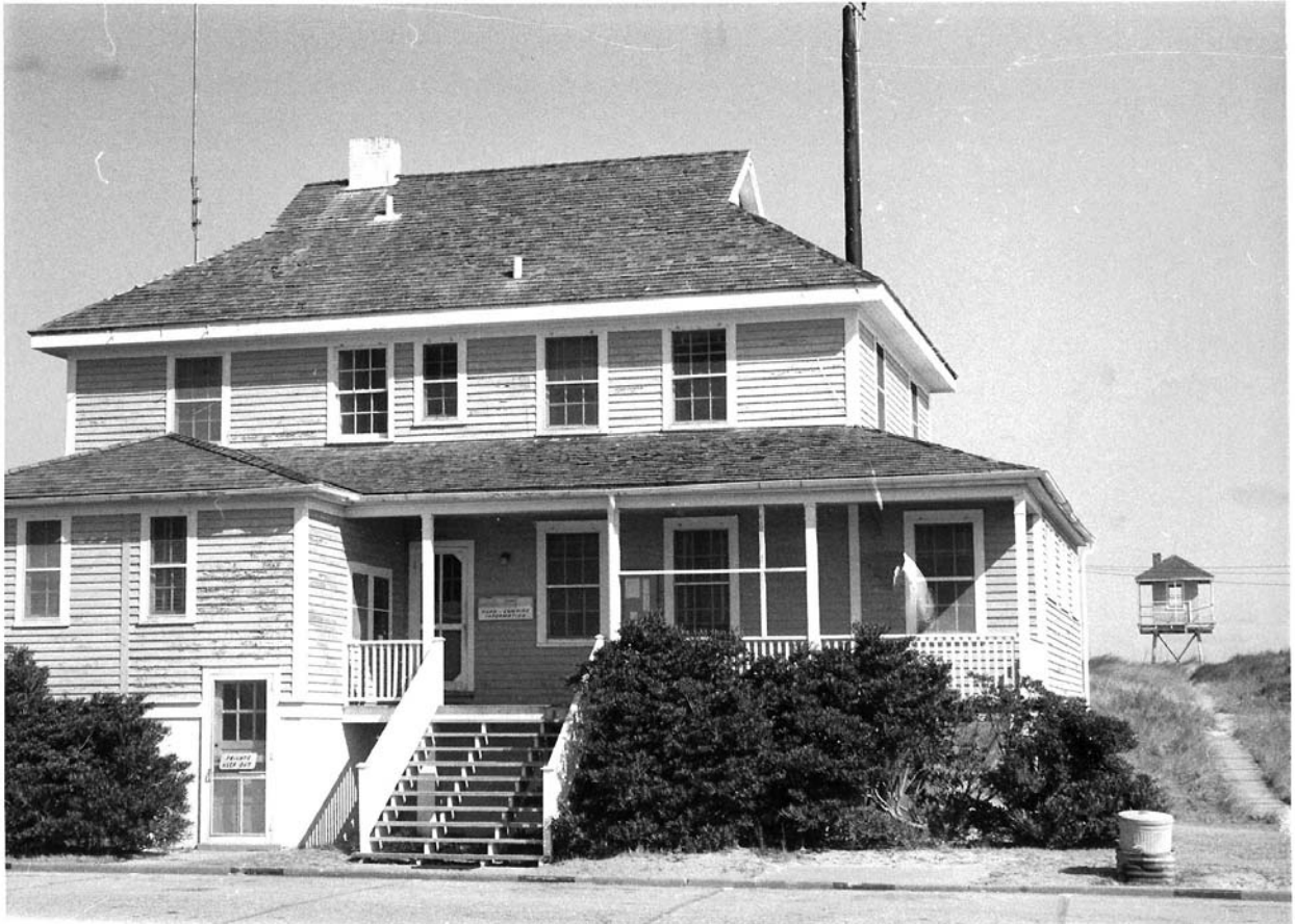
H.25 1925 Station from the southwest, ca. 1971. Label: “HS-1A Bodie Island Life Saving Service/Coast Guard Station Cape Hatteras National Seashore, Bodie Island, North Carolina.” Shows two windows on south wall of old stair tower, and door adjacent in west wall of station where a window was once located. The lookout tower is visible to the right.
