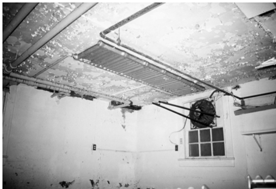
Figure C-12 Exhaust fan replaces top sash
