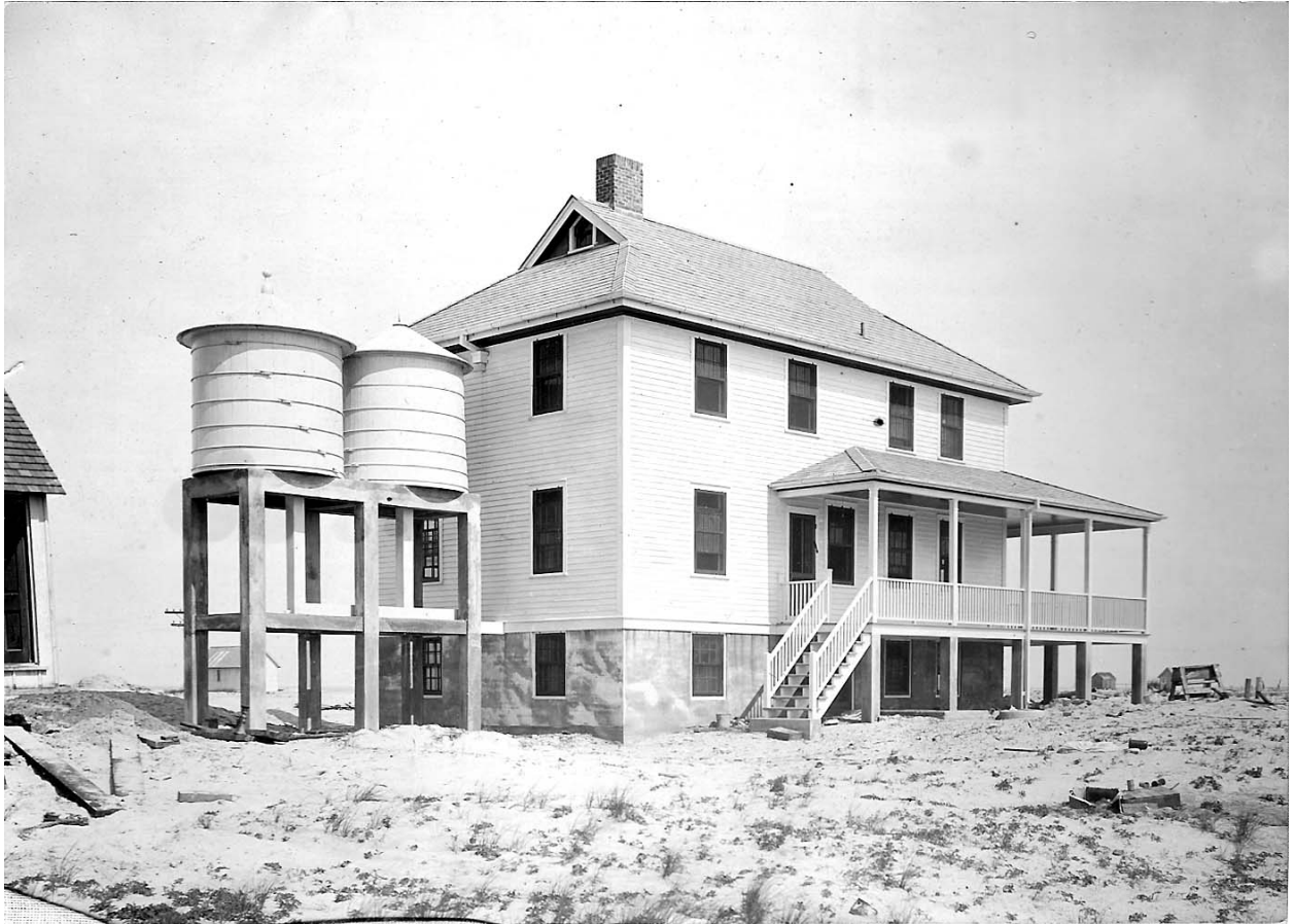
H.4 1925 Station from the northwest ca. 1928. Number 4 of 4 possible Frank L. Toon photographs. Shows station as originally constructed, north and west elevations with water storage tanks.
