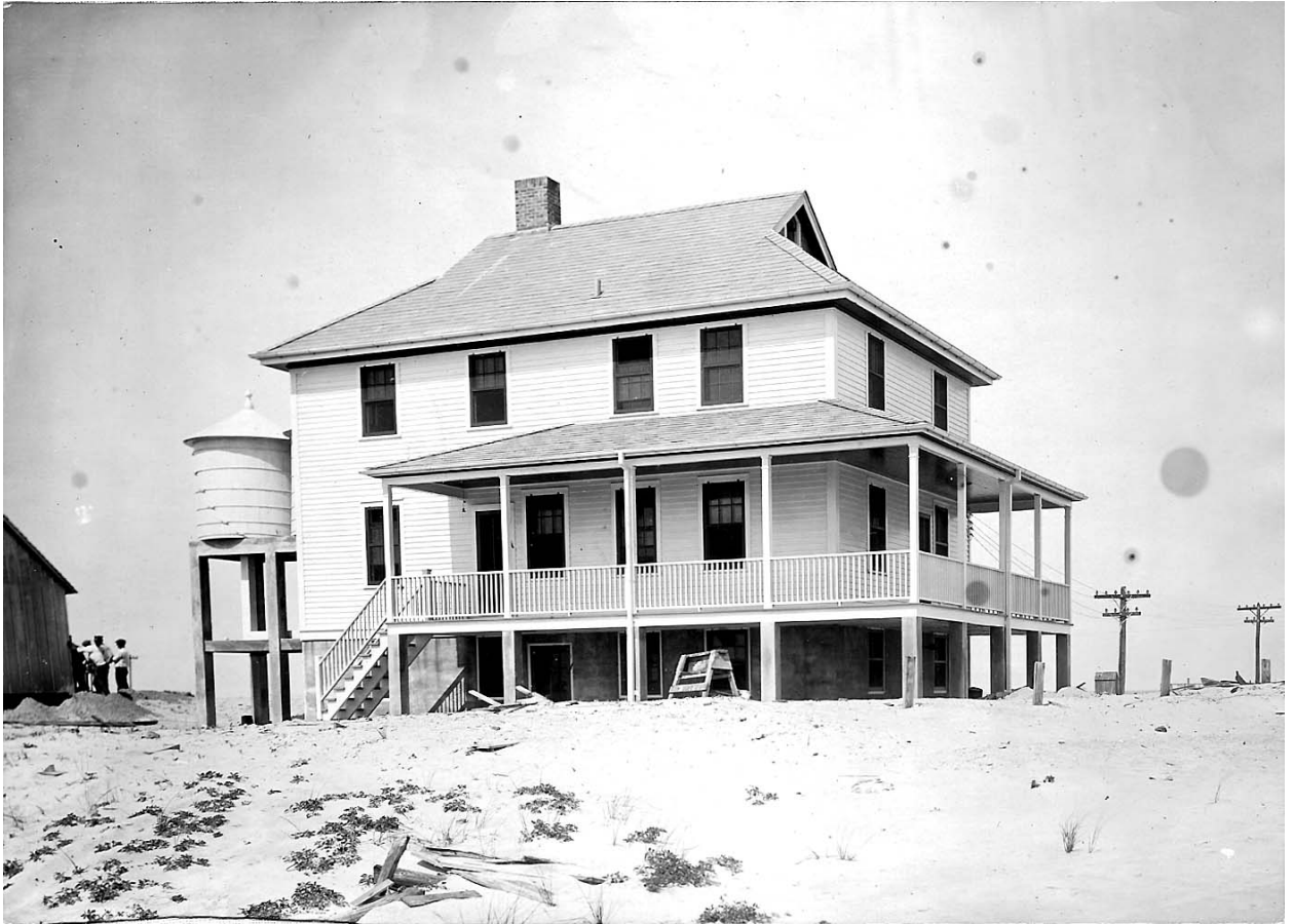
H.3 1925 Station from the southwest ca. 1928. Number 3 of 4 possible Frank L. Toon photographs. Shows station as originally constructed, west and south elevations with wraparound porch and basement entrance on west façade.
