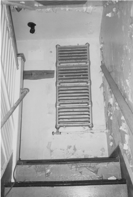
Figure C-14 Landing between first floor and basement
