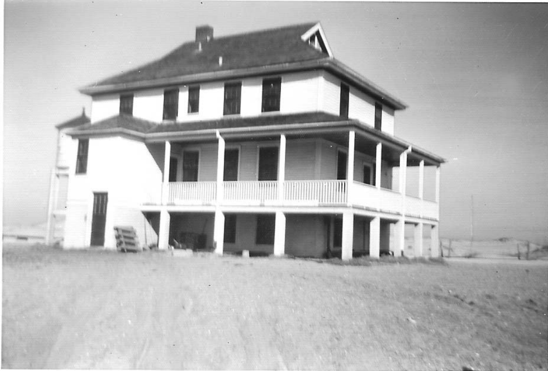
H.11 1925 Station from the southwest, ca. 1946. Label: "The barracks from the west side. 1946-47 photo by Charles D. Potts, 13 Alton Ct. Newark DE. 19711 Donated to CAHA 8/73. Former U.S. Coast Guard Stn. now NPS Ranger Stn. Bodie Island." Shows 1933 stair tower and added window into bathroom on second floor.
