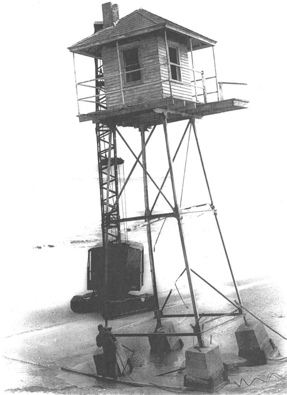
H.26 Crane in a failed attempt to save the 1925 Lookout Tower, Feb. 6, 1978.
