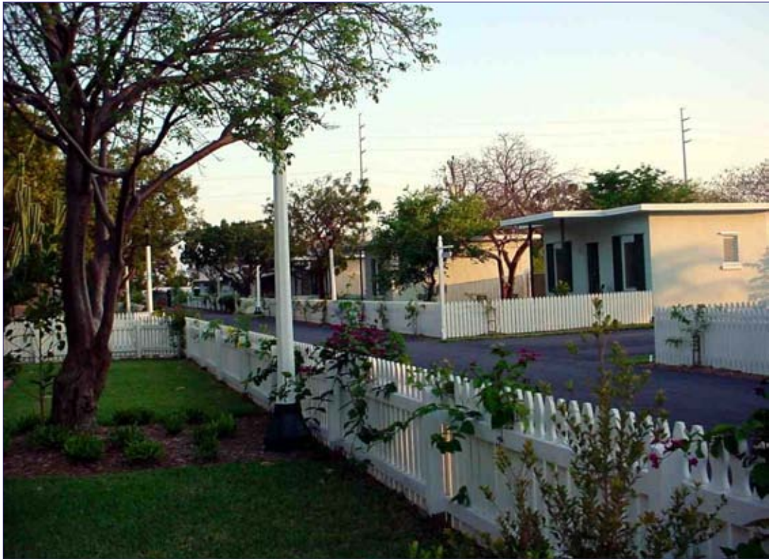
Overseas Village is an affordable housing redevelopment project resulting from a public/private partnership. Photo: Debbie Love
