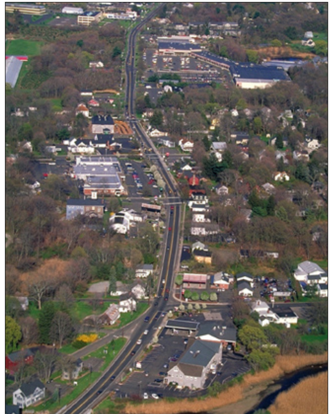
The town of Guilford, Connecticut wanted to control the future of development along Route 1, which ran through the middle of town. Source: Alex MacLean, Landslides
