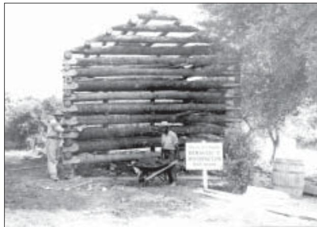
Figure 5.14. Construction of the cabin replica. Note the sign that identifies this as the location where Washington was born. 1949. BOWA files.
