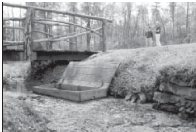
Figure 7.16. Spring box, located south of the Burroughs foundation. 2001. OCLP.
