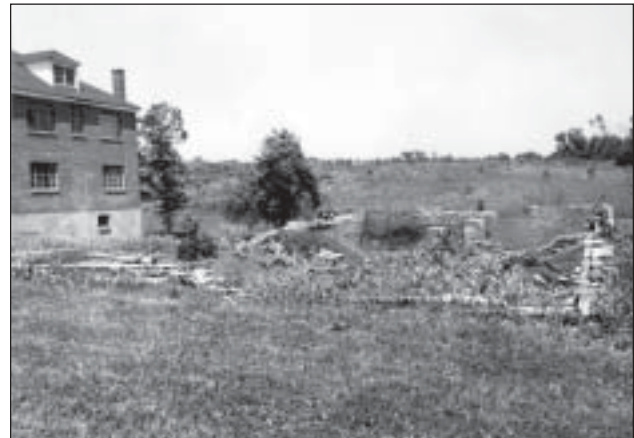
Figure 6.2. The remnants of Burch Hall. Construction never progressed beyond the foundation, which was left to deteriorate. Circa 1958. BOWA files.
