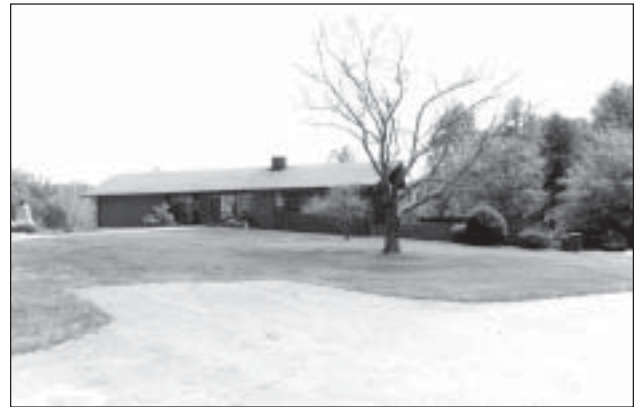
Figure 7.13. Visitor center. 2001. Photo courtesy of NPS, Stephen Clark. Cultural Resources Center/Building Conservation Branch.
