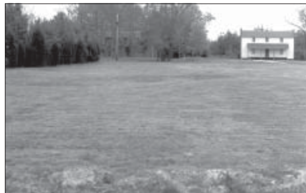
Figure 8.5. At Historic Stagville's Horton Grove, recent pine growth (left) obscures the view from Jock Road towards the five slave/tenant houses until one approaches the driveway (out of frame, right). Only one (painted white) is clearly visible here. 2001. Photo courtesy of Phillip Troutman.
