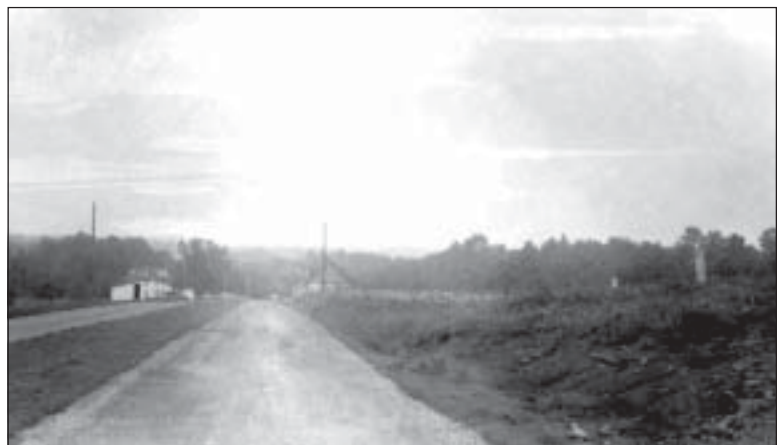
Figure 5.5. The completed double-lane boulevard style driveway. Note the graded roadbed and shoulder. The Burroughs family cemetery is visible at image right. Circa 1946. BOWA files.
