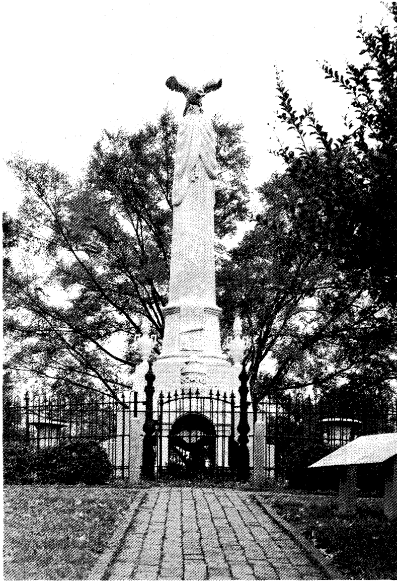
Figure 11. Monument Area, c. 1970.
