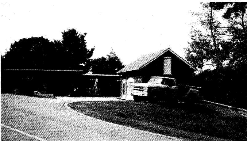
Figure 10. Maintenance additions to Stable/Utilityarea, 1991.
