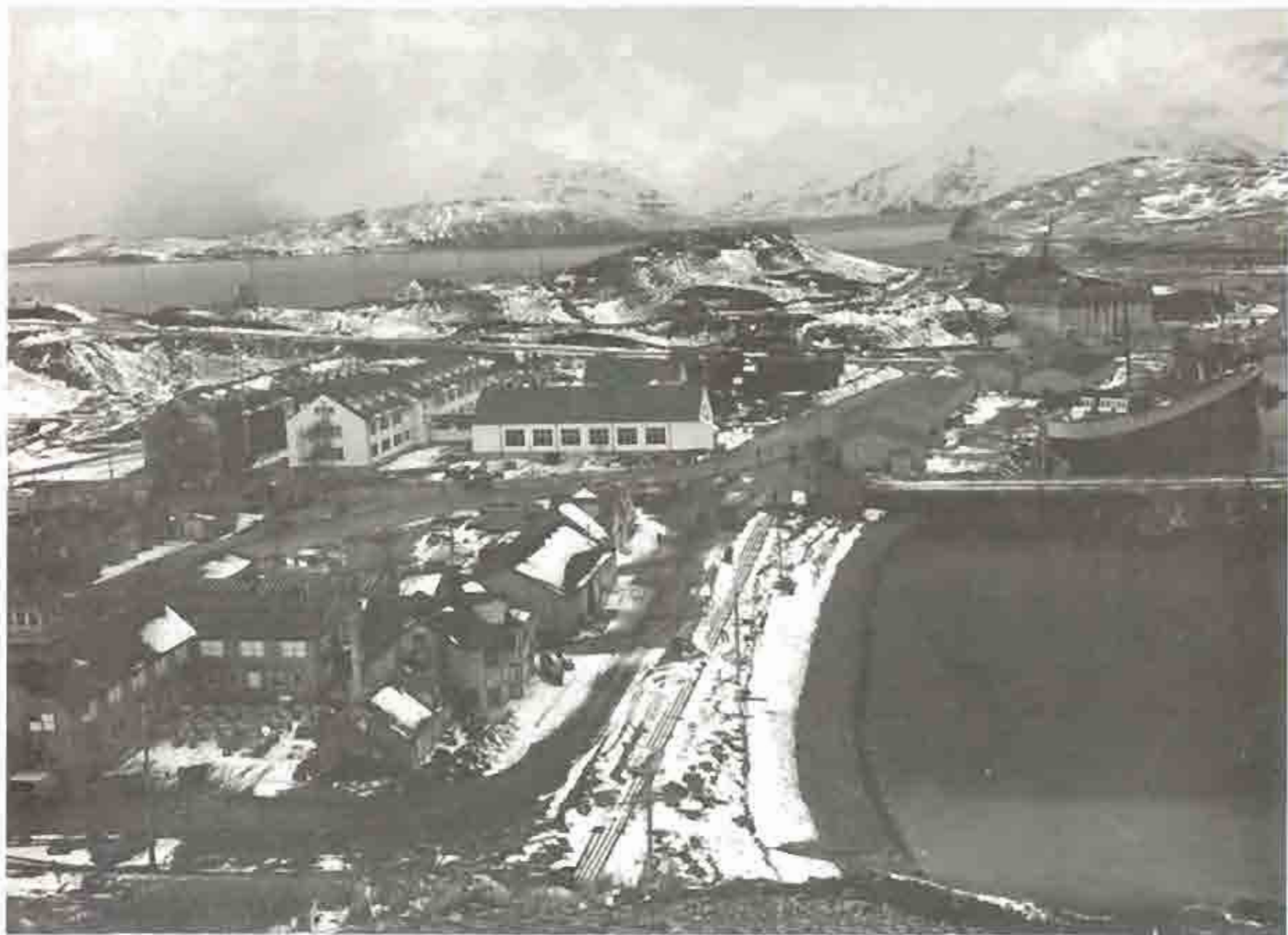
Headquarters Area, Dutch Harbor, 23 March 1942. Powerhouse and airfield under construction beyond USS Northwestern at dock.
