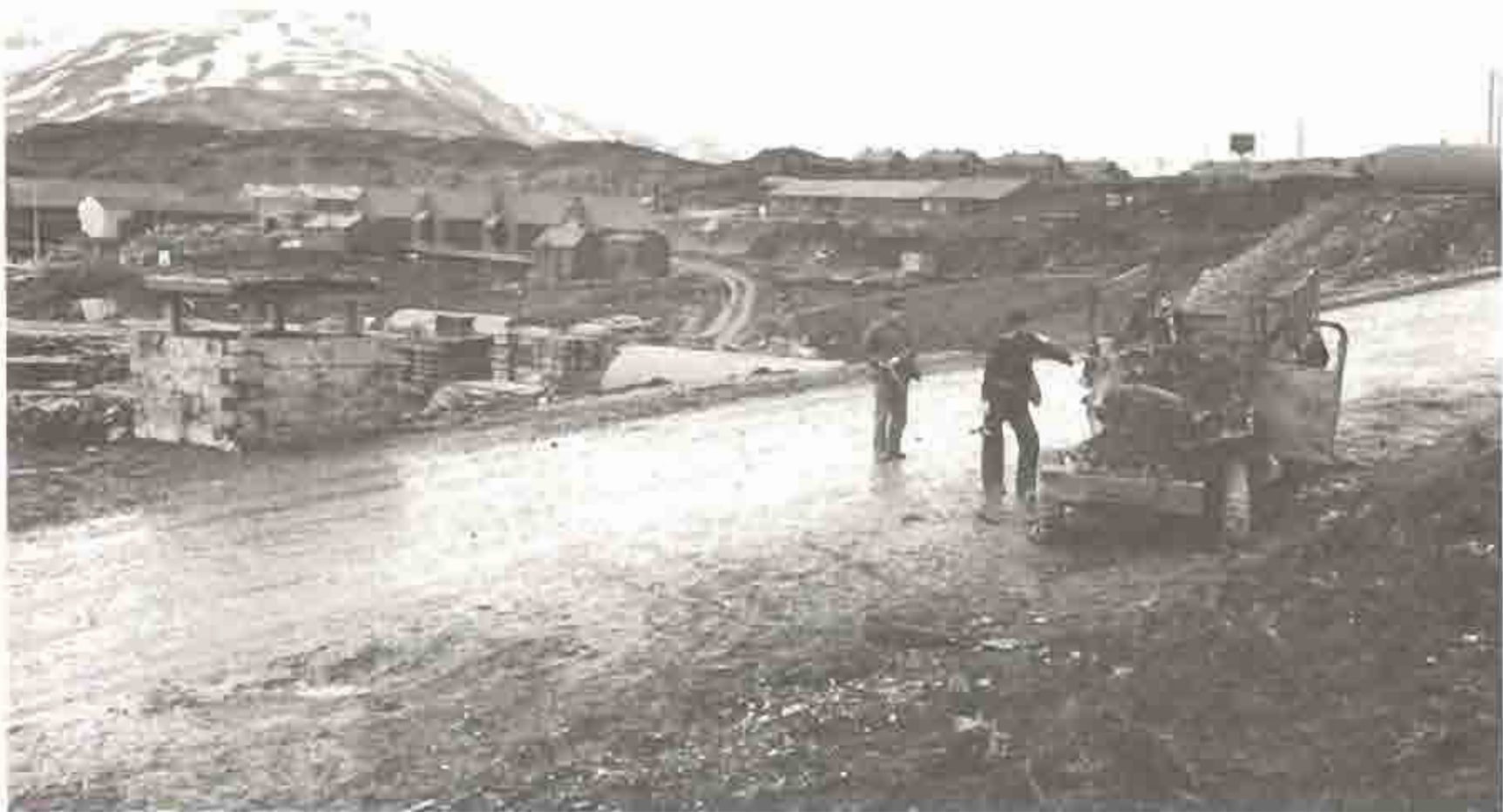
Bomb damage at Dutch Harbor.
