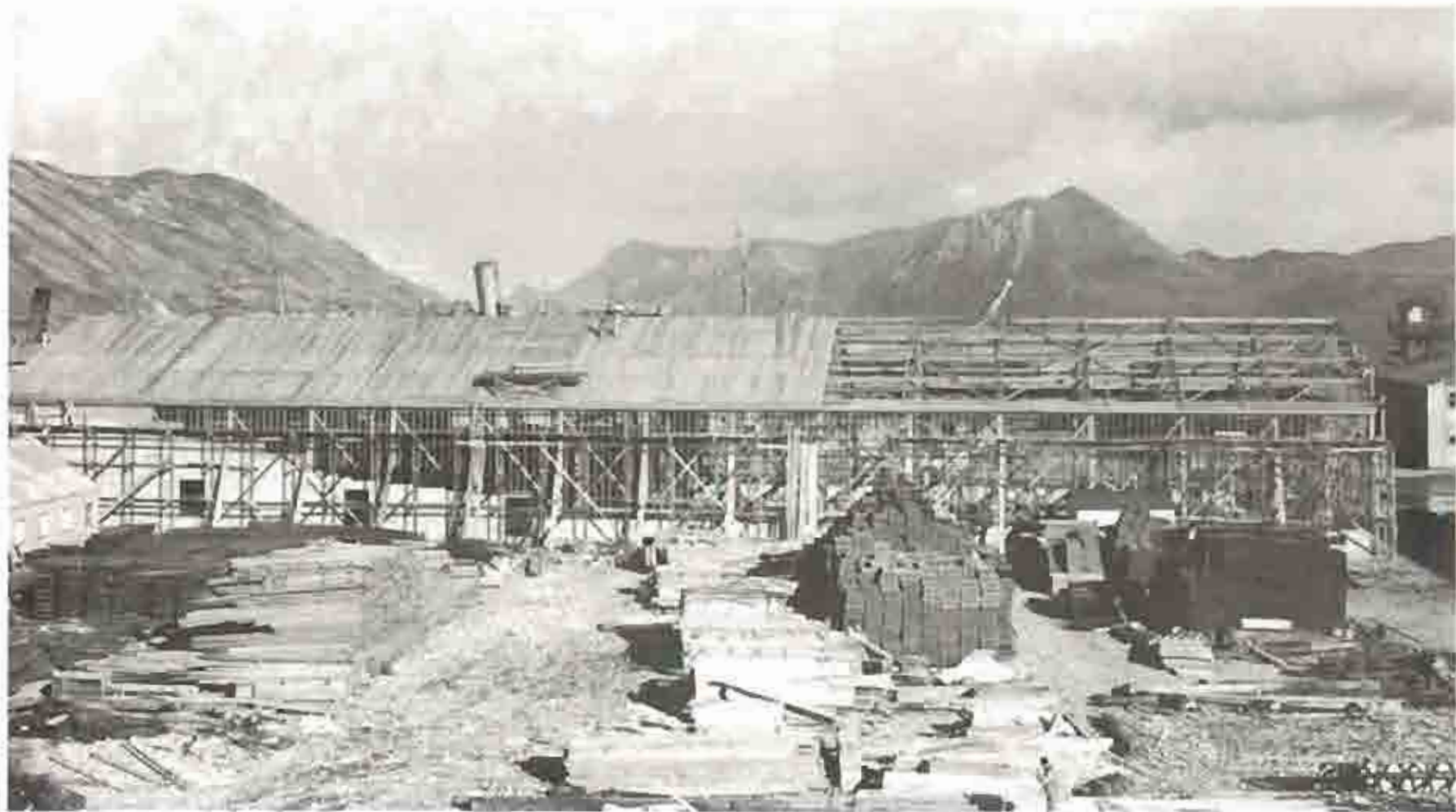
New recreation hall under construction, 30 October 1942.
