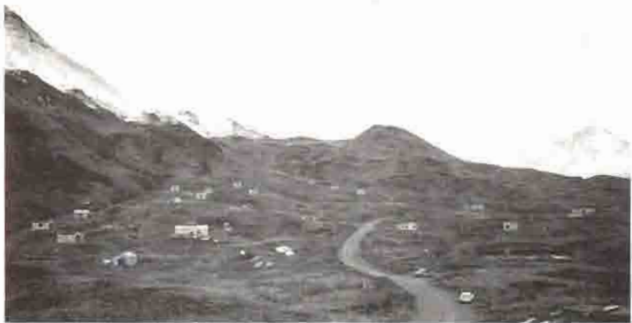
Pyramid Valley, Cabanas - Demolished.
