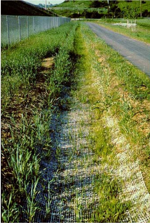
5-14 A biodegradable netting will prevent erosion until vegetation is established.
