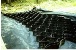
↑ Geocell ready for fill ↑
