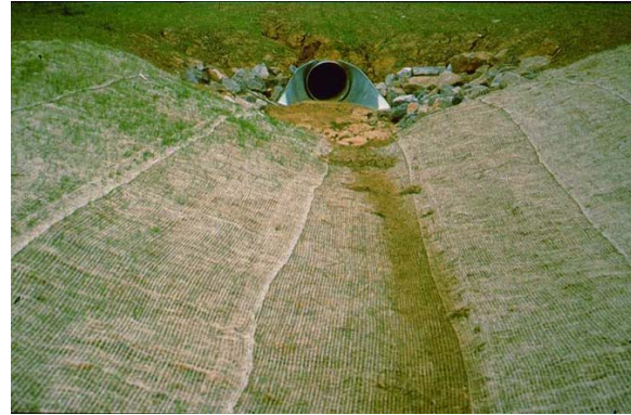
5-16 Good netting installation, but problems at pipe outlet need to be addressed.
