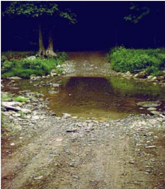
7-37 Stream fords cause erosion and sediment, degrading stream habitats. A perforated geoweb offers a stabilizing solution with proper hydraulic and stream ecology protection.
