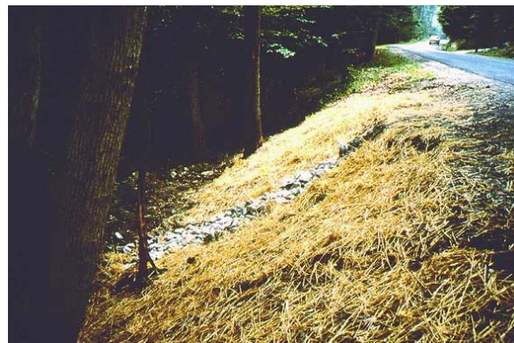
5-38 Using rip-rap for erosion prevention at culvert outlet.
