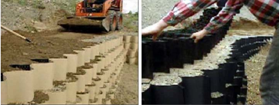
7-34 Geoweb retaining wall installations (Photos: WebTec, Inc. - TerraCell®)
