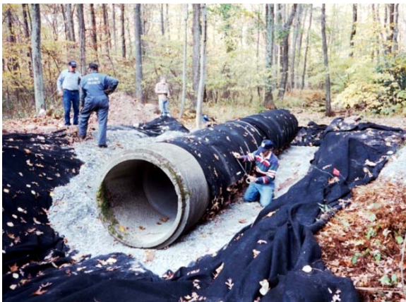
A7-06 Fabric wrap covers pipe joints, prevents fine material from entering.
