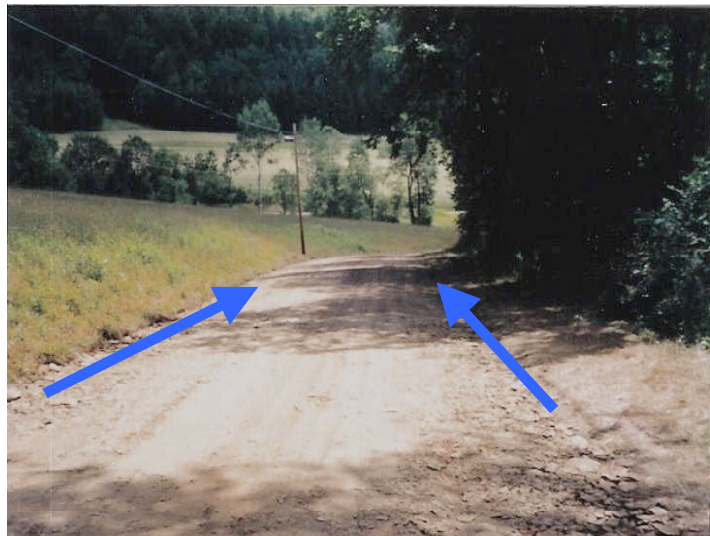
Before: The entrenched road trapped road drainage resulting in fast-moving concentrated ditchflow. This water eroded road material and deposited it directly into Pine Creek.
