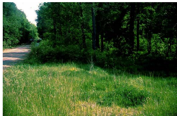
6-16 Grasses make good roadside plants, establishing surface erosion protection
