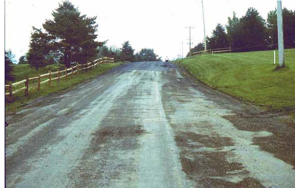
7-13 A mish-mash of road surface materials lends itself to a full-depth reclamation project.
