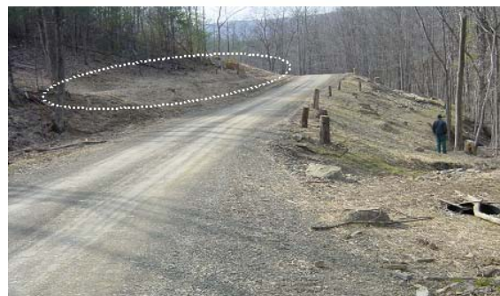
6-31 Newly constructed low-gradient bank benches.
