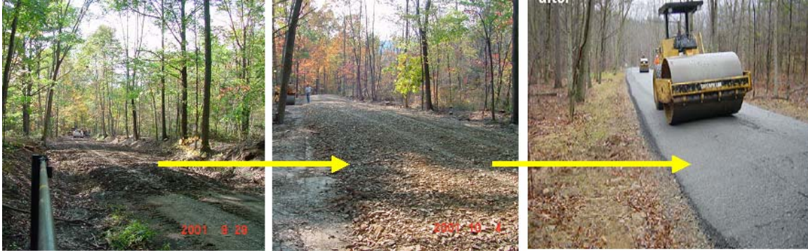
ESMP12-02 Raising the entrenched road—step-by-step.
