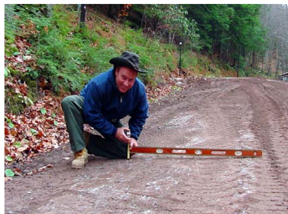
3-20 Checking Cross Slope to insure proper drainage.
