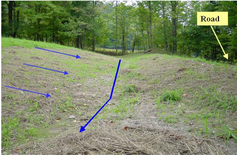
6-28 Diversion Swale: Wider swales and gradual slopes result in more infiltration and less water volume to handle.
