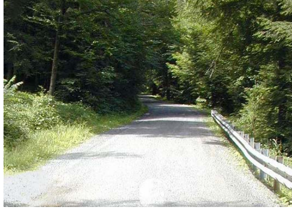
6-10 Pockets of deep shade can create irregular winter icing conditions.
