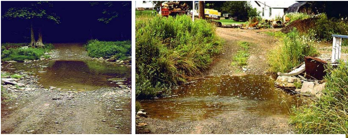
5-33 Existing fords should be stabilized to prevent erosion and stream degradation.
