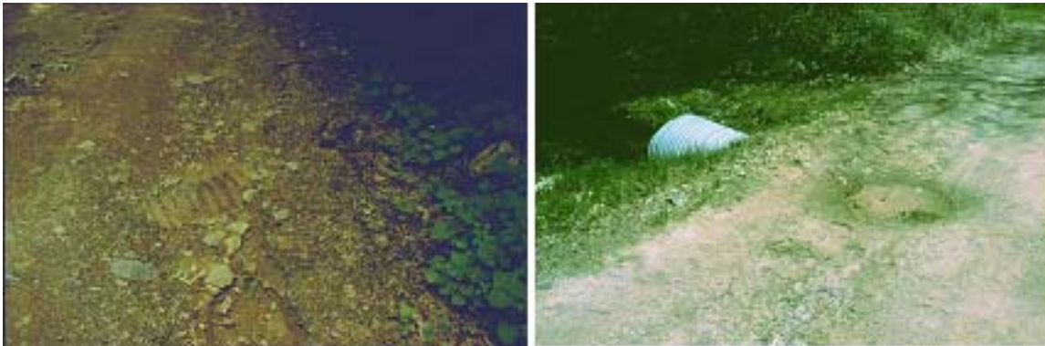
5-30 Shallow pipe installations can cause continual road deterioration.
