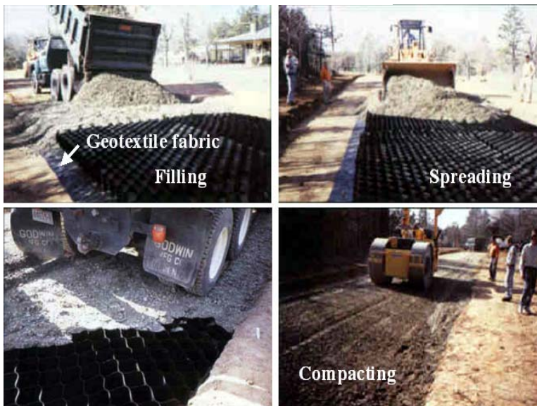
7-33 Geocells for road base stabilization. (Photos: WebTec, Inc. - TerraCell®)
