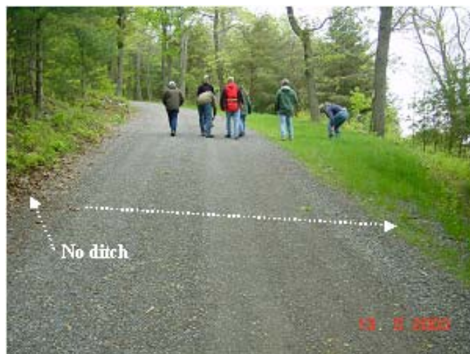
5-09 Outsloping this road proved beneficial, eliminating ditches and cross pipes.
