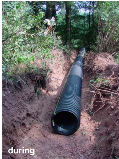
Pipes Through the Bank. Note the depth of the trench during construction. After construction the pipe has been covered and stabilized with vegetation.
