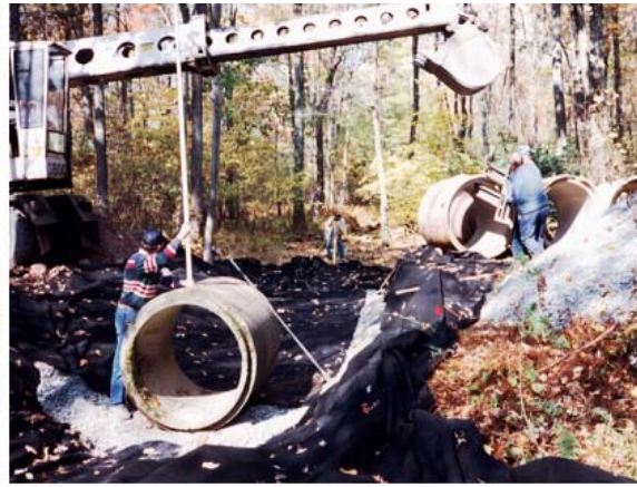
A7-05 New line and grade checked
