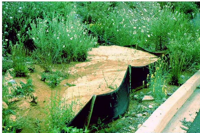
5-07 Cleaning is required when sediment reaches one-half the height of the fence.
