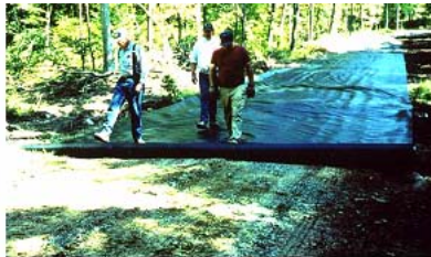
↑ Rolling out the fabric ↑
