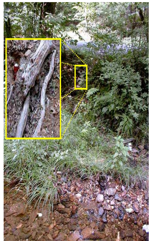
5-39 Brush, tree stumps, etc. can be effective energy dissipaters.
