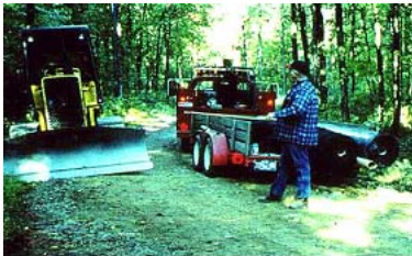
↑ Rolls of fabric waiting for installation ↑
