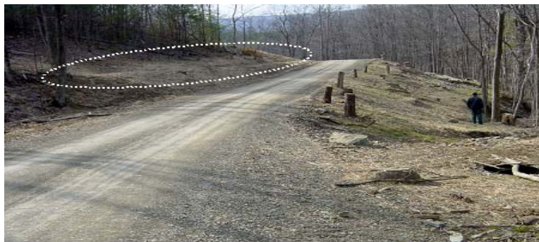
ESMP#13-04 Newly constructed low-gradient bank bench.
