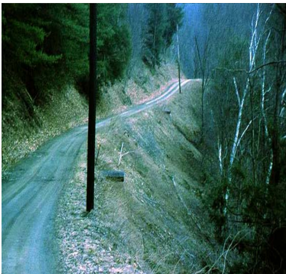
5-24 Grade breaks result in short road sections with reduced water volume and flow velocity.
