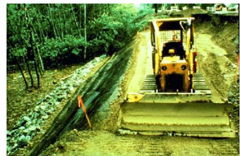
7-27 Construction of a geogrid reinforced embankment.
