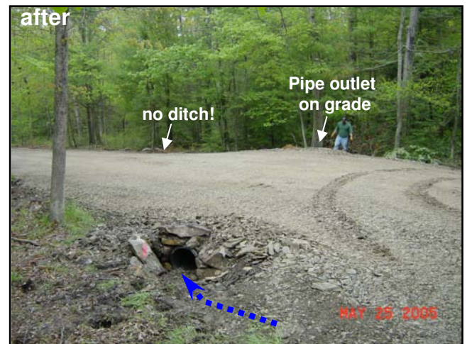
Photo 5. One of two new crosspipes installed. Notice the grade-break in the road over the pipe to get water off the road.
