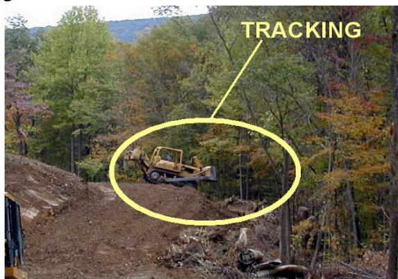
ESMP#13-03 Tracking newly constructed banks.
