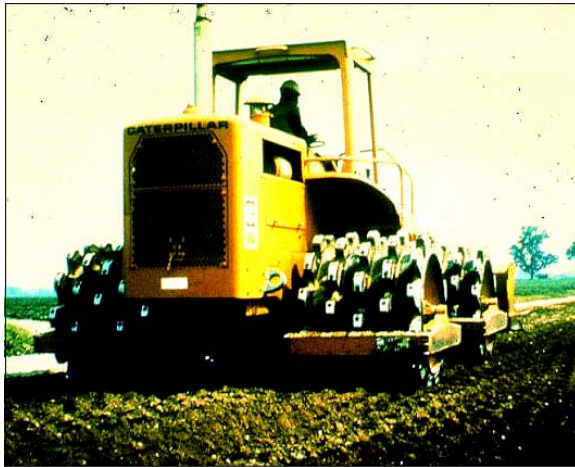
7-14 A sheep's foot roller is used for soil compaction.
