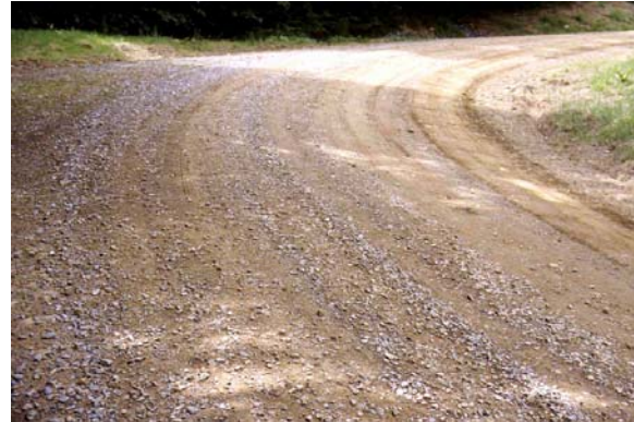
3-09 Banked (superelevated) curve.
