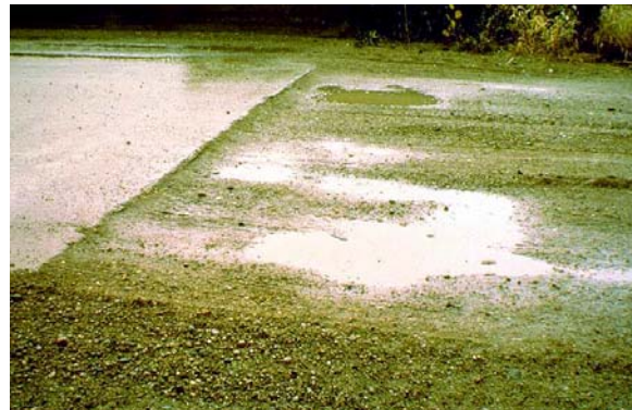
3-26 Bridge approach areas demand special attention and usually more maintenance.
