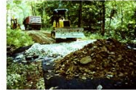
↑ Raising road elevation ↑
