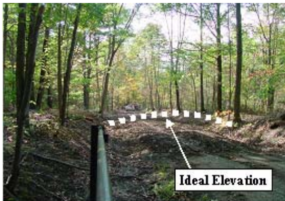
After finishing the shale
