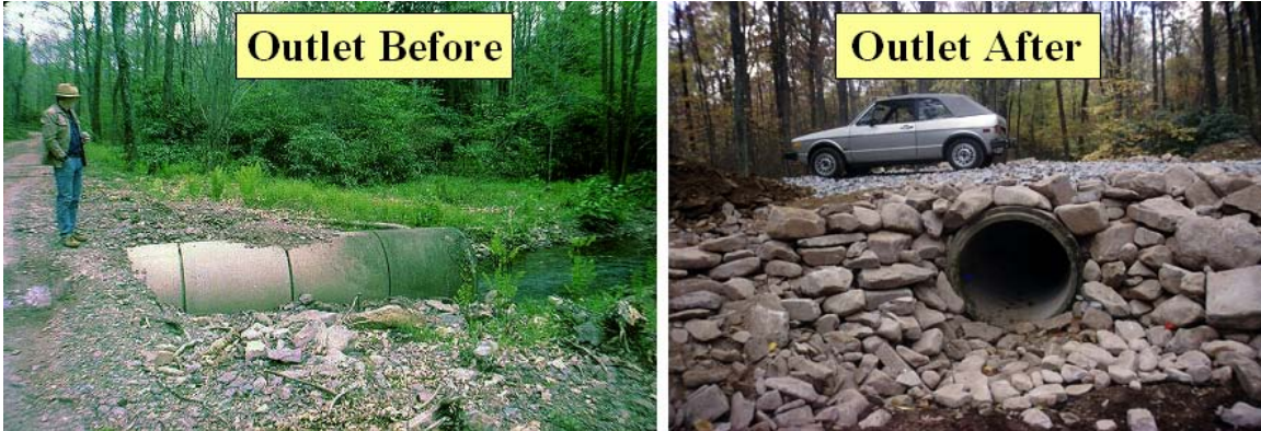
A7-11 Outlet conditions before and after the project.
