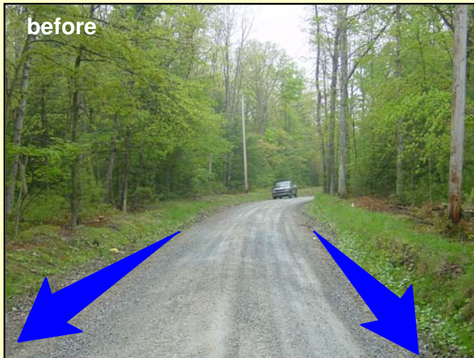
Photo 3. The entrenched road traps water in the road area and conveys it down to the stream. Note the elevation of the road relative to the utility pole on the right compared to Photo 4 .
