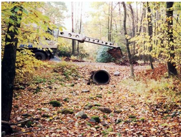
A7-02 Excavation of existing pipe during dry conditions.
