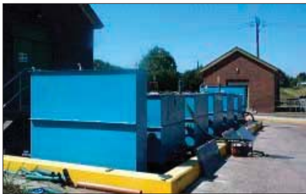
ABR installation. Photo courtesy of Atkins Water, 2006.
