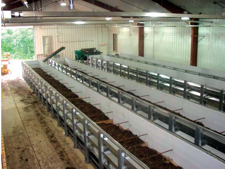
Granville Township, PA vermicomposting facility (Photo courtesy of Granville Township)
