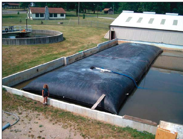
Geotube® Container at Cambridge WWTP after being filled with 250,000 gallons of biosolids. (Mastin and Lebster, 2006).
