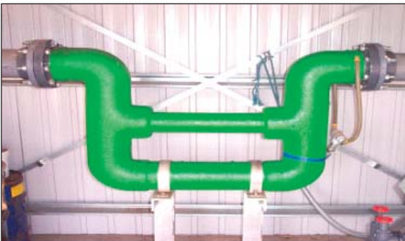
Rapid Flocculation Mixer
