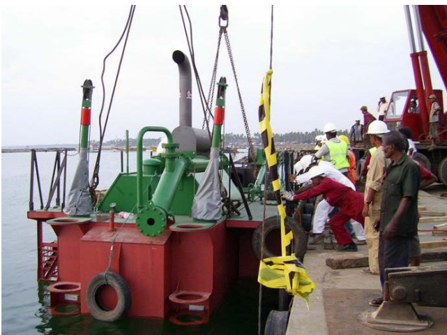
The dredger is launched at Hikkaduwa Harbor.
