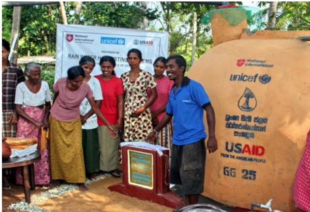
New rainwater harvesting systems for tsunami-affected families in Hikkaduwa, Sri Lanka are the first of 680 such systems to be constructed in partnership with UNICEF and local communities.
