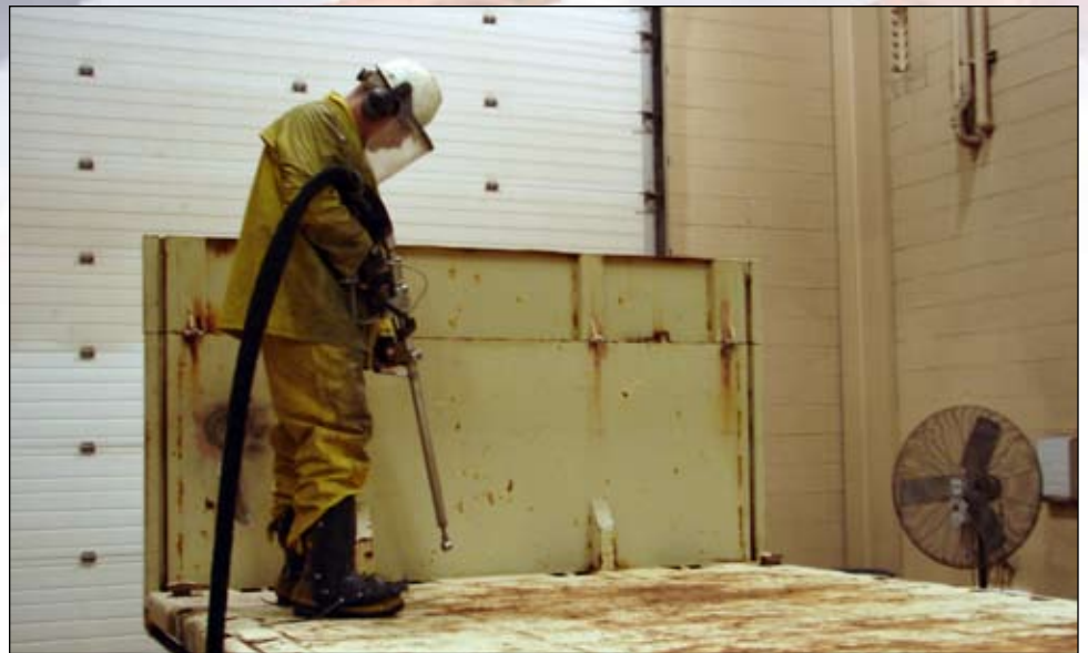
A painter uses claws equipment to strip paint from a MIARNG vehicle. The system recycles the water used for paint stripping through a filtration system. The substitution to water-based paint processes has also benefited soldier health and safety by minimizing their exposure to potentially harmful toxins.
