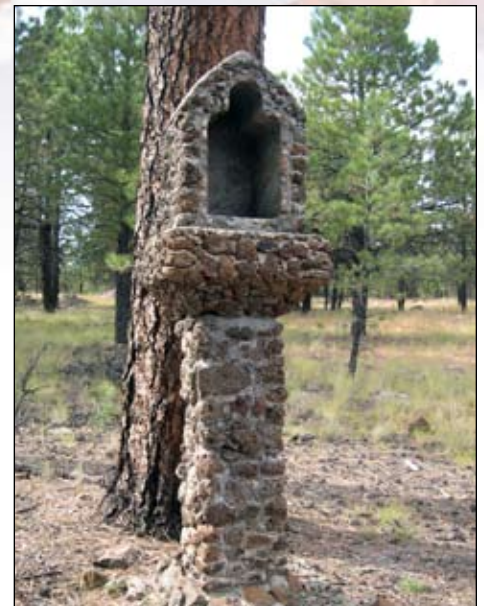
This 2007 photo depicts a hand-made shrine (statue niche) built by Austrian WWII POWs at Camp Navajo. The shrine was constructed of fist-sized and larger chunks of volcanic rock held together with a concrete mortar. The style, shape and size of construction is based up on the POW's mental template of a proper shrine and is reminiscent of staupe niches found throughout Austria along trails and pathways. (Photo by Dorenda Coleman, AZ ARNG Environmental Staff)
