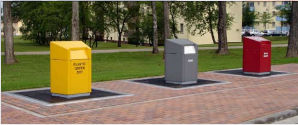
A modern underground recycling set for glass, cans and plastic. Only the inlets are visible. The containers are in the ground and can be lifted by the truck.
