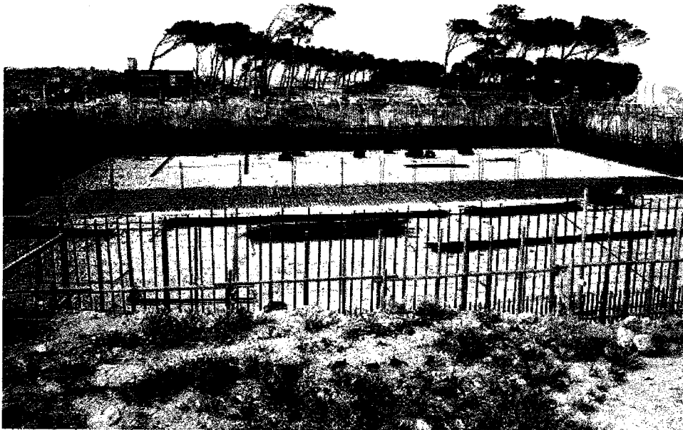
Construction of a 10,000 cubic meter water storage reservoir in Bethlehem. (May 1998)
