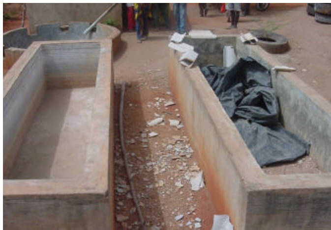
Photograph of empty tile-curing basins at ADF's Brick and Tile project in Benin. The economic analysis predicted that there would be times when the project would not be able to produce at full capacity because the curing basins would be full.
