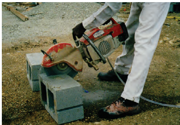
When applying water to the blade, exposures of handheld saw operators to silica are considerably reduced. (Photo courtesy of OSHA.)
