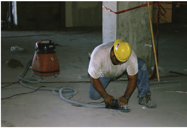
Grinder with attached VDC system. (Photo courtesy of OSHA Directorate of Construction.)
