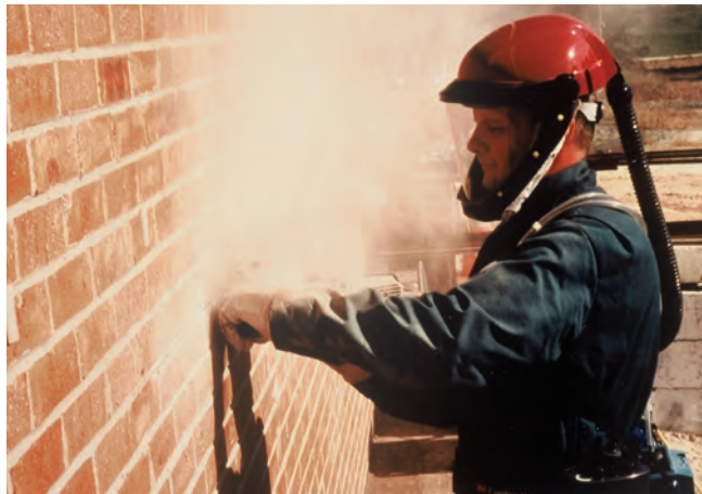
Grinders who perform tuckpointing without dust controls are frequently exposed to extremely high silica levels. (Photo courtesy of CPWR.)
