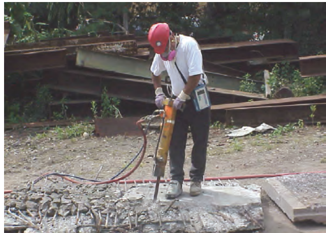
Employee chipping concrete with a jackhammer while using a wet method. (Photo courtesy of NIOSH.)
