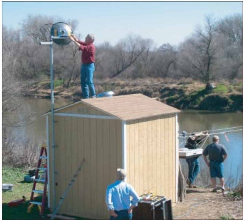
Fig. 3. Pulsed Doppler radar on the bank of the San Joaquin River, California, provides surface-velocity measurements. Cable across channel is used to suspend GPR system over the water to measure channel cross section.
