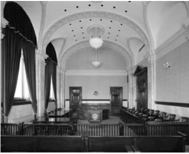
FIGURES 19-20 Limit recessed lighting to the ceiling perimeter to avoid overpowering historic chandeliers and changing the character of historic ceilings.
