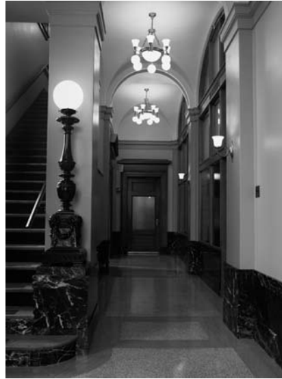
FIGURE 3 Interior upgrade projects often provide opportunities to restore compromised spaces and make a historic building more marketable.
