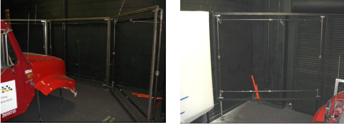
Figure B.7: Front screens frame structure and support
