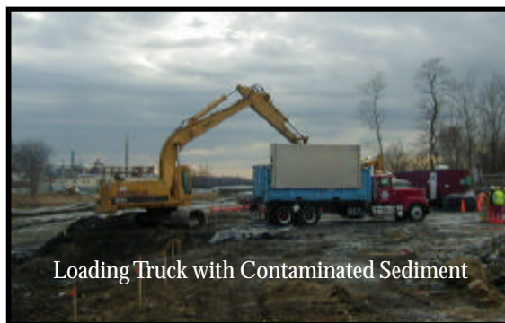
Removing Contaminated Sediment North of Wood / Slocum Street
