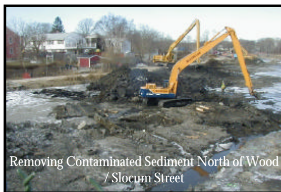
Acushnet River North of Wood / Slocum Street
