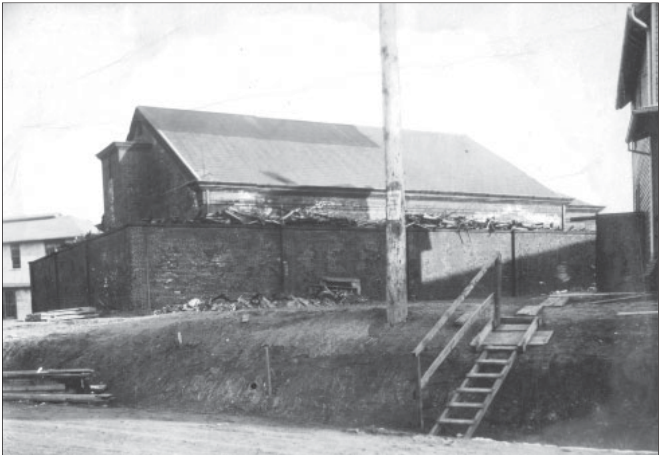
Figure 4.29. Photograph of southwest portion of Fort McHenry c. 1924. The handbill posted on the utility pole reads, "Labor Will Win the War." Note accumulation of refuse within outer Magazine perimeter wall. Fort McHenry Library Special Collections, FOMC 5468.
