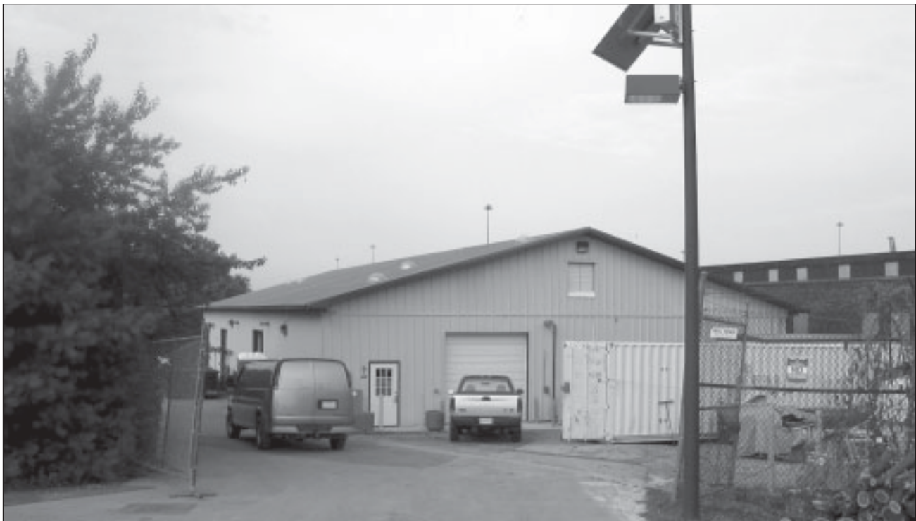
Figure 6.4 Inside the Fort Avenue gate, south of the entrance road, an additional park maintenance compound has been developed, using a salvaged metal building obtained from Gettysburg NMP. OCLP, July 2003.
