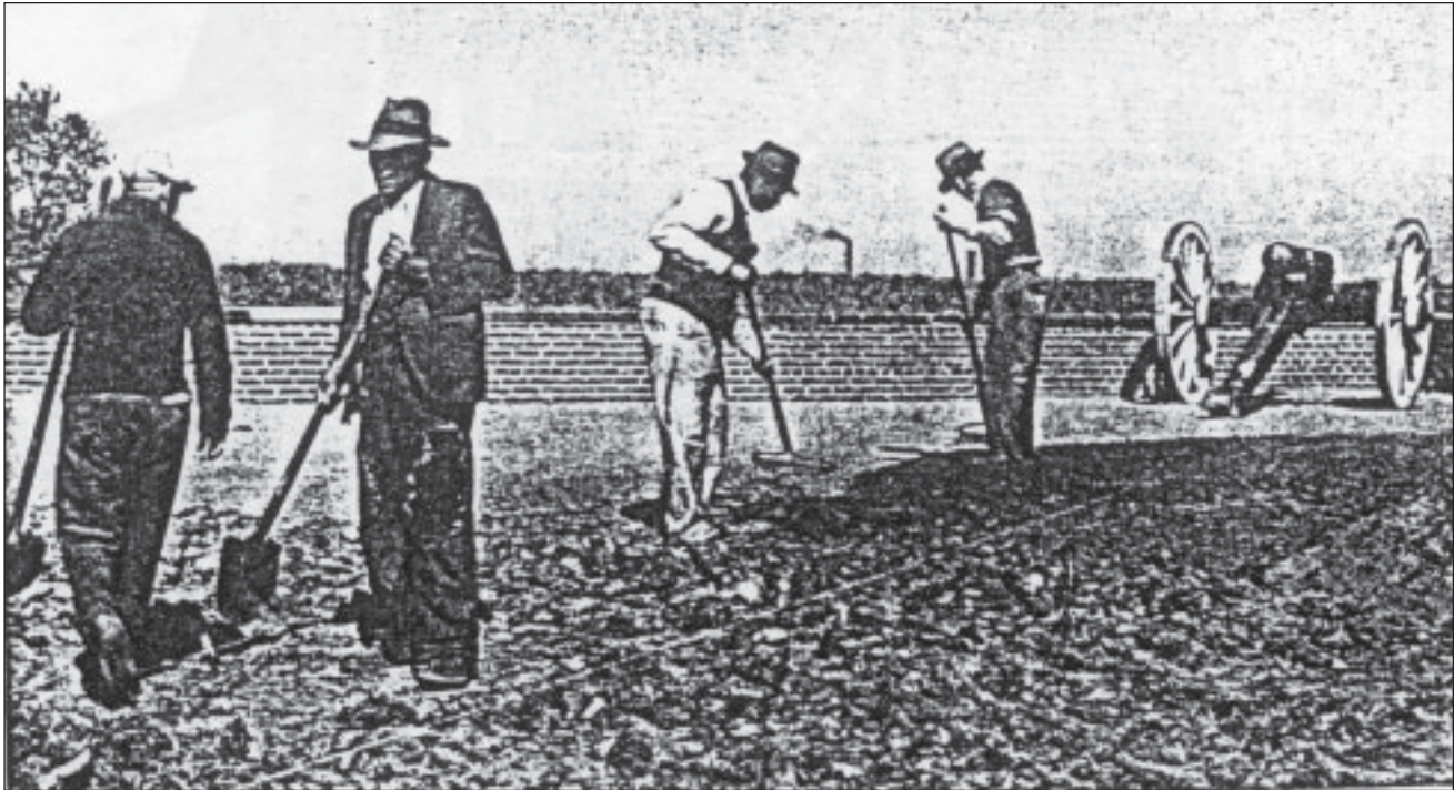
Figure 5.5. Most of the relief labor directed to Fort McHenry as part of President Roosevelt’s “New Deal” was concentrated at the historic Star Fort and areas east of the 1814 reservation boundary. Work performed was predominantly unskilled or semi-skilled, such as grading, painting, pointing mortar joints in brick walls, and assorted landscape related tasks utilizing laborers hired through local WPA agencies. Skilled trades were obtained under contract, such as the construction of public restrooms inside a historic barracks building. Superintendent’s Monthly Narrative Report for July 1938. Fort McHenry Library Special Collections.
