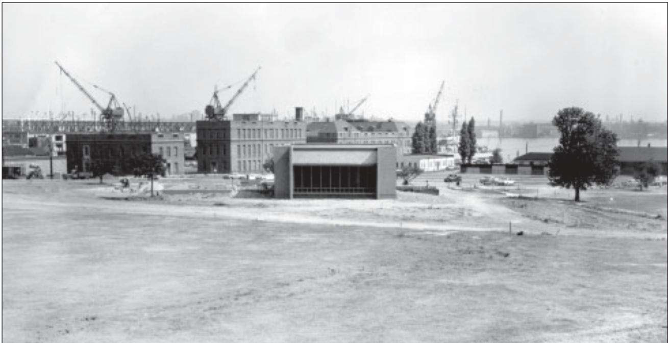
Figure 5.21. Construction progress photograph, 1963. The park's new visitor center building was designed to be inconspicuous and understated. Its north and south facades featured extensive window glazing, creating views out into the landscape. Fort McHenry Library Special Collections.
