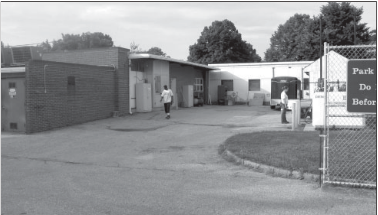
Figure 8.24 Maintenance Shop. The maintenance shop was built in 1963-64. It is located in the northwest corner of the monument grounds adjacent to the Park housing complex. Non-contributing. OCLP July 2003.
