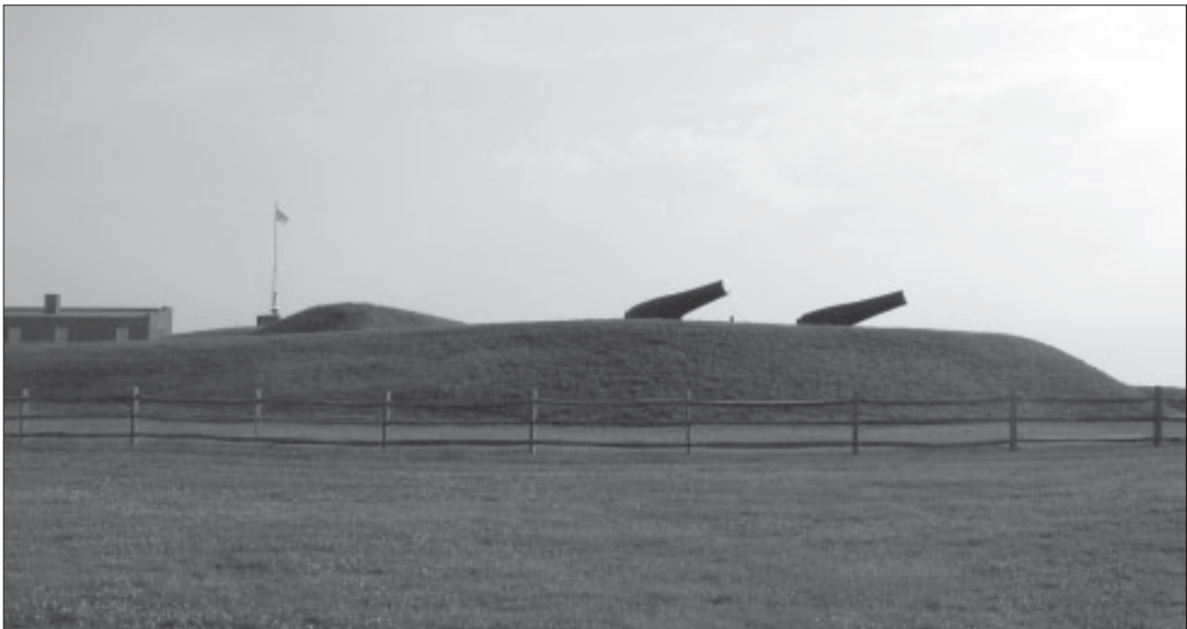
Figure 8.18 Outer Battery. Fort McHenry's Outer Battery was built between 1836 and 1837. Featuring emplacements for thirty-nine guns, its purpose was to provide a first line of defense between the fort and the Seawall. Extensive modifications were made in 1866, following the end of the Civil War. Contributing. OCLP, July 2003.
