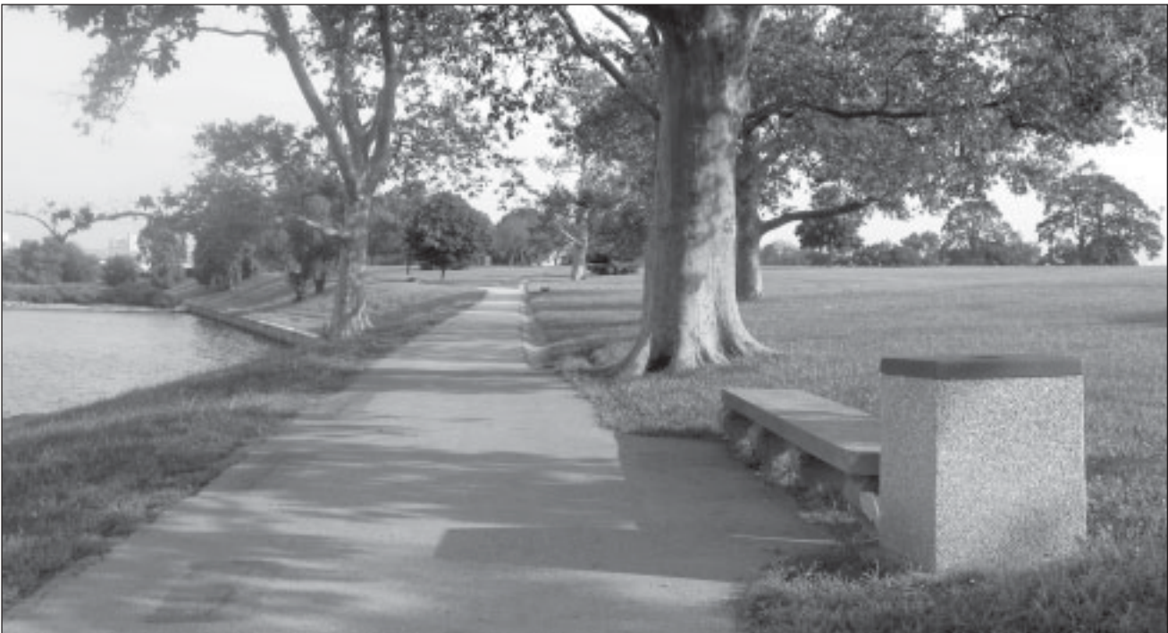
Figure 8.7 Classically Styled Concrete Benches. During the War Department's stewardship of "Fort McHenry National Park," seventeen additional benches were designed and installed on the outboard side of the Seawall Trail. These benches draw upon the design features of the earlier stone benches, yet were fabricated of inexpensive concrete. These benches have since been relocated to the inboard side of the Seawall Trail. Contributing. OCLP, July 2003.
