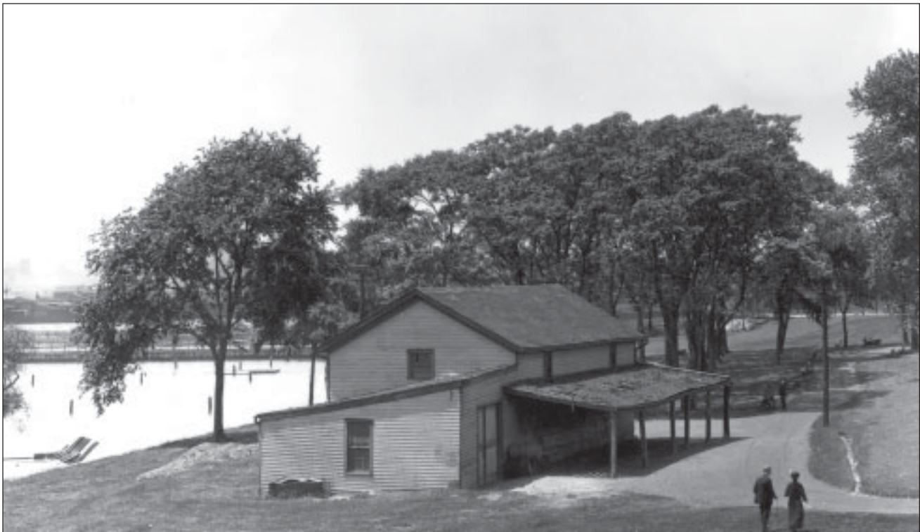
Figure 4.5. Fort McHenry c. 1914-1915. This image is paired with Figure 4.6 to the right, depicting landscape conditions southwest and west of the Star Fort. Note failing porch roof of former Quartermaster's Stables. Fort McHenry Library Special Collections, FOMC #8996M.
