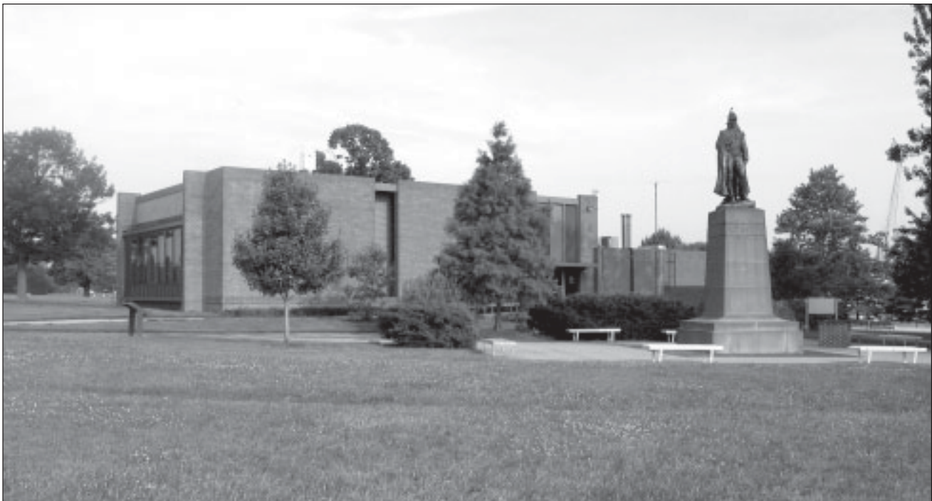
Figure 8.22 Visitor Center. The 2400 square foot visitor center was constructed in 1963-64 during the period of development in the NPS known as Mission 66. It is located approximately 300' north of the fort. It exhibits a functional contemporary design typical of late 1950s and early 1960s modern architecture. Non-contributing. OCLP, July 2003.
