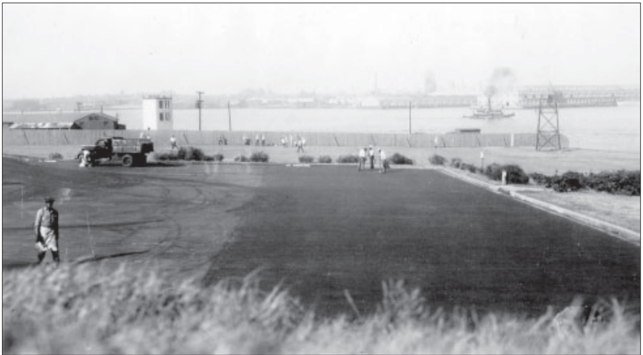
Figure 5.2. Photograph of fifty-car parking lot being resealed c. 1934. Note board fencing surrounding Dept. of Engineers parcel. Fort McHenry Library Special Collections.
