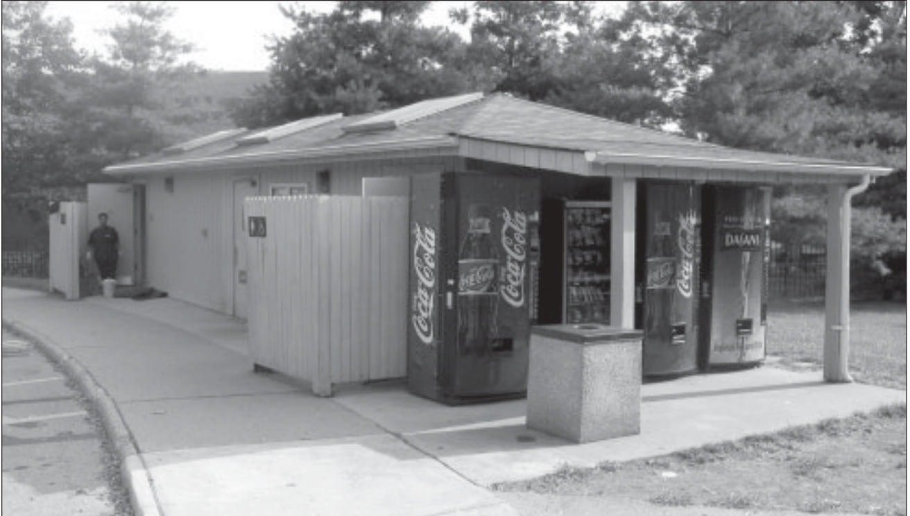
Figure 8.23 Comfort Station. This building, constructed in 1988, is located near the picnic area and tour boat dock. The one-story building measures 18' by 58'. The hipped roof building has entrances at either end with screened enclosures. Non-contributing. OCLP July 2003.
