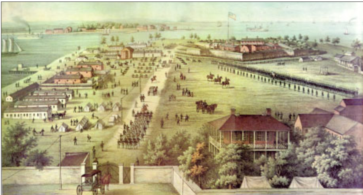
Figure 2.12. 1865 color lithograph by E. Sachse of Fort McHenry showing landscape conditions during the final months of the Civil War. Note the conversion of the three 1843 stables to house Confederate prisoners, employing the use of surrounding stockade fence and guard towers. The post cemetery and gallows is also prominently in view. Following the end of the war, the prison buildings were converted into enlisted men's barracks and remained on site until 1926. Enoch Pratt Free Library, Baltimore, MD. Cator Collection No. 166.
