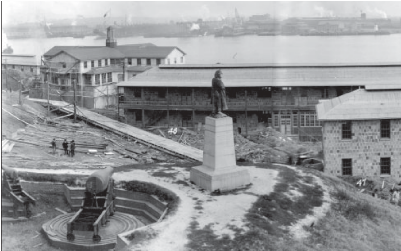
Figure 4.17. Panoramic photograph. This image is paired with Figure 4.18 to the right, depicting conditions during construction of General Hospital #2. Note absence of seat-wall exedra at Armistead statue. General Hospital #2, Fort McHenry, Balto., MD. J. Henry Miller, Inc. Contractor, 1918. Fort McHenry Library Special Collections, FOMC #2368.
