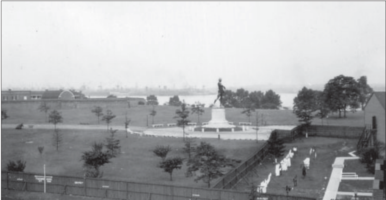
Figure 5.10. Looking southeast from Coast Guard Training Station, November 1944. Late in the war, the area north of the central driveway was occupied with a compound constructed by the Navy Department. The buildings were former CCC barracks in West Virginia, dismantled and transported to Fort McHenry. Fort McHenry Library Special Collection No. 46, U.S. Coast Guard.
