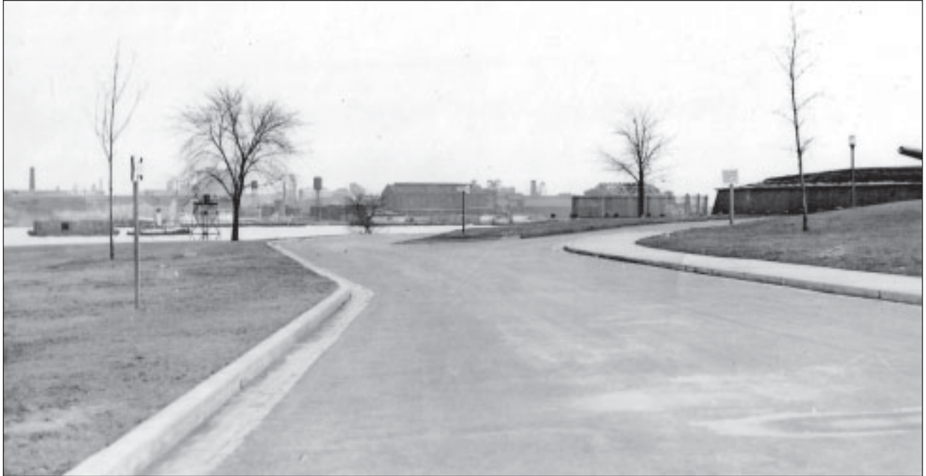
Figure 5.1. Photograph of entrance drive leading to parking lot c. 1934. Note concrete curbing with brick gutter, arrow shaped directional signage and cast iron street light fixtures. Also note Washington Elm and protective iron fencing. Fort McHenry Library Special Collections.
