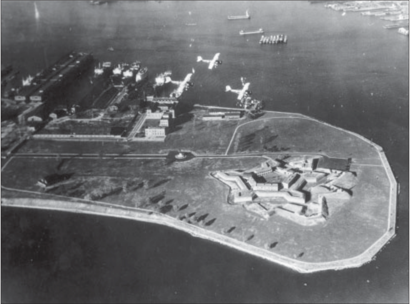
Figure 4.31. This c. 1930 oblique aerial photograph shows Fort McHenry near the completion of the U.S. Army's site restoration and park development program. The overall character of the site would remain essentially as shown here until the National Park Service MISSION-66 development program of 1962. Fort McHenry Library, Special Collections.
