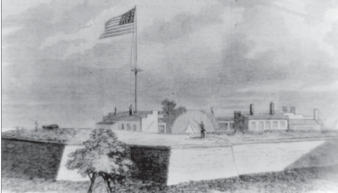
Figure 2.8. This c 1861 engraving from Ballou’s Pictorial depicts a sentinel posted on Bastion II, Columbiads next to star fort, point to Washington Monument and the City of Baltimore. Note the specimen deciduous tree in foreground, and the Columbiad mounted on Bastion I. Fort McHenry Library Special Collection.
