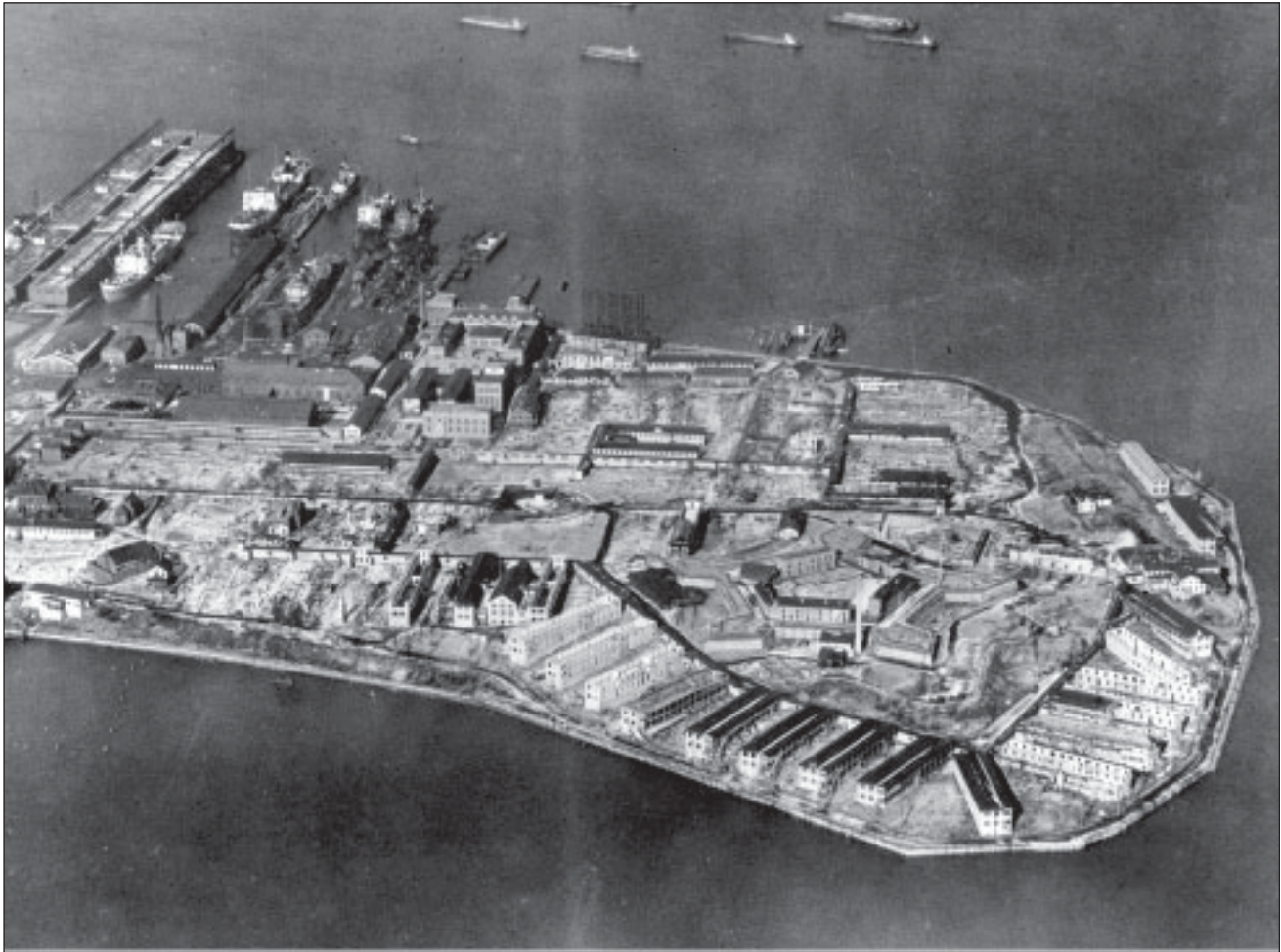
Figure 4.30. This 1926 oblique aerial photograph captures Fort McHenry during the process of demolishing unused hospital buildings. Fort McHenry Library, Special Collections.
