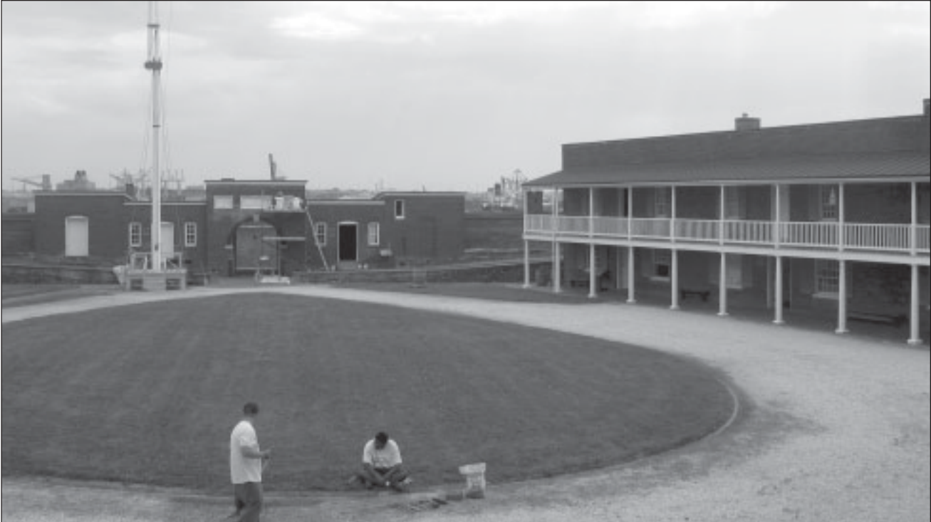
Figure 6.11 The ensemble of historic structures within the Star Fort together create an informal courtyard or parade. The teardrop-shaped carriage turn is believed to have appeared soon after the Civil War. Yet, soon after the historic bombardment the post flagstaff occupied a position on Bastion IV, rather than the location shown above. OCLP, July 2003.
