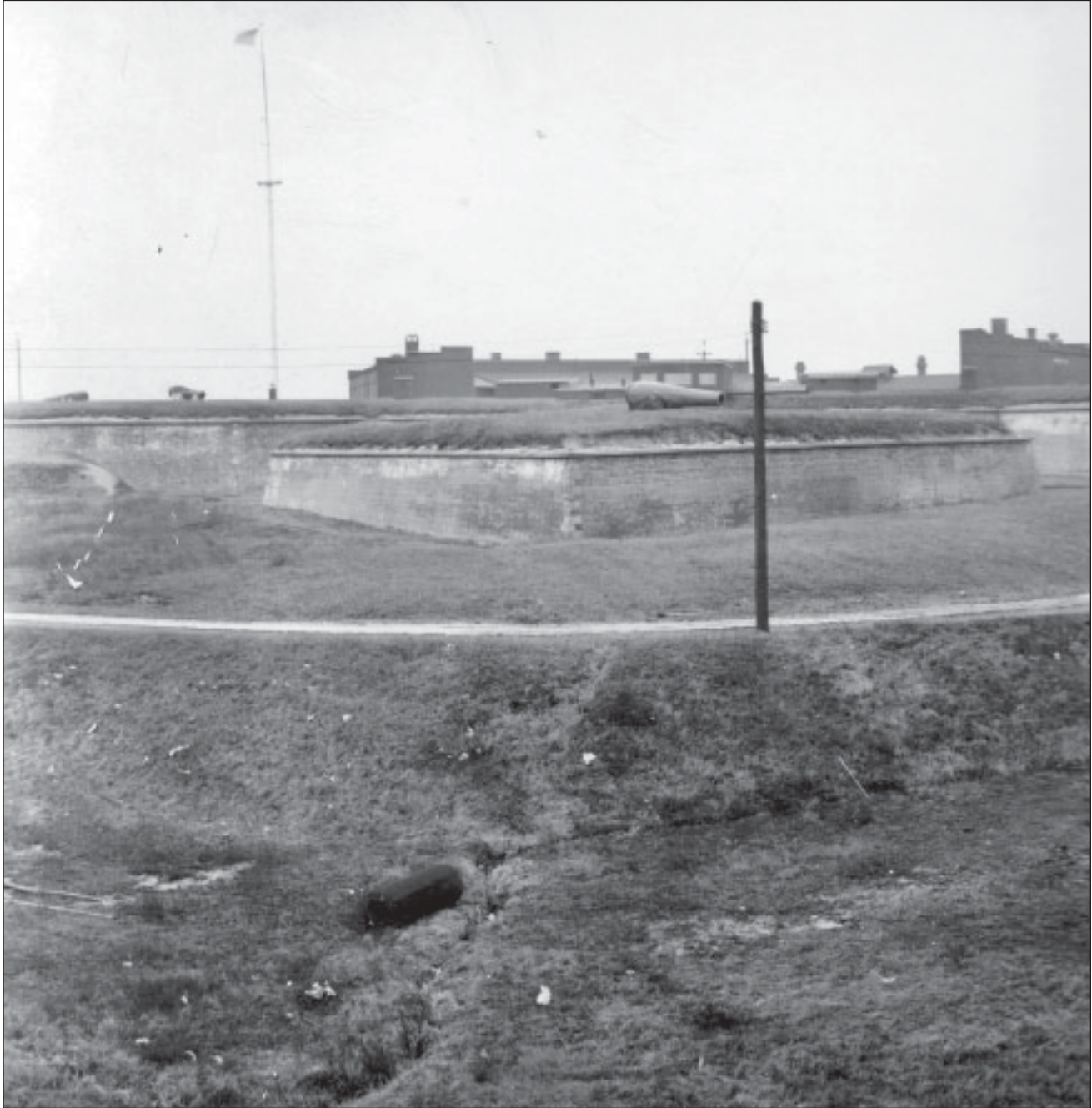
Figure 4.21. Panoramic photograph. This image is paired with Figure 4.22 to the right, depicting landscape conditions during construction of General Hospital #2. Note depth of the dry ditch, still intact in front of the Ravelin. This was removed by the NPS in 1962 during regrading work part of the removal of the War Department's 1930 parking lot. General Hospital #2, Fort McHenry, Balto., MD. J. Henry Miller, Inc. Contractor, 1918. Fort McHenry Library Special Collections, FOMC #2347.
