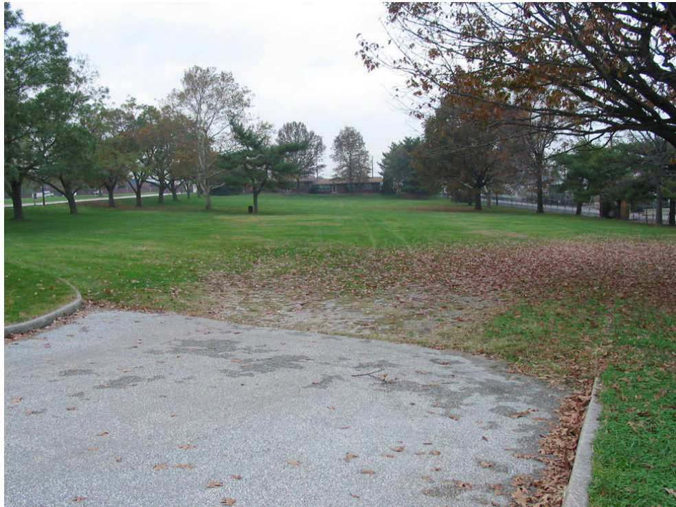
Overflow Parking-Existing Conditions (CRJA, 2003)
