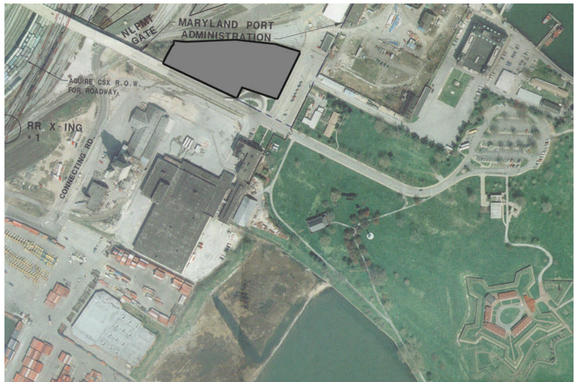
Aerial Photograph of Fort McHenry and Off-site Parking Area (MPA, 2002)
