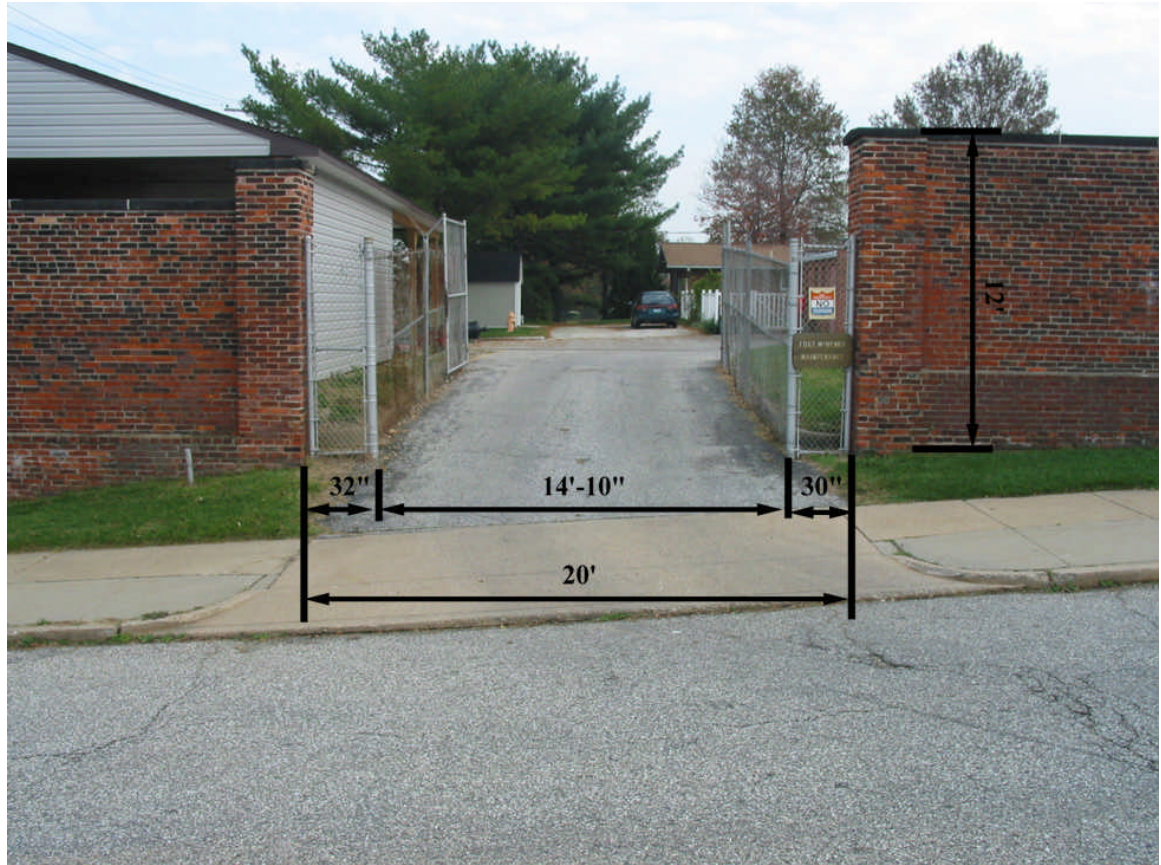
Maintenance Gate-Existing Conditions (CRJA, 2003)
