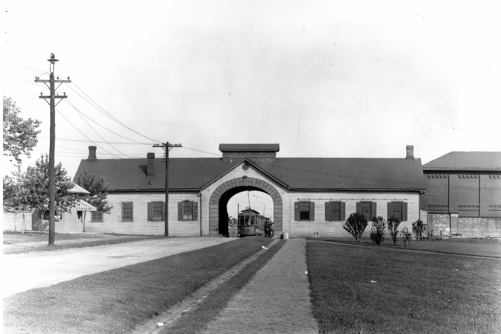
East Fort Avenue Gate-1907-1912 (Provided by the Olmsted Center for Landscape Preservation)
