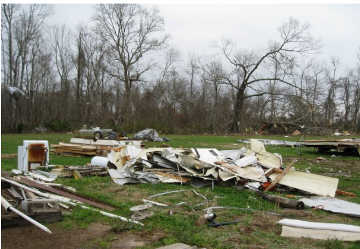
A mobile home was rolled several times and destroyed by an EF1 tornado northeast of Palmetto, Louisiana on February 17, 2008 (photo by Sam Shamburger, forecaster)
