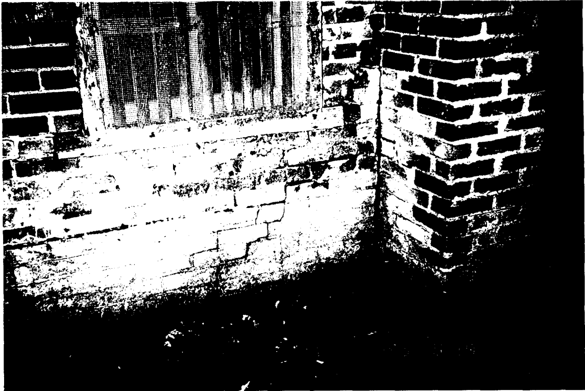
151-S South Slave Cabin - Deteriorated brick on inside of basement walls. (RSA)
