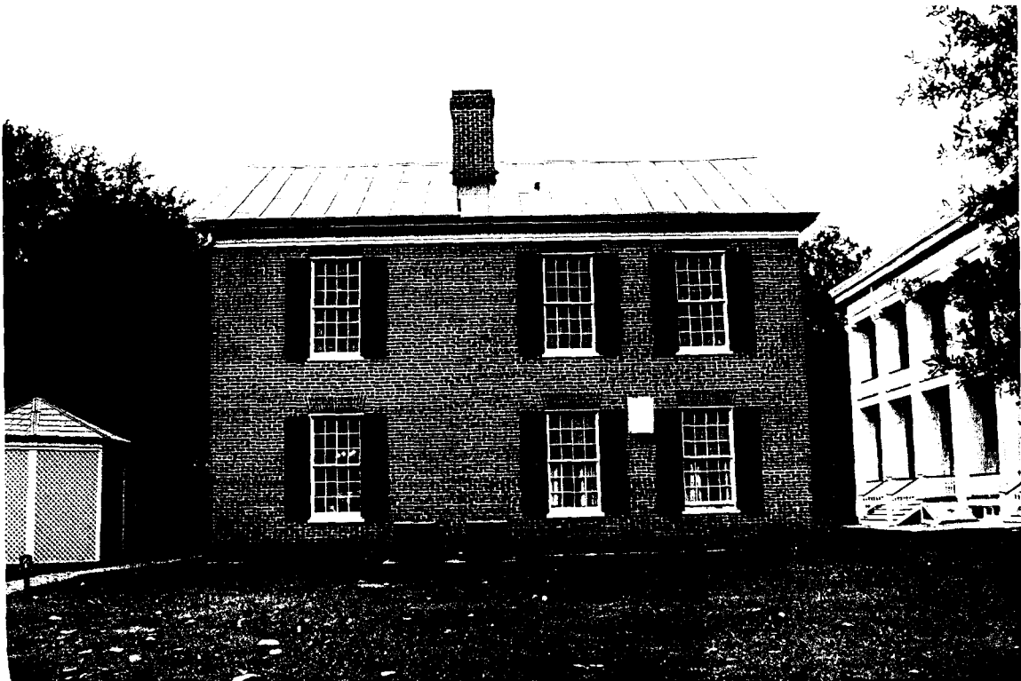
99-A Kitchen - Sagging in roof. (ABA)
