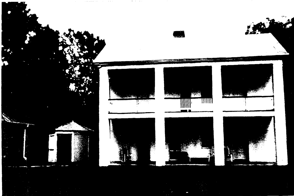
101-A Dairy - North Elevation (ABA)
