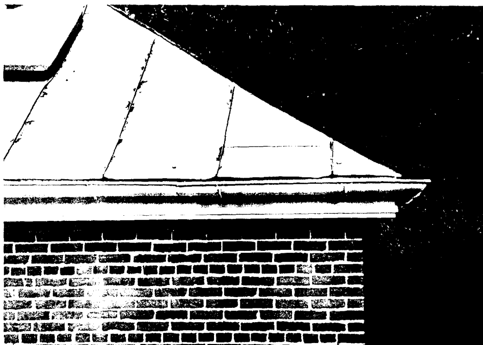
165-A Smokehouse - Sags in gutters. (ABA)
