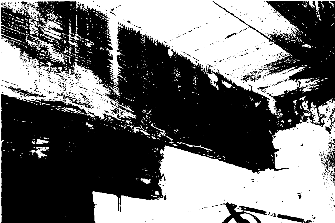
86-S Main House - Insect damage to wood under south porch. (RSA)
