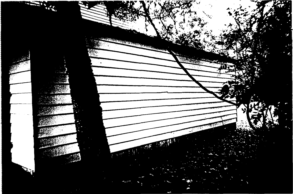
118-A Carriage House - Lack of gutter on north side. (ABA)
