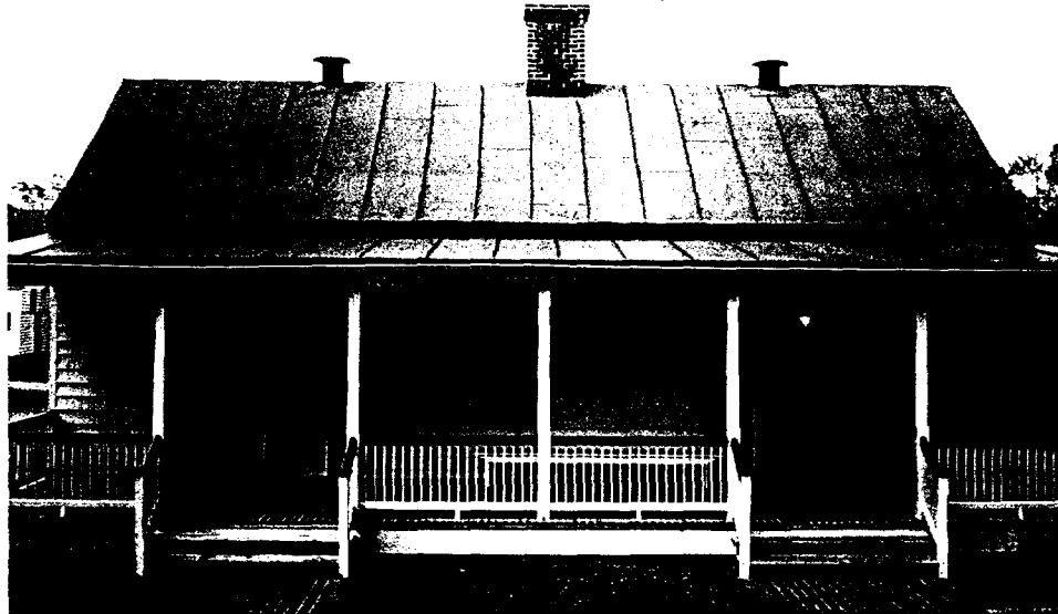
140-A North Slave Cabin - Non-historic roof vents. (ABA)
