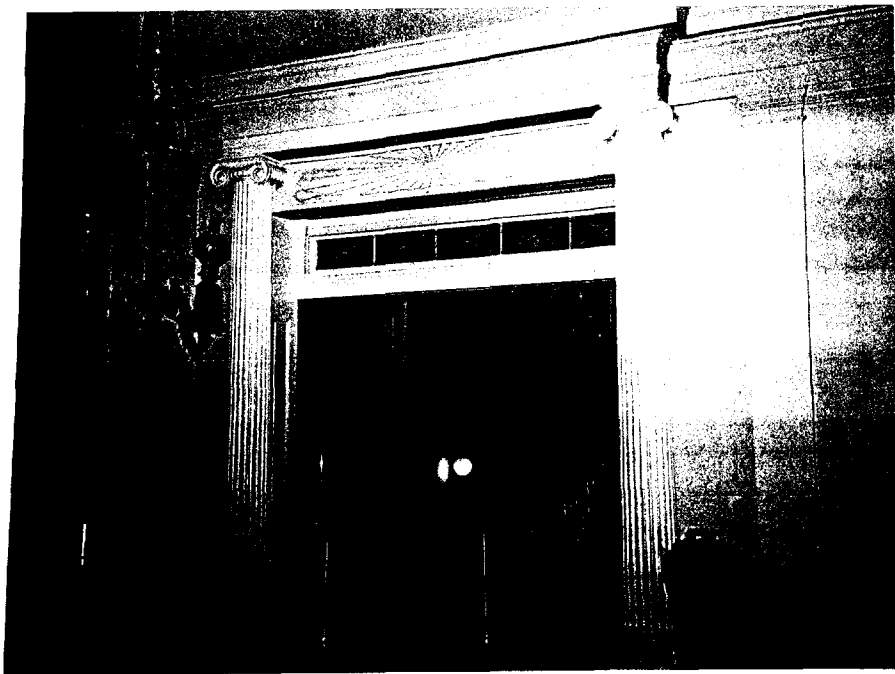
74-A Main House - Doorway between Saloon and Stairhall. (ABA)
