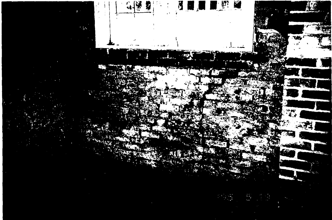
79-S Main House - Crack in southeast corner of basement. (Robert Silman Associates - RSA)
