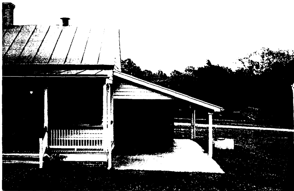
139-A North Slave Cabin - Downspout at southwest corner does not discharge onto a sloped grade. (ABA)
