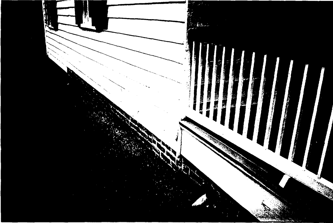
142-A North Slave Cabin - Loose siding at floor line on north wall. (ABA)
