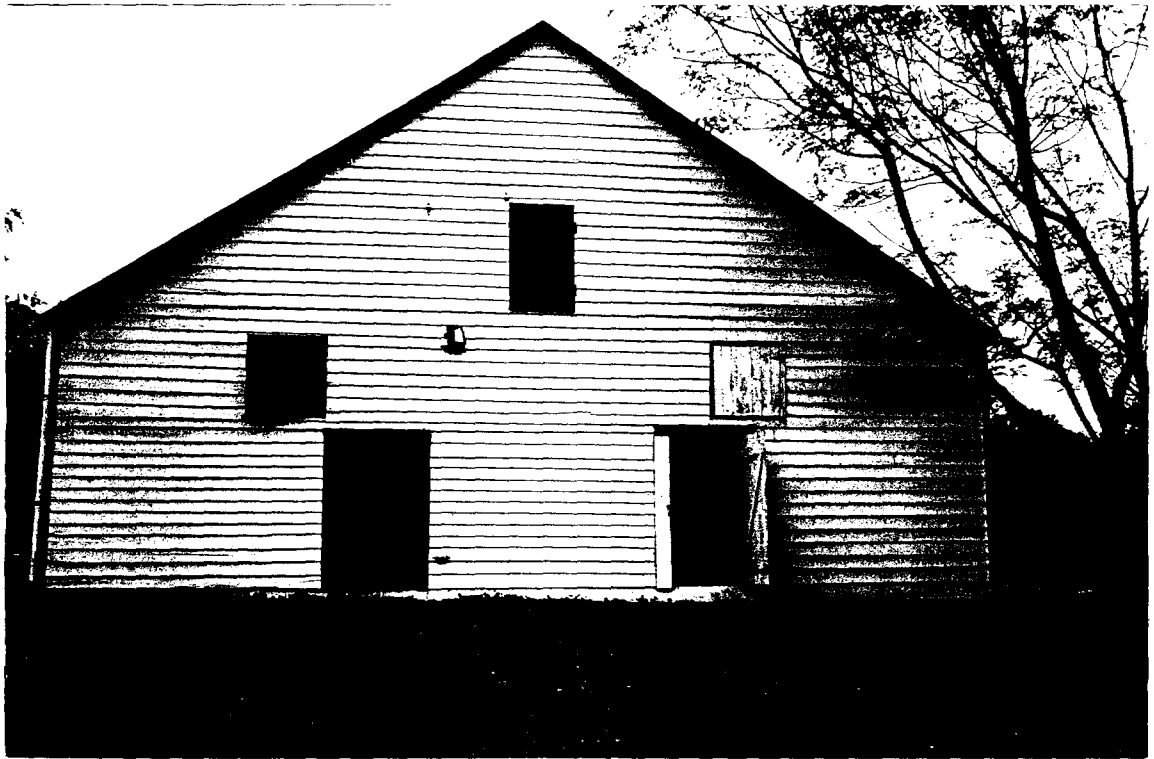
127-A Stable - South Elevation (RRA)
