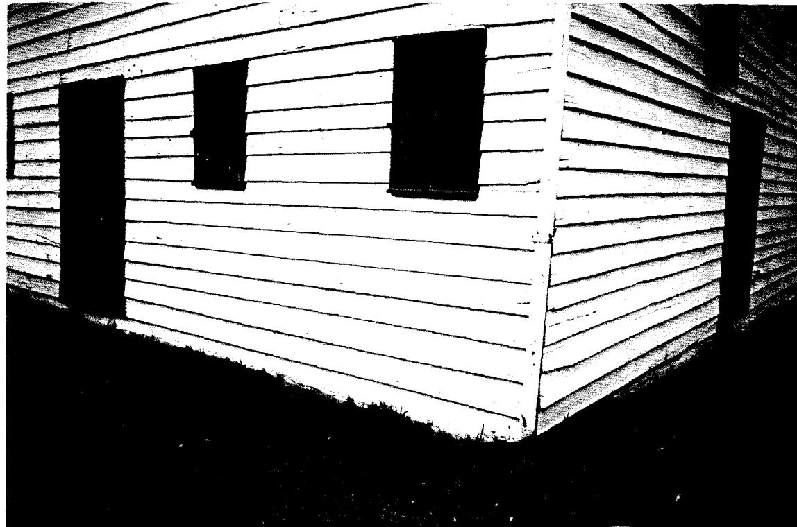
133-A Stable - Rotting wood and peeling paint on west wall. (ABA)
