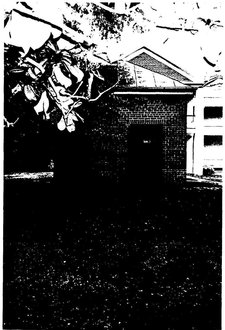
157-A Privy - East Elevation (RRA)
