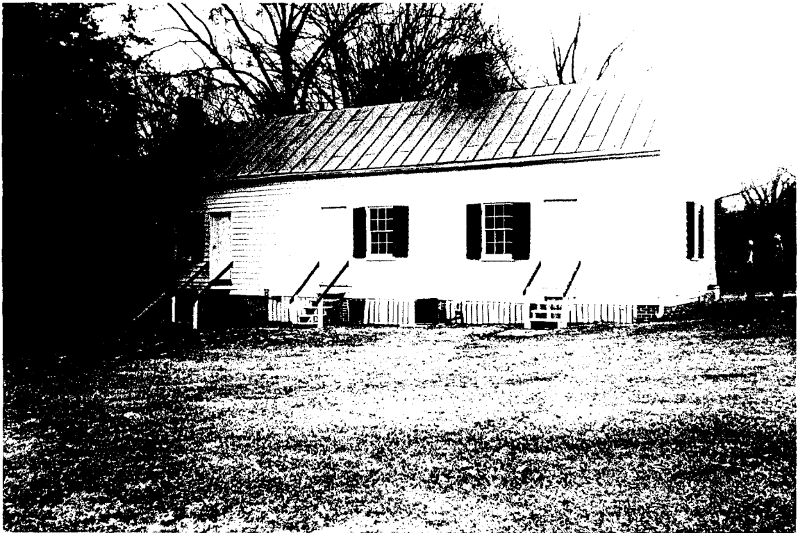
144-A South Slave Cabin - East Elevation (RRA)
