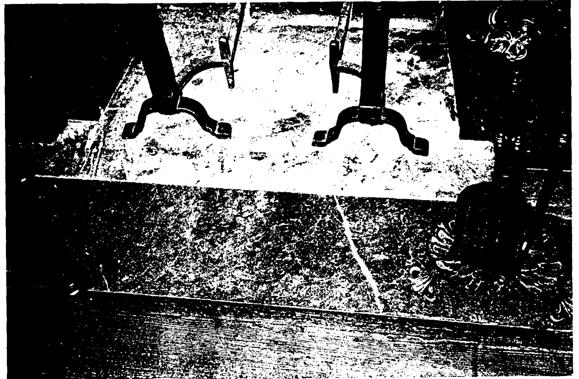
66-A Main House - Crack in fireplace hearth in Middle Bedroom. (ABA)
