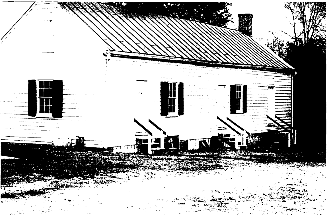
145-A South Slave Cabin - West Elevation (RRA)
