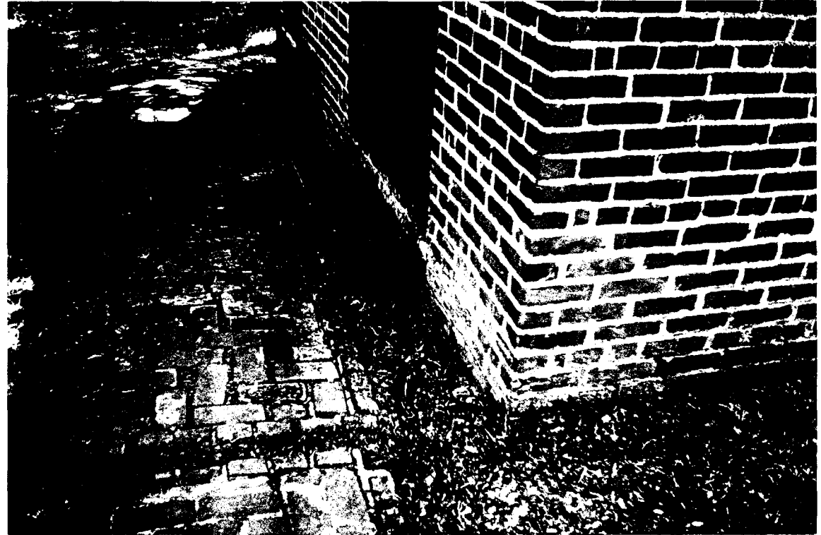
159-A Privy - Deteriorated brick at corner. (ABA)
