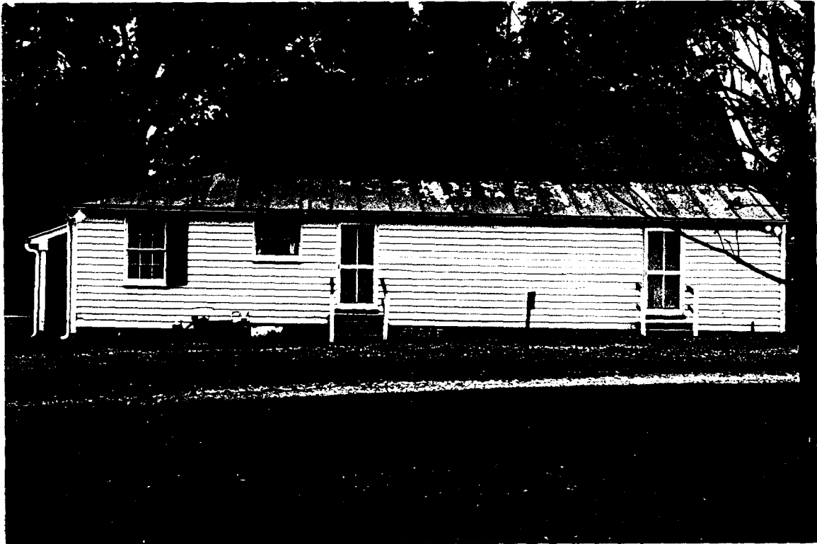
134-A North Slave Cabin - East Elevation (RRA)
