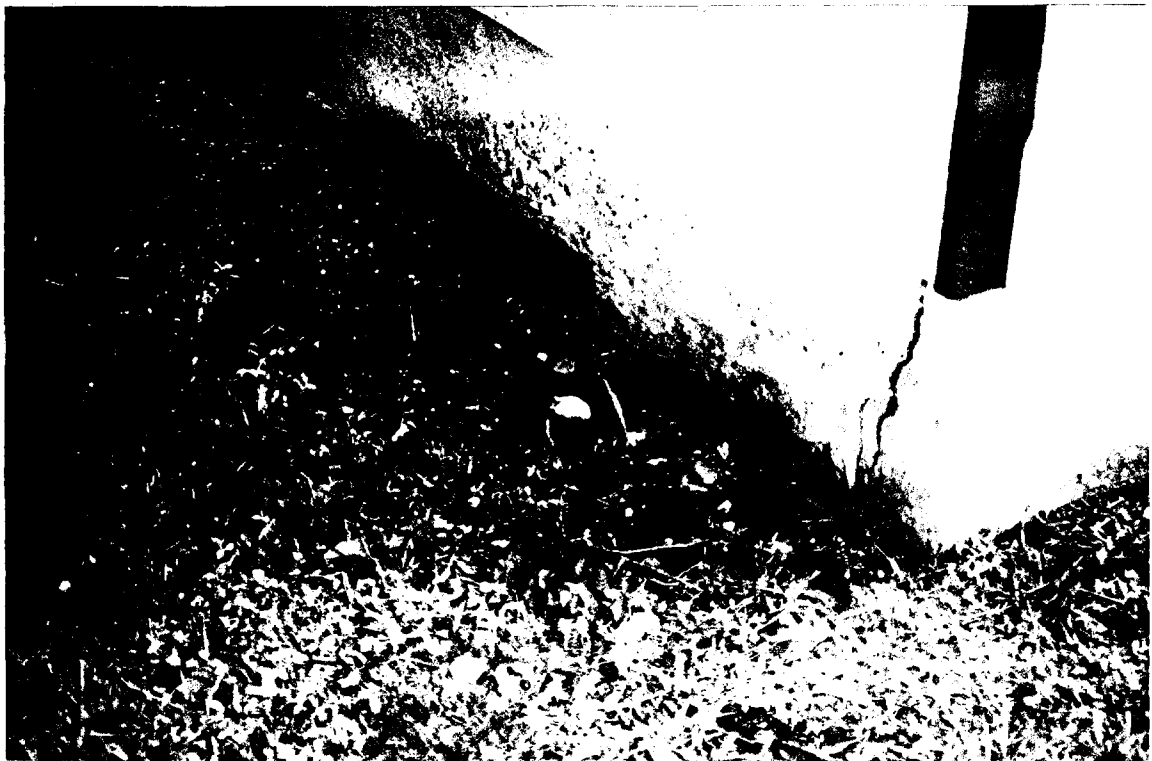
119-A Carriage House - Cracked concrete foundation wall at northeast corner of shed. (ABA)
