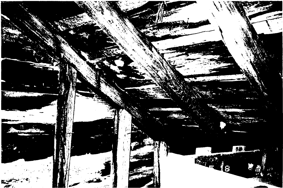
123-S Carriage House - Water infiltration to wood roof framing. (RSA)
