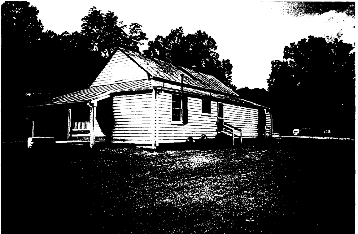
137-A North Slave Cabin - South Elevation (RRA)
