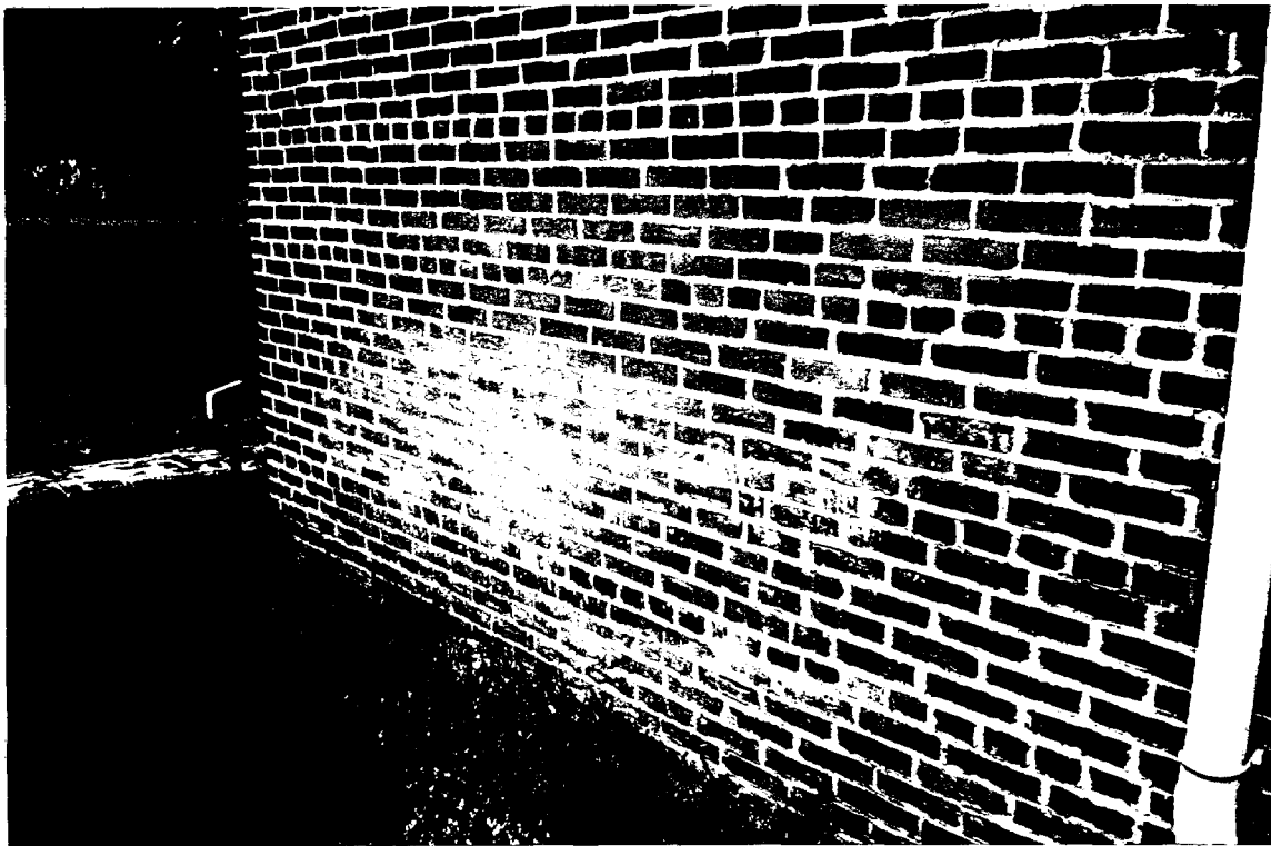
161-A Privy - Visually incompatible restoration attempts on brick walls. (ABA)
