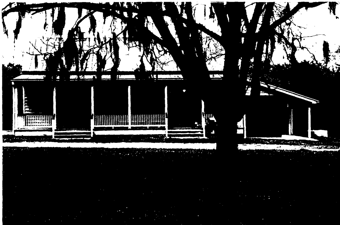
135-A North Slave Cabin - West Elevation (RRA)
