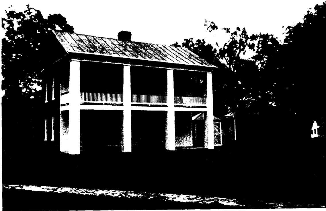
95-A Kitchen - South Elevation (ABA)
