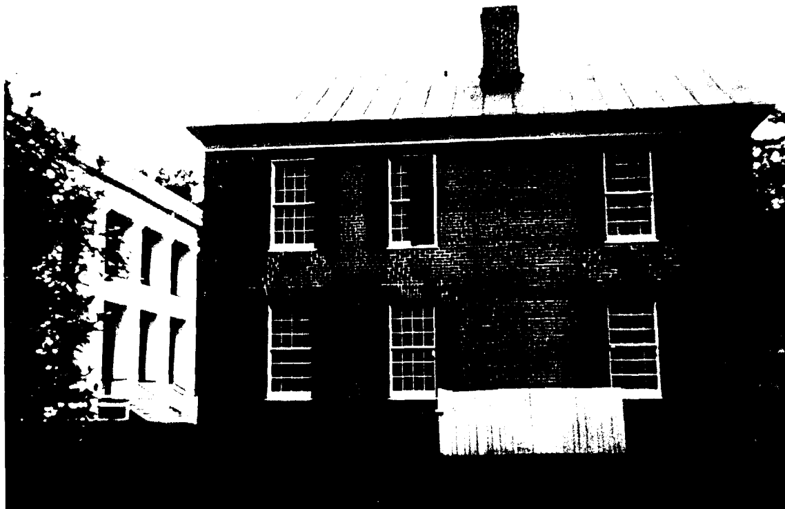
103-A Dairy - South Elevation (ABA)
