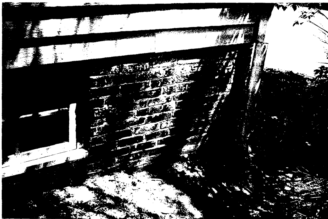
149-A South Slave Cabin - Bowing south brick wall of cellar. (ABA)
