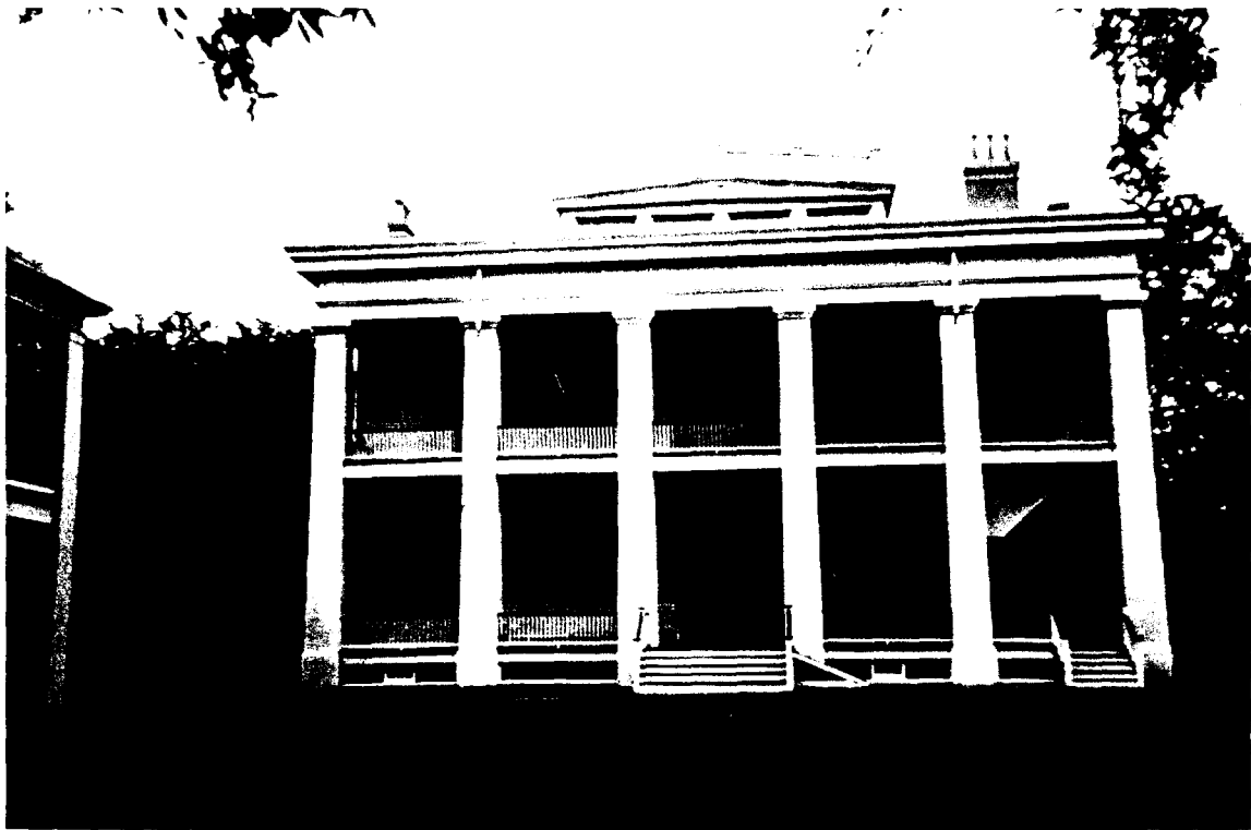
48-A Main House - East Elevation (ABA)
