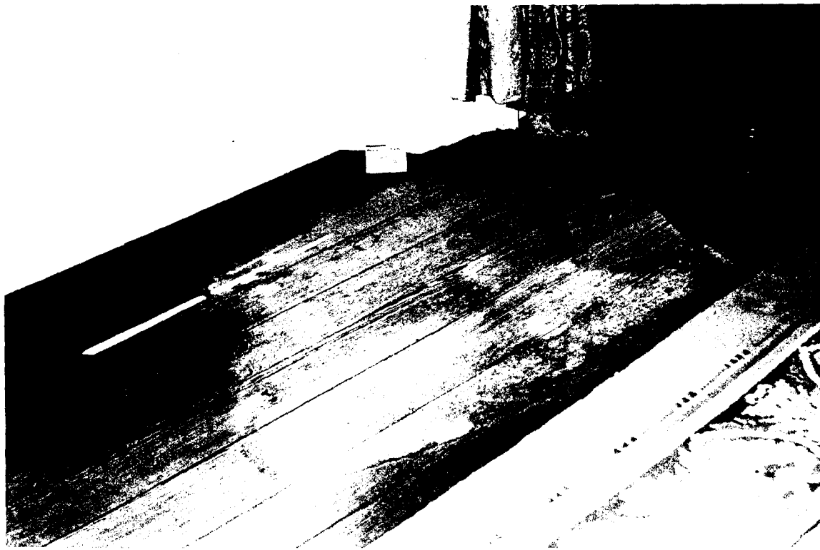
62-A Main House - Floor damage caused by humidifiers. (ABA)
