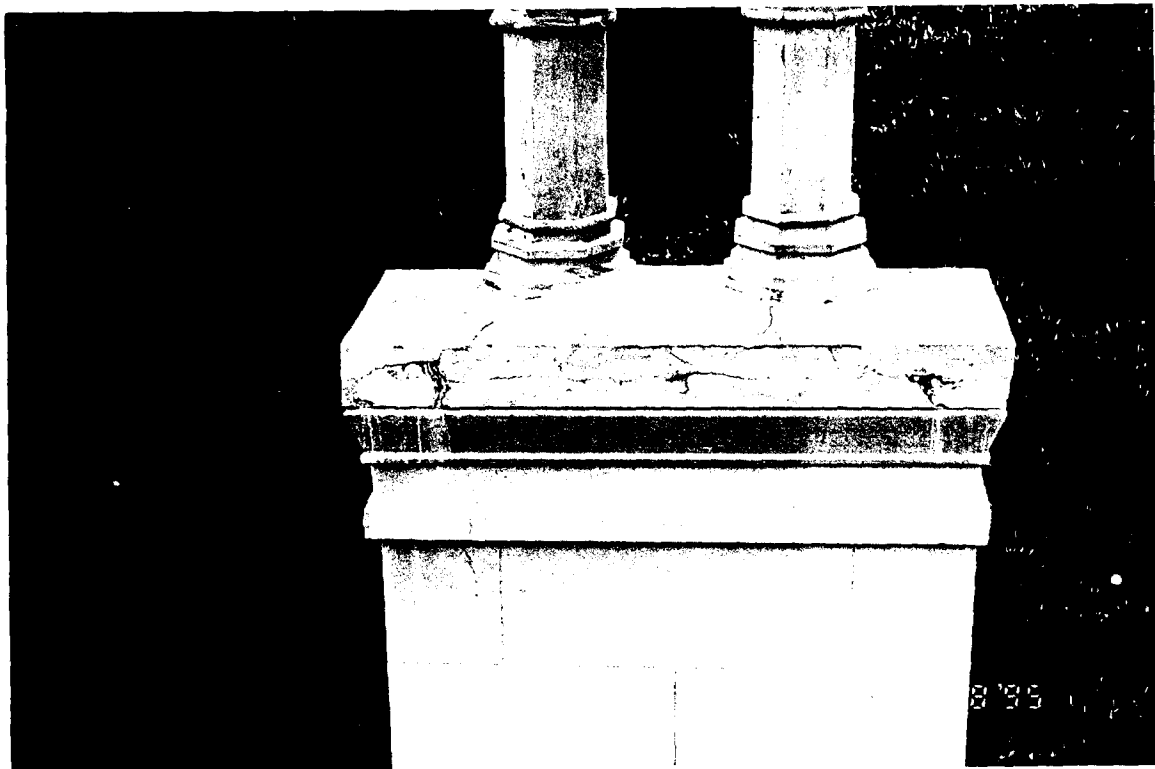
54-A Main House - Spalling at chimneys. (ABA)
