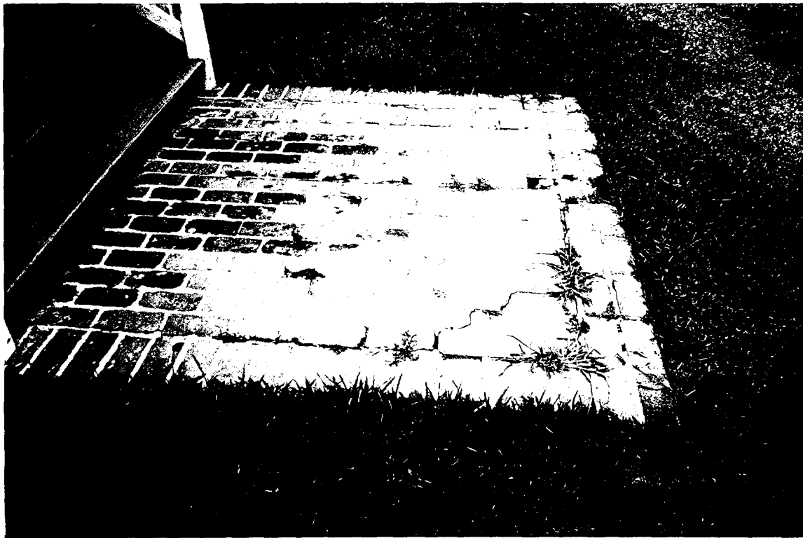
138-A North Slave Cabin - Brick landings with loss of mortar and settlement. (ABA)
