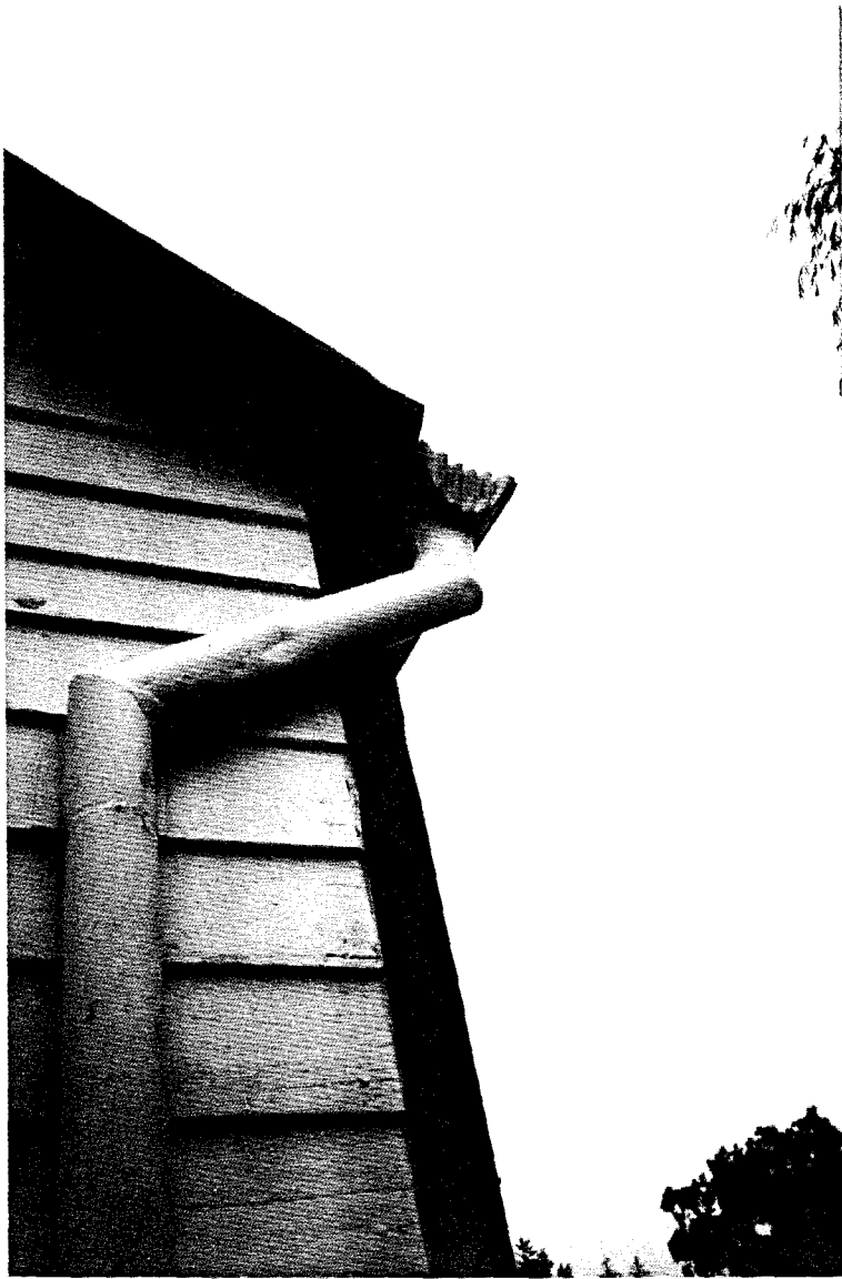
128-A Stable - Metal roofing turned down and nailed into eaves and rakes. (ABA)
