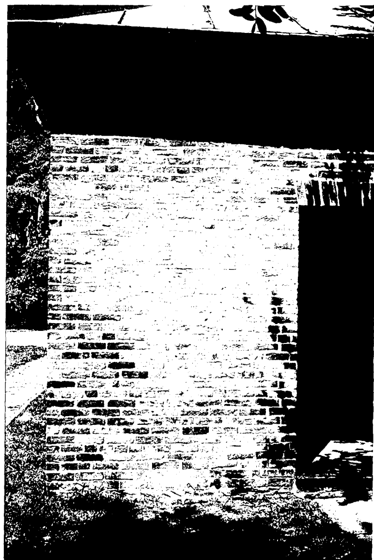
166-A Smokehouse - Deteriorated bricks below floor line. (ABA)
