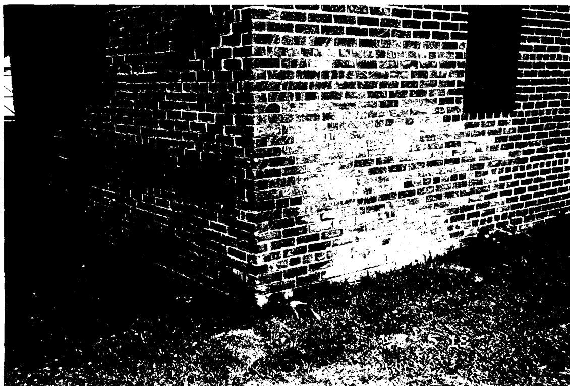
171-S Smokehouse - Rising damp and related damage to masonry. (RSA)
