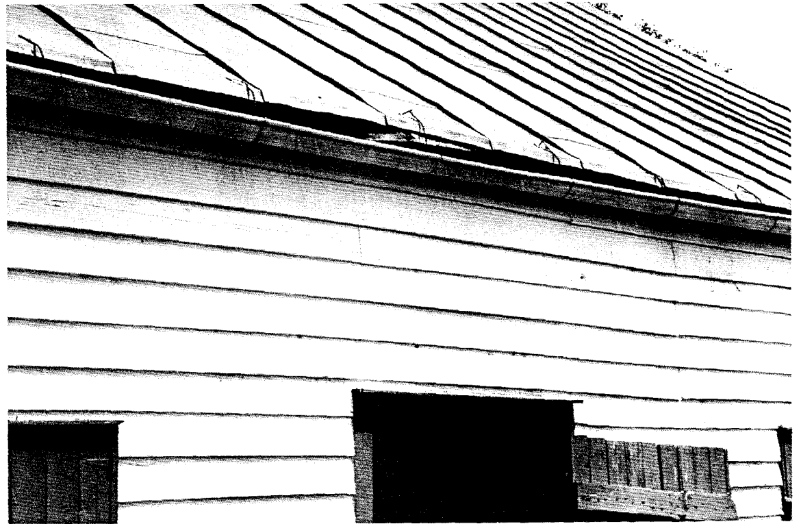
129-A Stable - Hanging gutters. (ABA)
