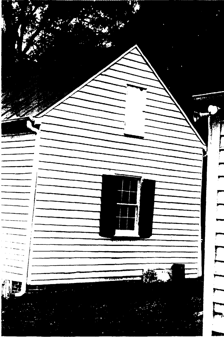
146-A South Slave Cabin - North Elevation (RRA)
