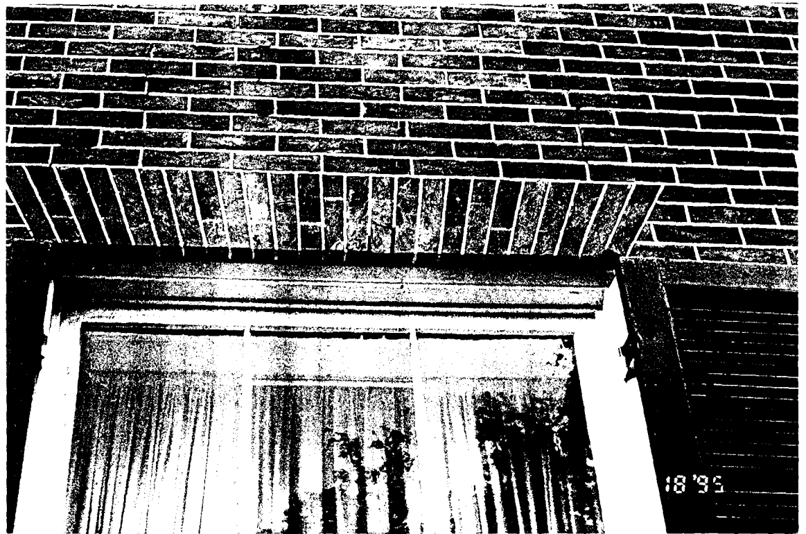
56-A Main House - Mortar loss at jack arch. (ABA)
