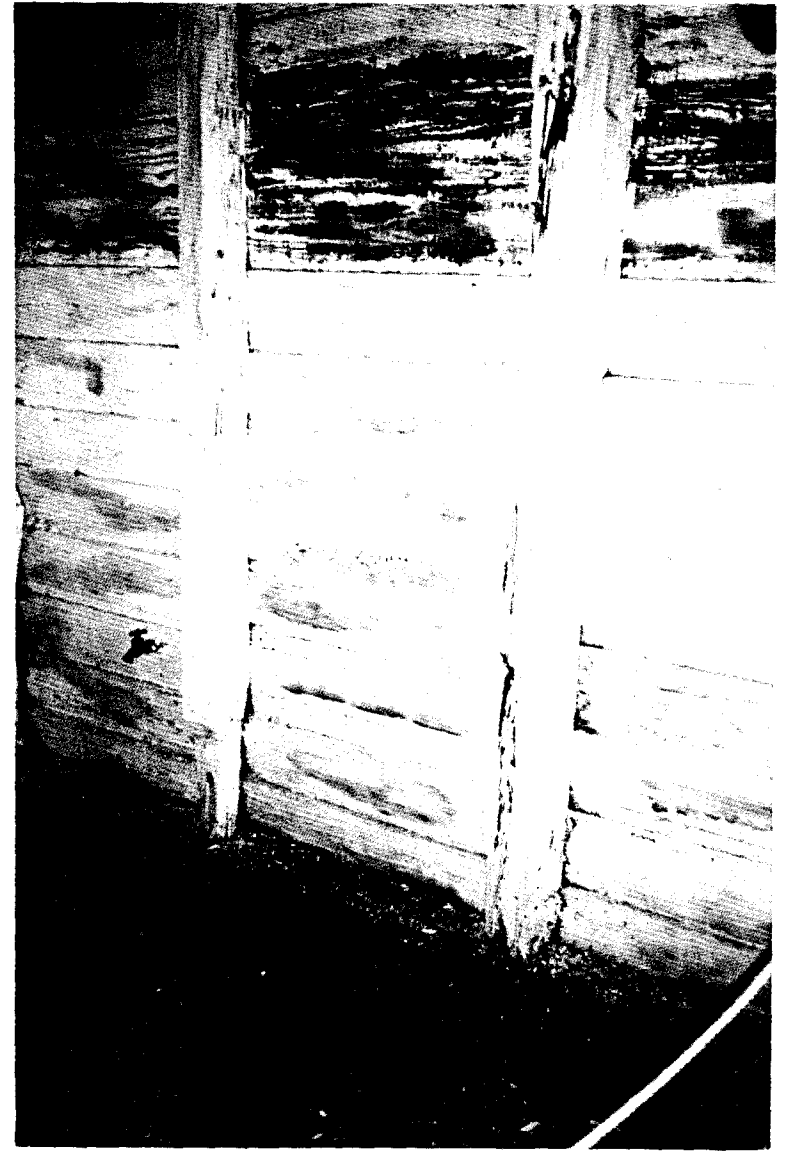
131-A Stable - Rotted and insect damaged columns, interior view. (ABA)
