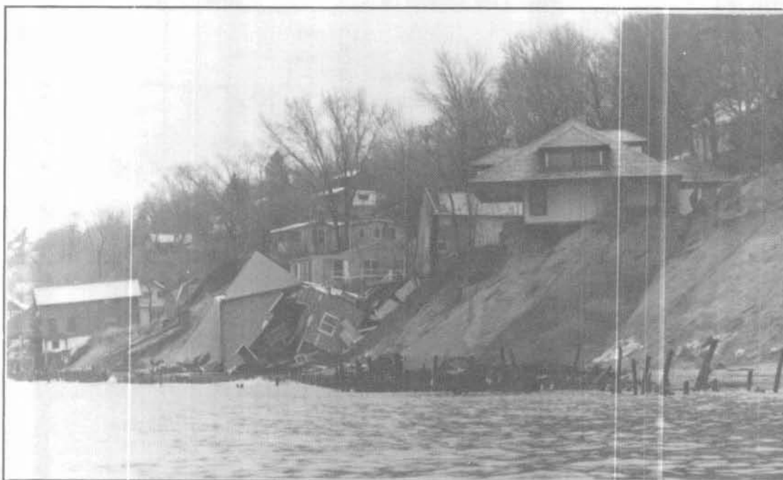
Storms during high lake levels cause severe damage to shorelines.
