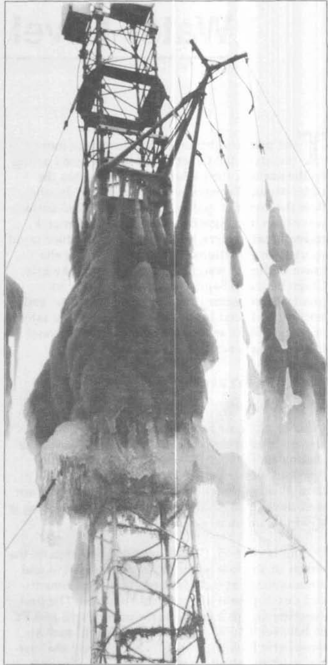
Figure 19. A wave tower used on Lake St. Clair during the GLERL–NWRI study on wave processes. Ice formed on the tower before it was retrieved December 1986.
