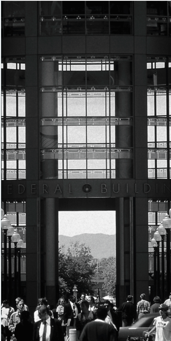
Oakland Federal Building, Oakland, CA
