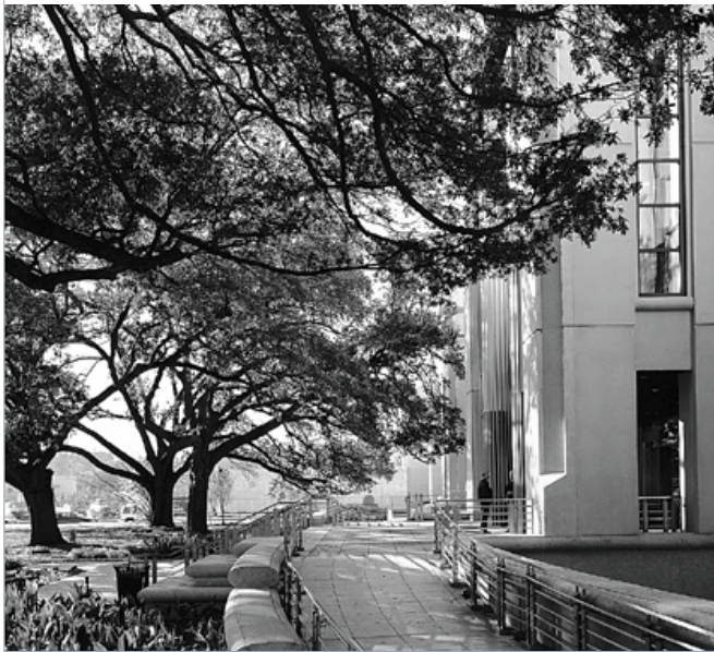
Russell B. Long Federal Building and United States Courthouse
