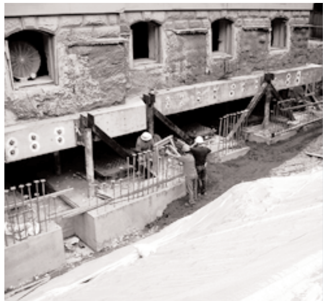
Base isolator installation at the historic Pioneer Courthouse, Portland, OR
