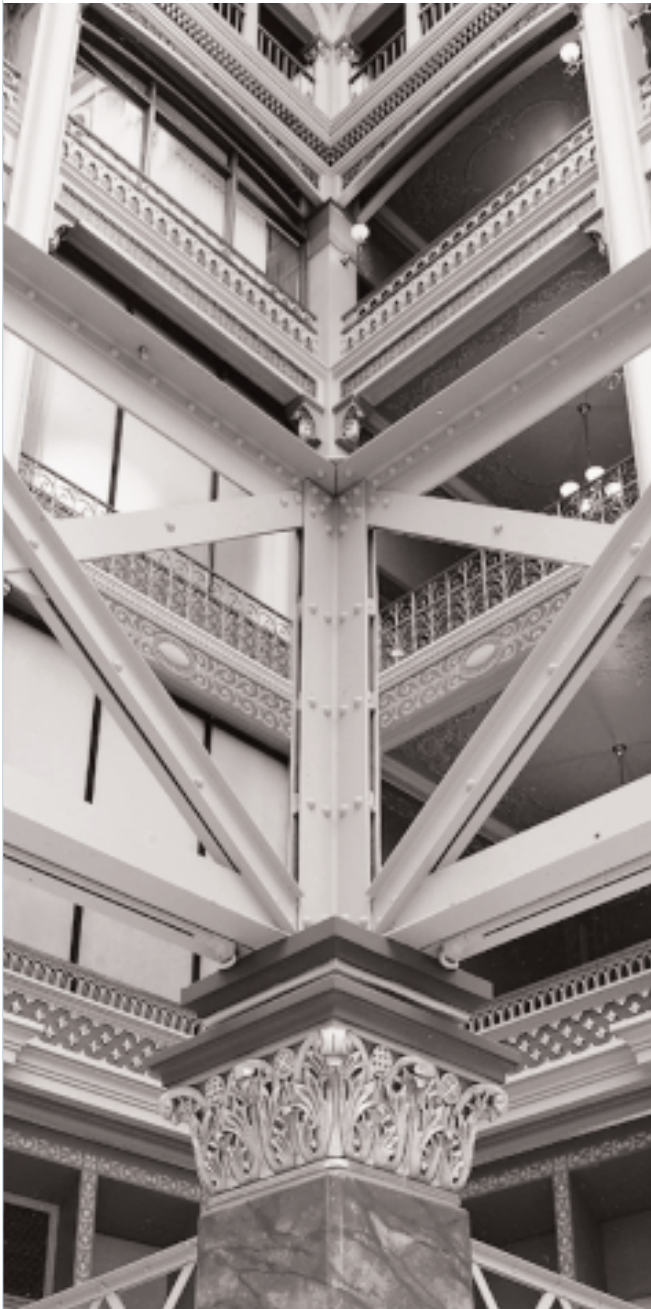
Steel bracing in the Milwaukee Courthouse
