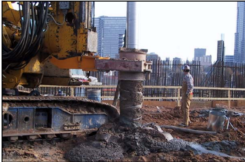
(a) Full Displacement Pile
