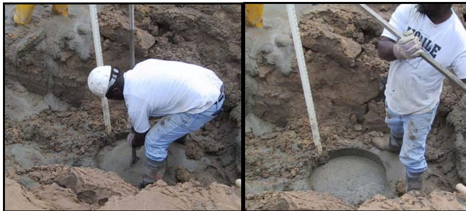
(c) and (d) Contaminated Grout Removal
