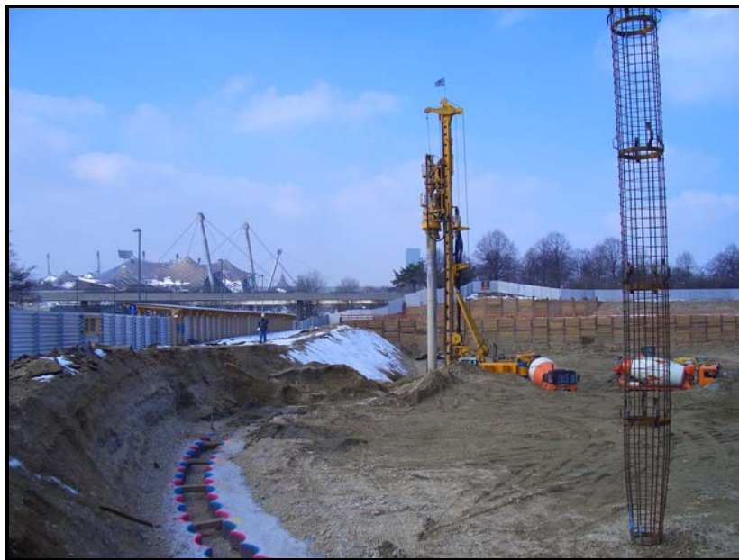
Figure 3.15: Drilling CFA Piles through Guide for Secant Wall
