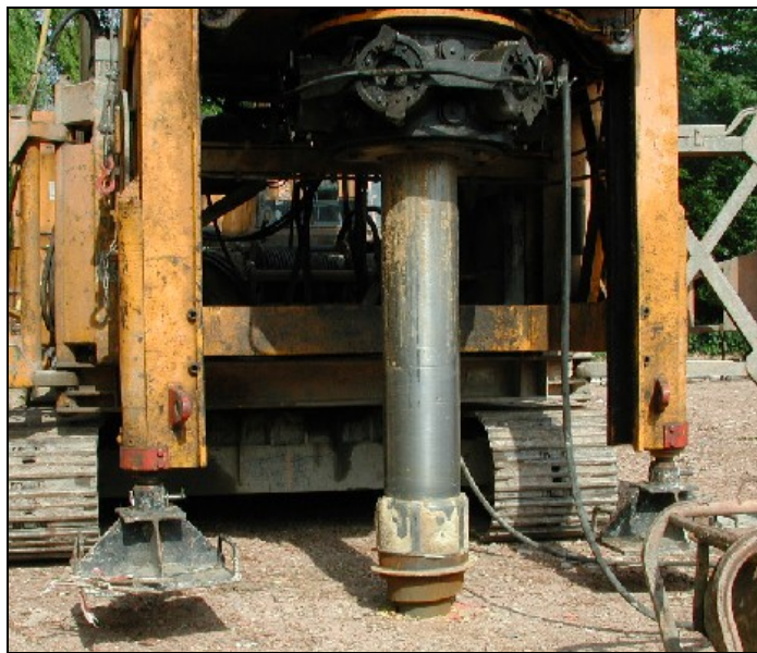
Figure 4.13: Fundex Screw Pile
