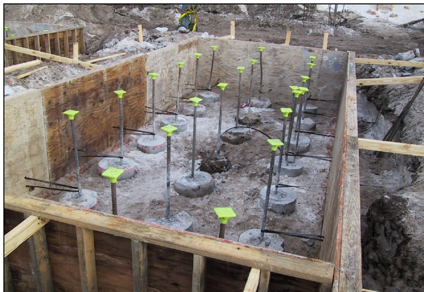
Figure 2.4: Group of CFA Piles with Form for Pile Cap
