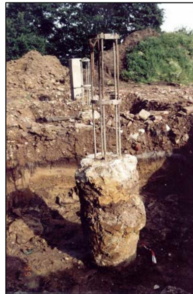
Figure 4.13: Fundex Screw Pile
