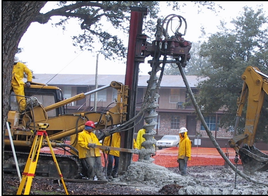
Figure 3.4: Low Headroom CFA Pile Application
