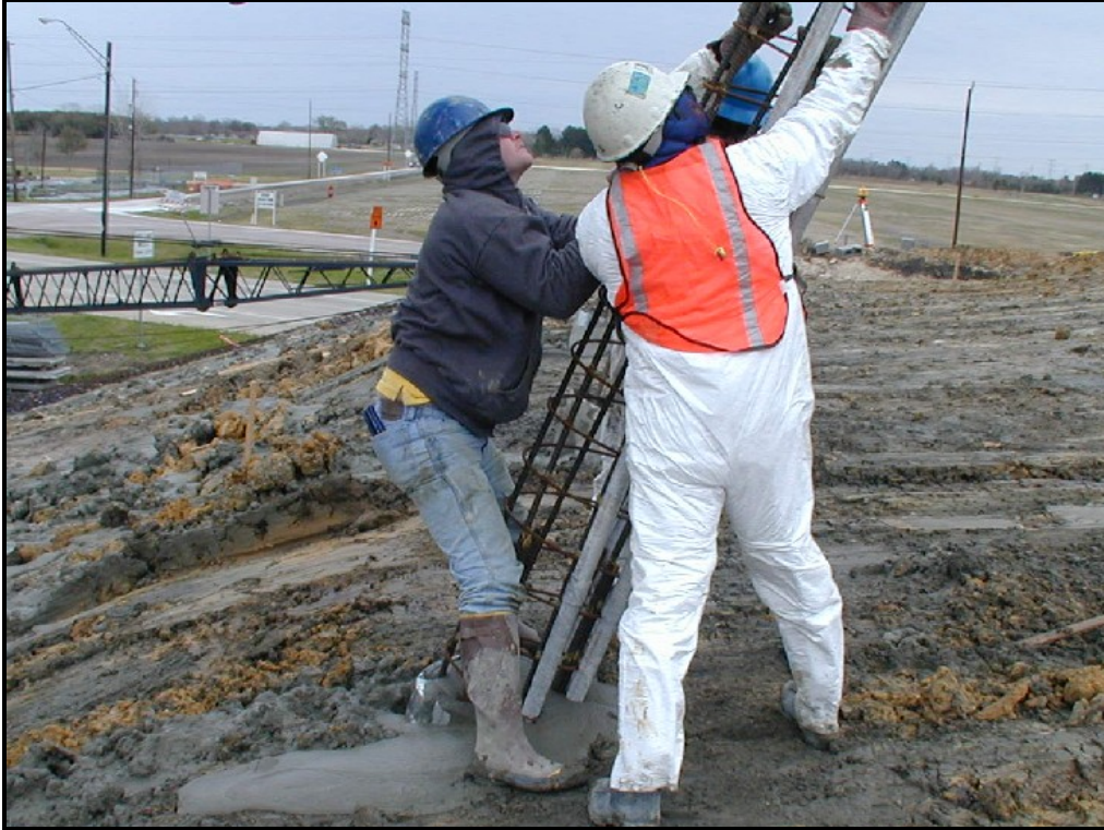
Figure 4.26: Installation of Reinforcement Cage into Battered CFA Pile
