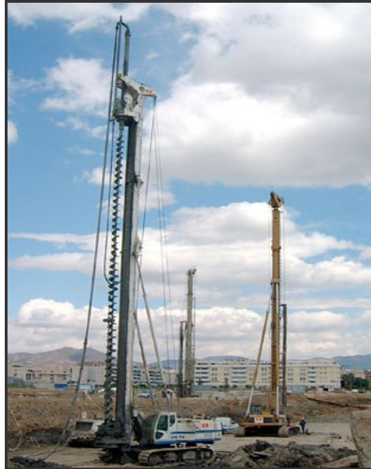
Figure 4.6: Soilmec Hydraulic CFA Rig with Kelly-Bar Extension
