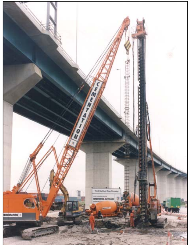
Figure 3.3: CFA Piles at Bridge Interchange
