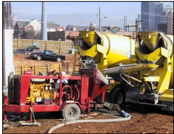
Figure 2.8: Grout Delivered to Pump
