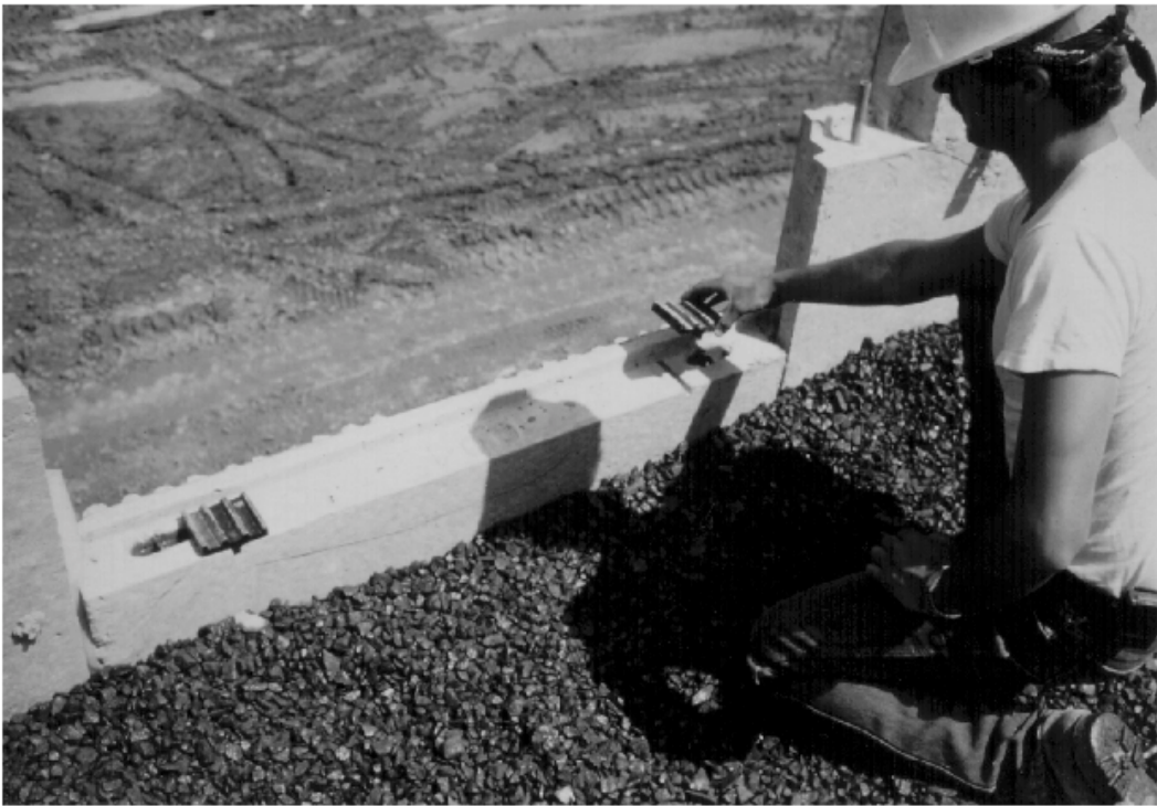
Figure 86. Geotextile joint cover and neoprene pads.
