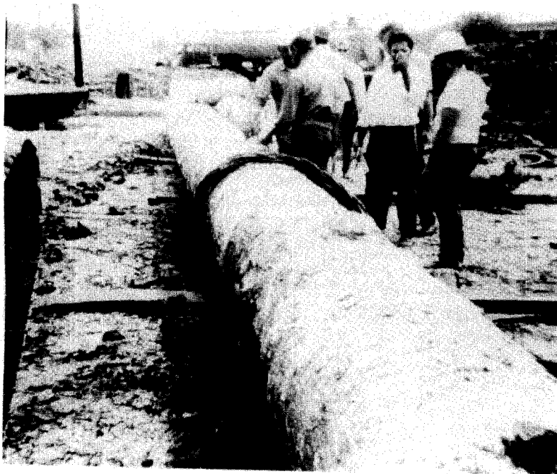
Figure 8.19 b. Drilled shaft of excellent quality after exhumation
