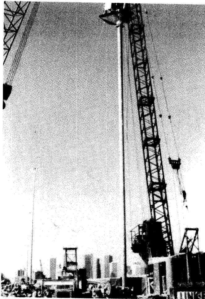
Figure 8.11. Photograph of gravity-fed tremie partially extracted
