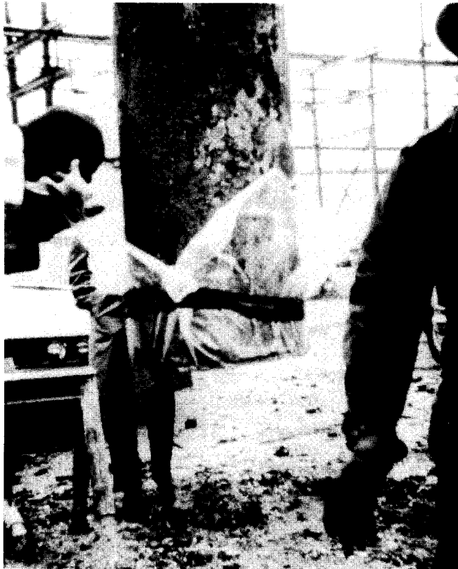
Figure 8.10. Photograph of simple plywood loose plate closure on a gravity-fed tremie
