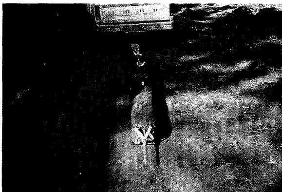
P50. Exhumed sacrificial test nail. Note lack of grout from bottom centralizer to tip of nail. Problem resulted from (1) not placing tremie grout pipe completely to bottom of drillhole; and (2) using too stiff a grout (e.g., shotcrete mix).
