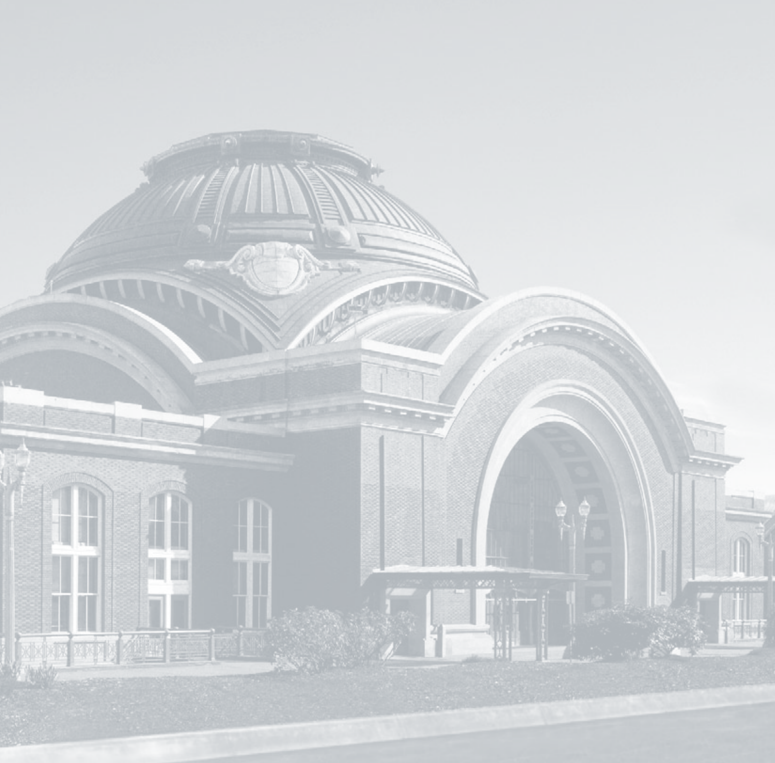
U.S. COURTHOUSE TACOMA, WA, 1909-1911, 1992
