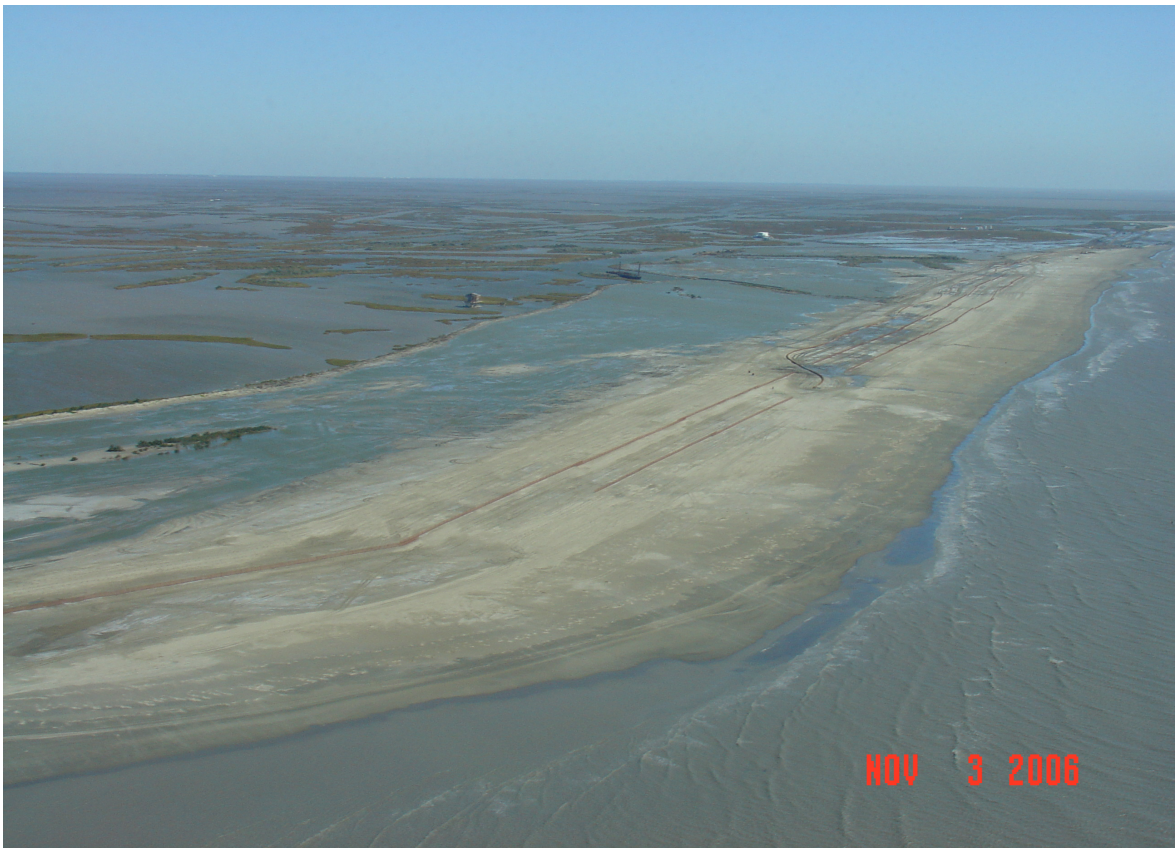
Figure 5-3. Barrier Island Project Nearing Completion in Fall 2006
