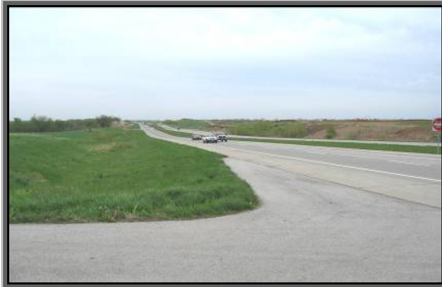
PHOTOGRAPH No. 19: LOOKING EAST ON MISSOURI HIGHWAY 150 FROM THE BOTTS ROAD INTERSECTION
