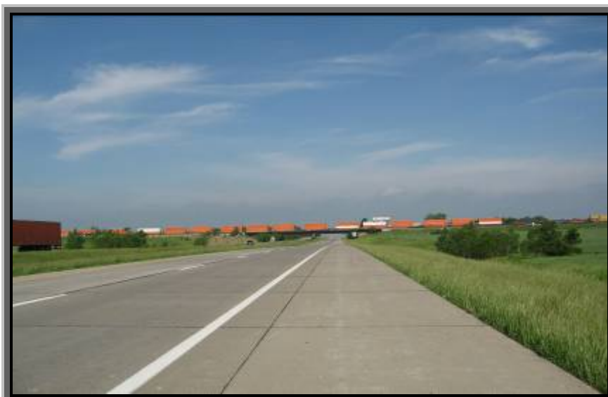
PHOTOGRAPH No. 21: THE KANSAS CITY SOUTHERN RAILROAD BRIDGE OVER MISSOURI HIGHWAY 150 AT THE SOUTHWEST CORNER OF THE REDEVELOPMENT AREA
