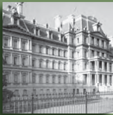
Dwight D. Eisenhower Executive Office Bldg. Washington, DC
