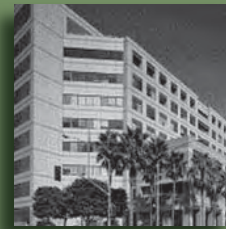
Glenn M. Anderson Federal Bldg. Long Beach, CA
