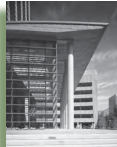
U.S. Courthouse Seattle, WA
