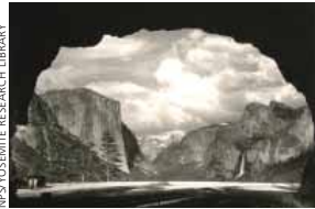
View exiting Wawona Tunnel, 1930s.
