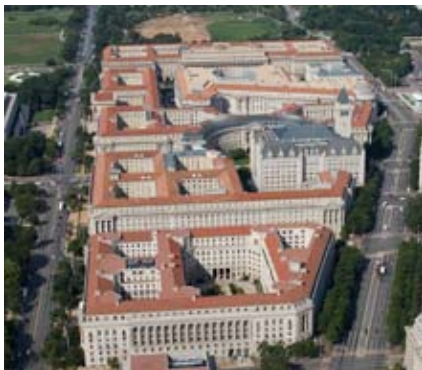
FIGURE 1 Clay tile roofing dominates and unifies aerial views of Washington's Federal Triangle, a vantage point also enjoyed by visitors to the Old Post Office tower in the center of the complex. Tile roof repairs require special care to achieve consistent color distribution across an entire roof.
