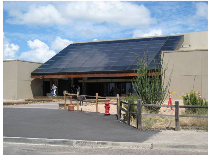
A large array of solar panels marks the main entry into the newly renovated Visitor Center. (NPS photo by Stan Allison)
