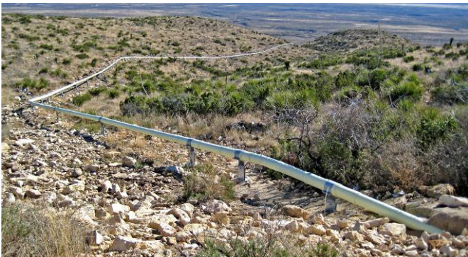
The completion in the summer of 2008 of a new double-walled outfall sewer line from the Visitor Center to sewage lagoons off the escarpment is a major milestone in the long-term protection of Carlsbad Cavern. (NPS Photo by Dale Pate)
