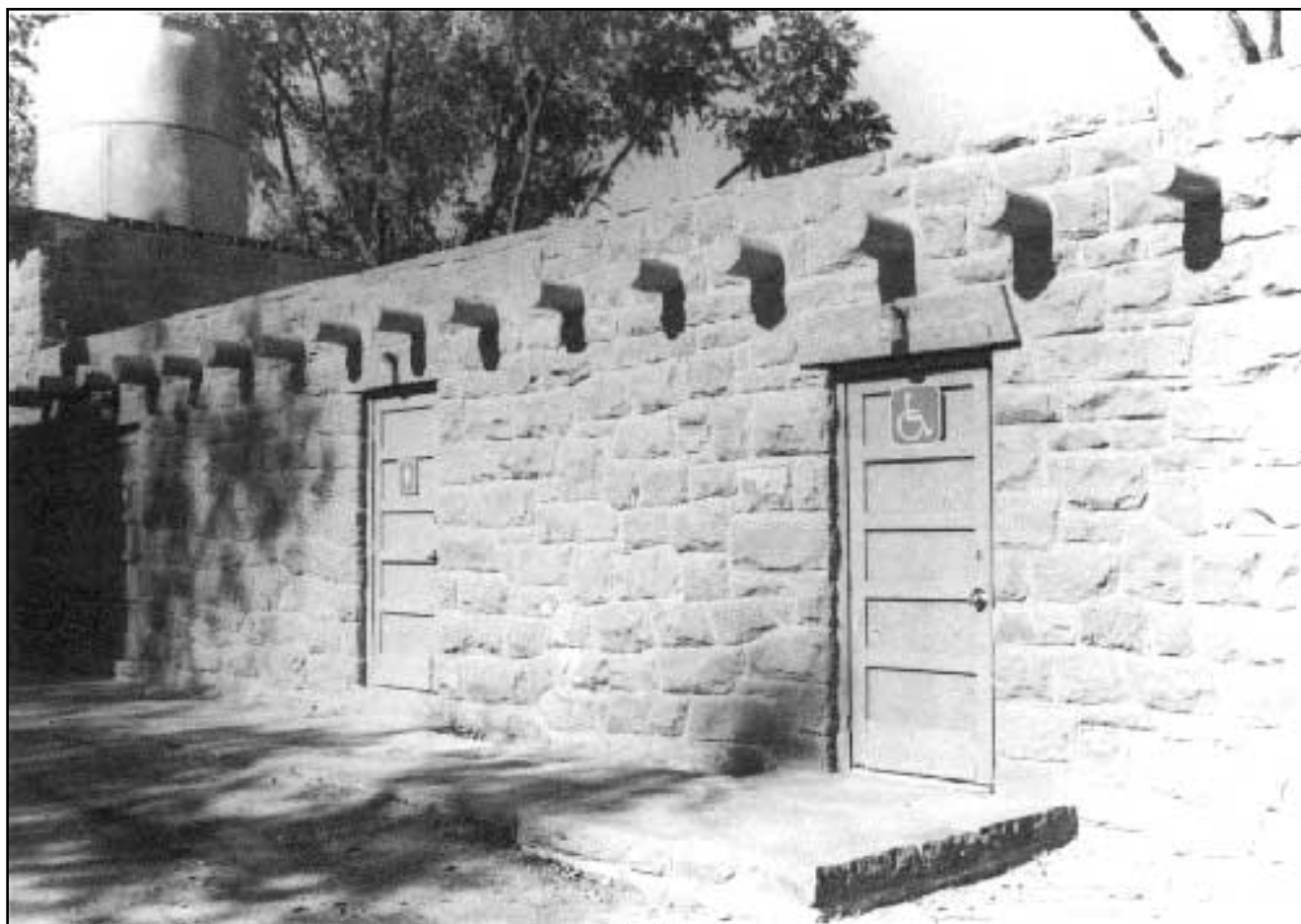
Figure 35. The Restrooms, HB-13, were converted to their present use in 1980. The building was formerly a pump house. NPS photo by E. Bauer, October, 1984, HUTR Neg. R74#34.
