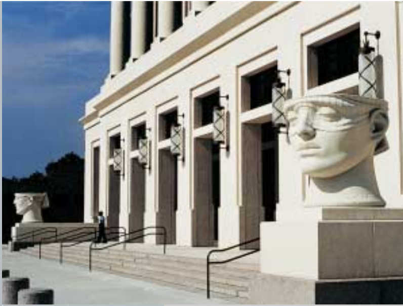
1998 JOHN M. SHAW U.S. COURTHOUSE LAFAYETTE, LOUISIANA
