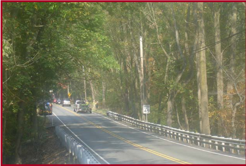
Tree canopy on PA 663. Guide rail with turn down end treatment
