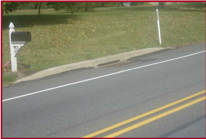
Drainage inlet south of Little Road
