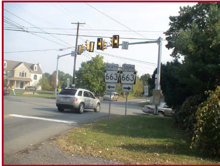
Kutztown Road eastbound approach to PA 663
