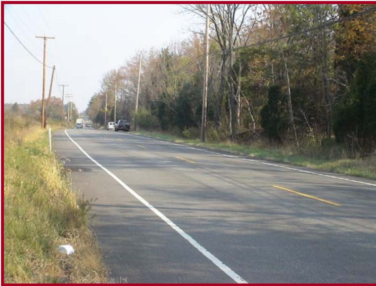
Passing zone on PA 663 approaching between PA 73 and Hoffmansville Road
