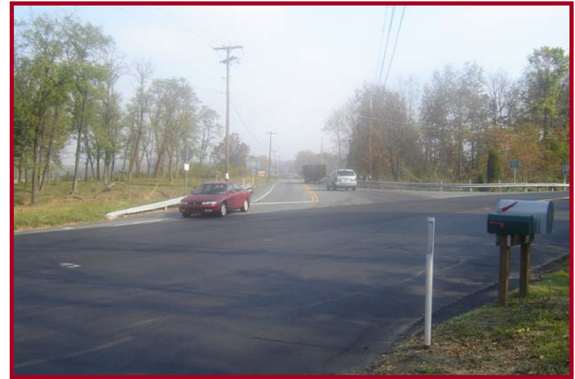
Intersection of PA 73 (Big Road) and Layfield Road (PA 663) looking north – skewed
