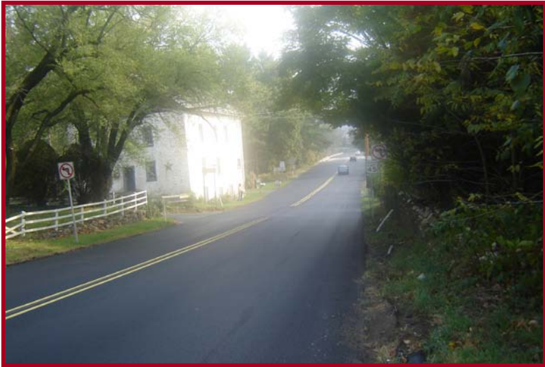
PA 73 (Big Road) looking east at the Ludwig Road intersection – crumbling rock wall and damaged delineators on the right
