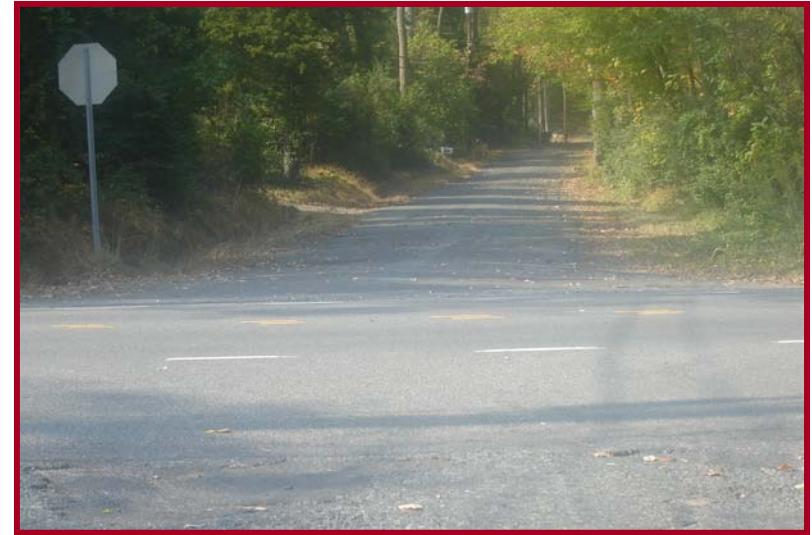
PA 663/Deep Creek Road intersection looking west
