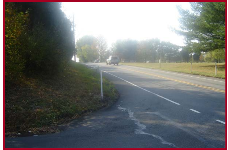
Little Road looking north on PA 663 south – limit sight distance due to curve
