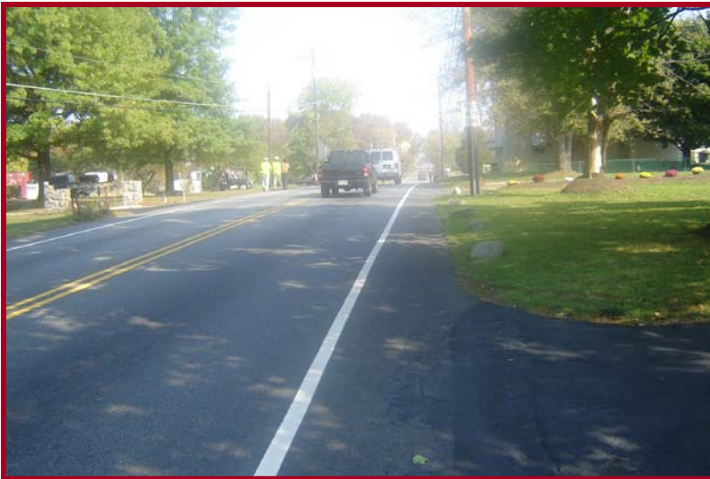
Rocks in the clear zone used for landscaping north of the Hoffmansville Road intersection
