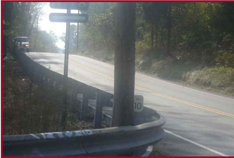
Guide rail at Deep Creek Road intersection
