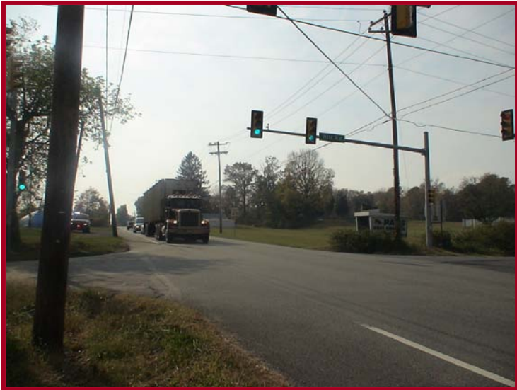
PA 663 at the Hill Road intersection
