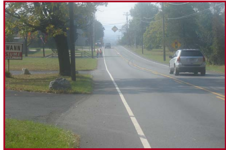
Southbound approach of the Hoffmansville Road intersection. Overhead advance warning sign hardly visible in the sunlight
