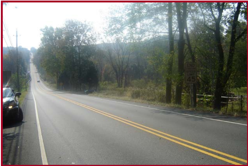
Southbound approach to box culvert over Deep Creek
