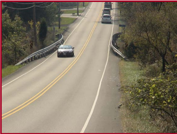
Box culvert over Deep Creek
