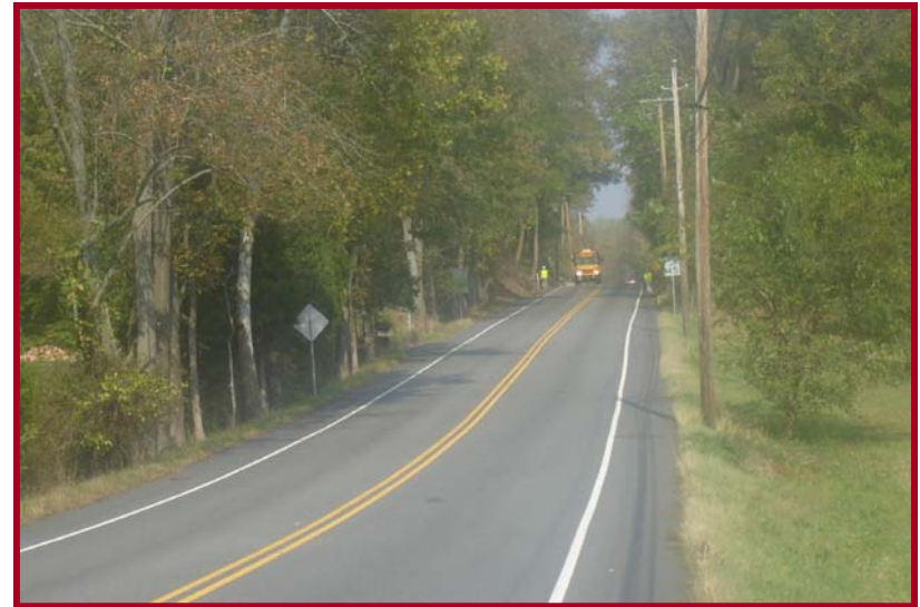
PA 663, north of box culvert over Deep Creek
