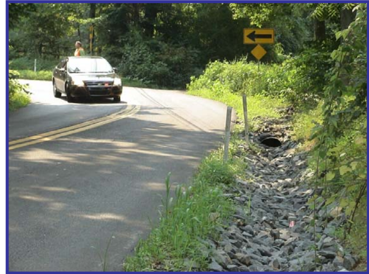
Treated drain on Aquetong Road on curve east of Sugan Road
