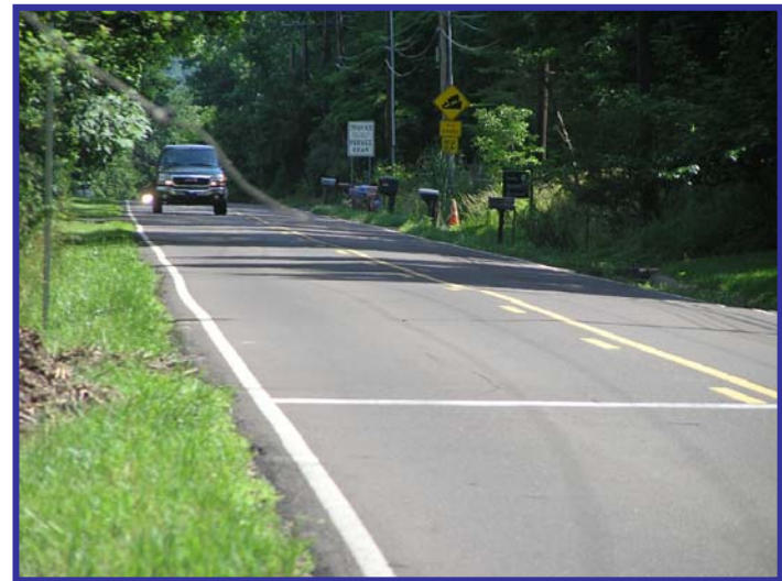
Windy Bush Road looking north at Cornwell Drive – passing zone, narrow shoulders
