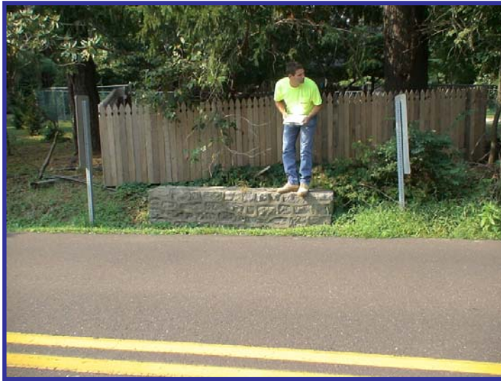
Stone headwall on Aquetong Road
