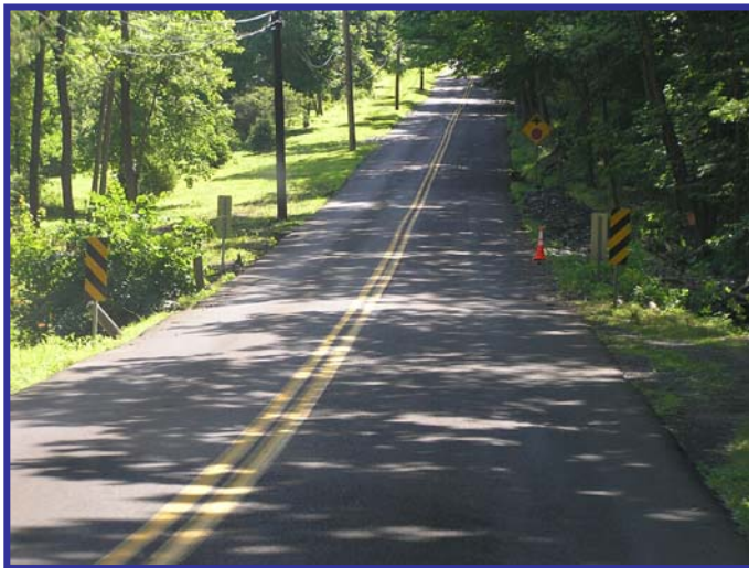
Narrow pavement of Aquetong Road, signs delineating inlet
