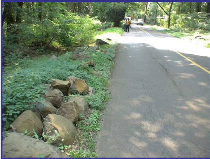
Rocks along Aquetong Road in the clear zone
