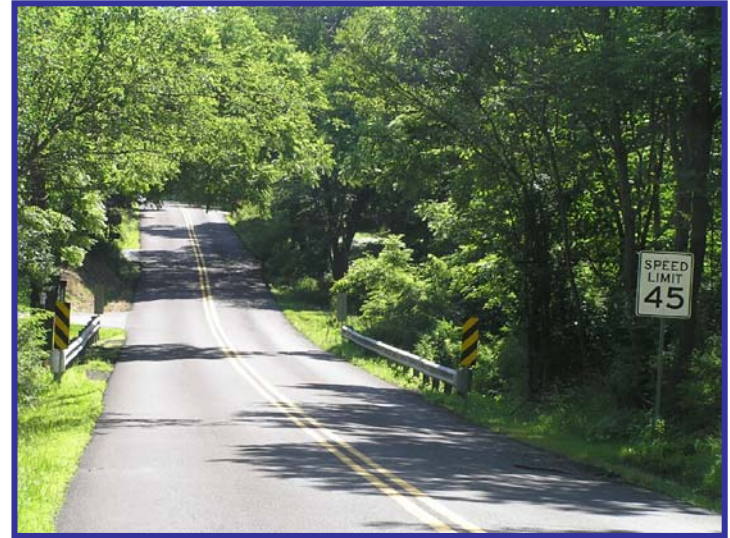
Narrow pavement of Aquetong Road west of Sugan Road, chevron signage at guide rail
