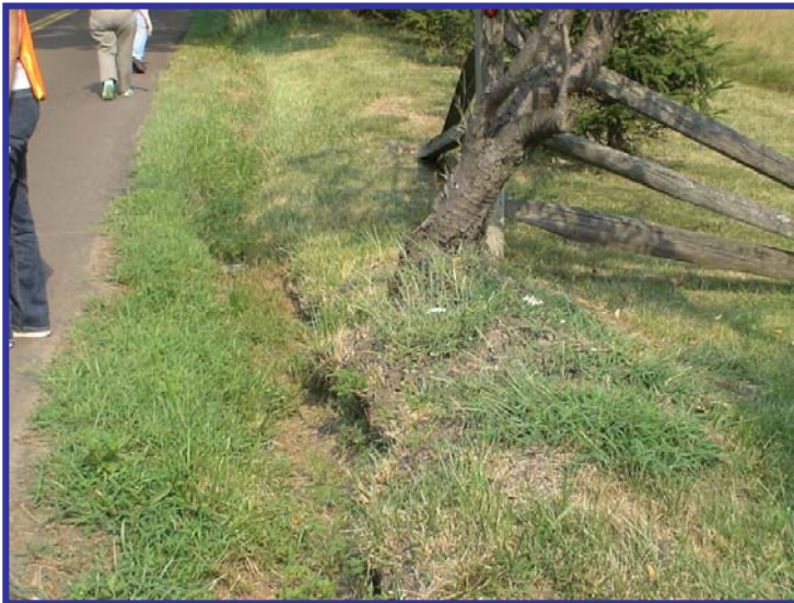
Poor drainage on Aquetong Road west of Cover Bridge Road
