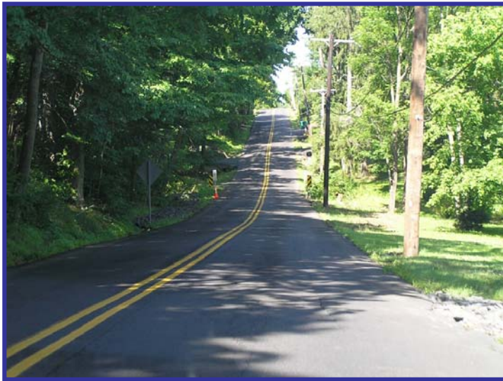
Utility poles in the clear zone on Aquetong Road east of Sugan Road
