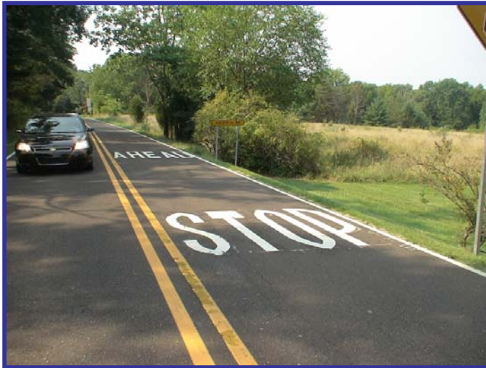
Pavement marking on Windy Bush Road north of the Aquetong Road intersection
