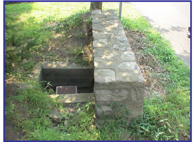
Stone headwall and inlet on Aquetong Road
