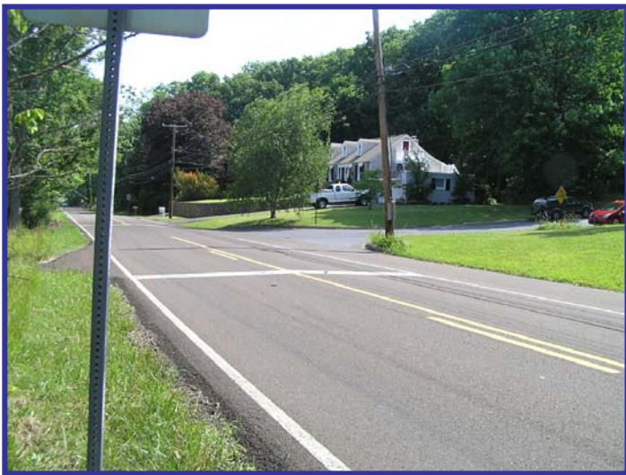
Windy Bush Road looking north at Cornwell Drive – passing zone, wider shoulders for decel lane
